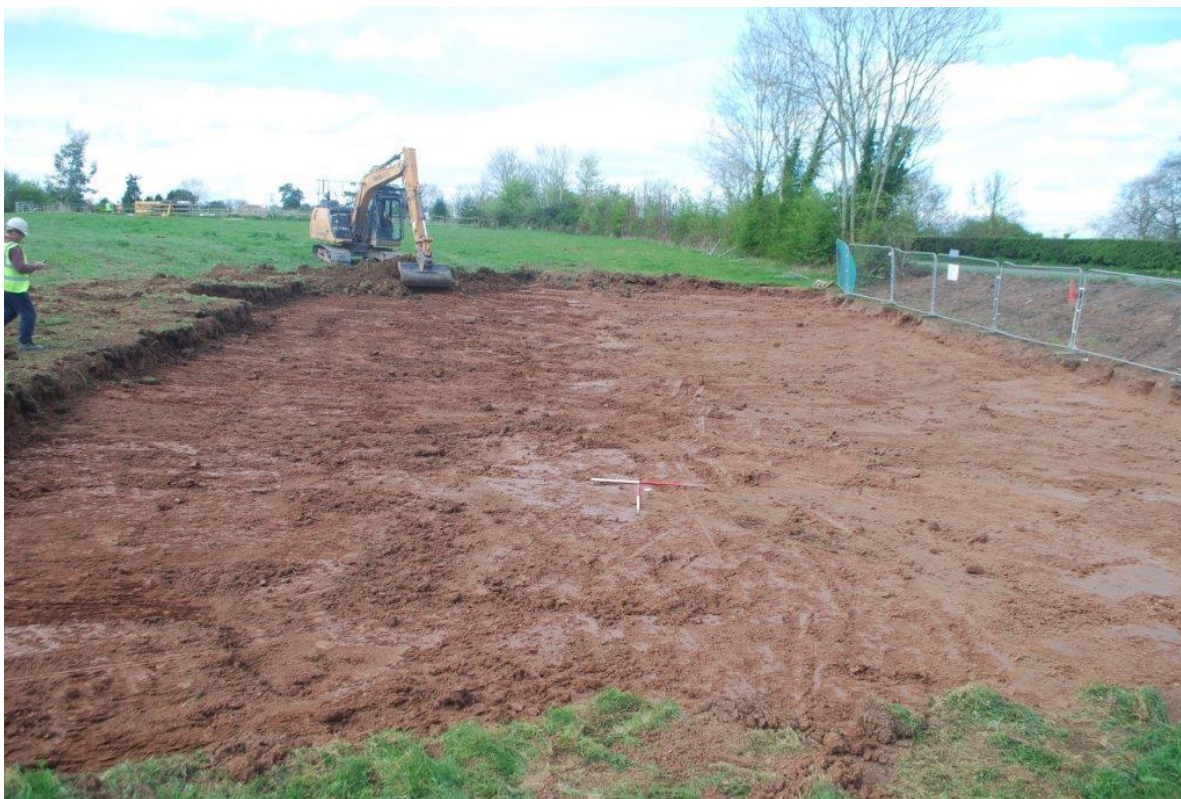
Plate 2 Topsoil stripping the southern access road. View North. 2 x1m scales.
