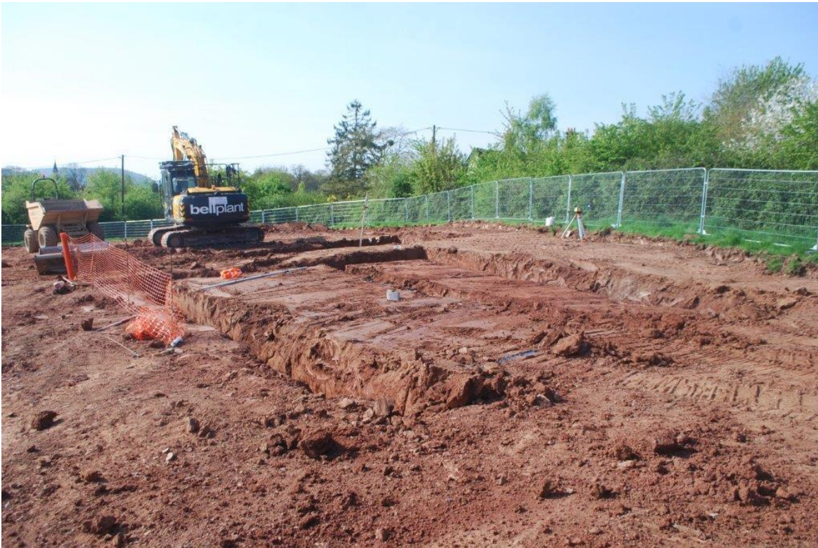
Plate 9 House footings in Northwest corner of south field
