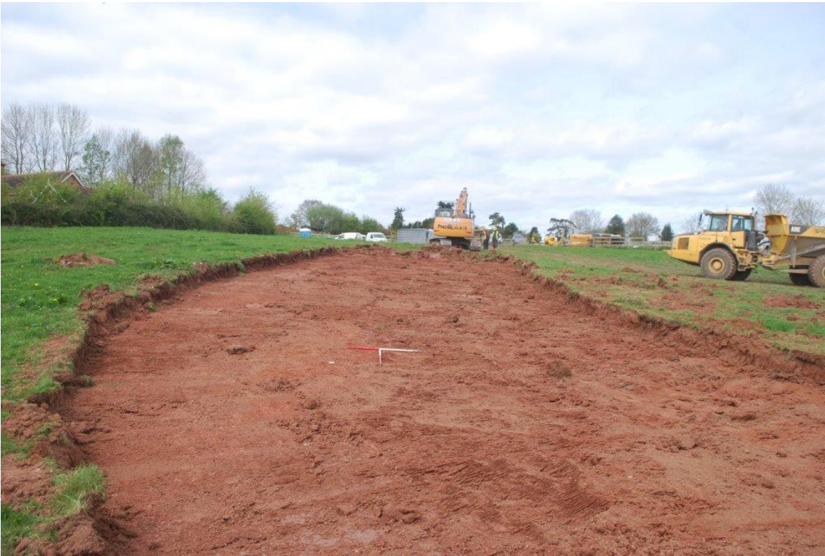
Plate 3 The road excavation onto natural clay. View North. 2x1m scales.
