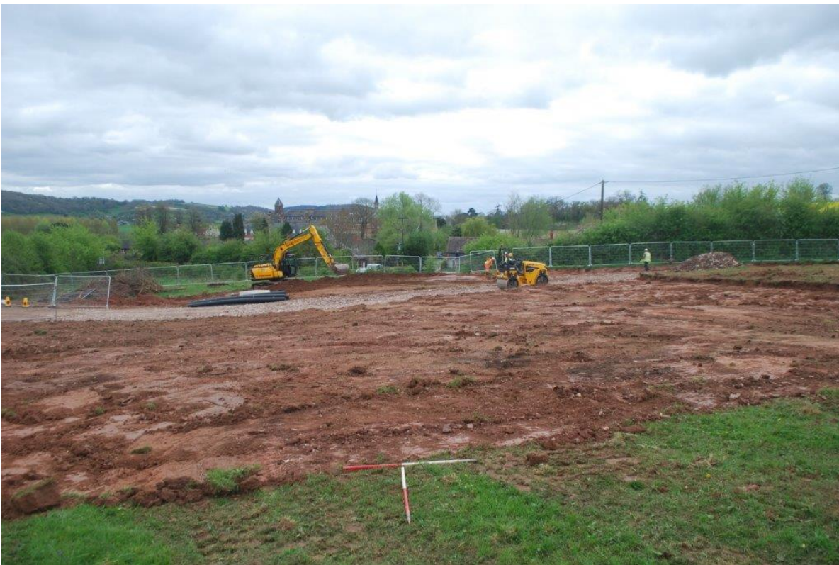
Plate 8 The hardcore track 104. View southwest with Convent in background.
