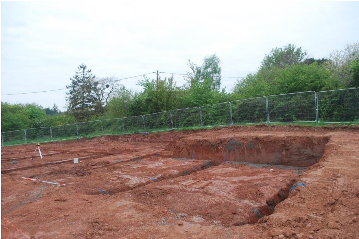
Plate 10 House footings and ground reduction in south field
