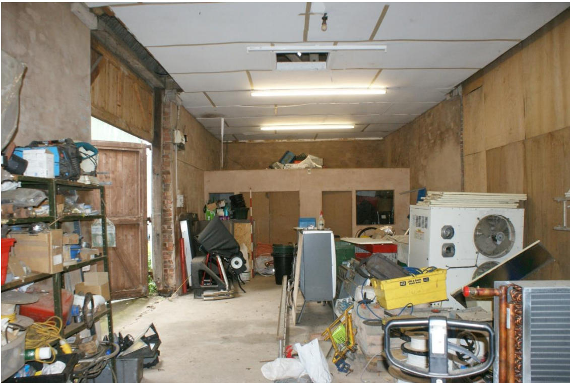
Plate 7 Phase 1 barn, looking east
