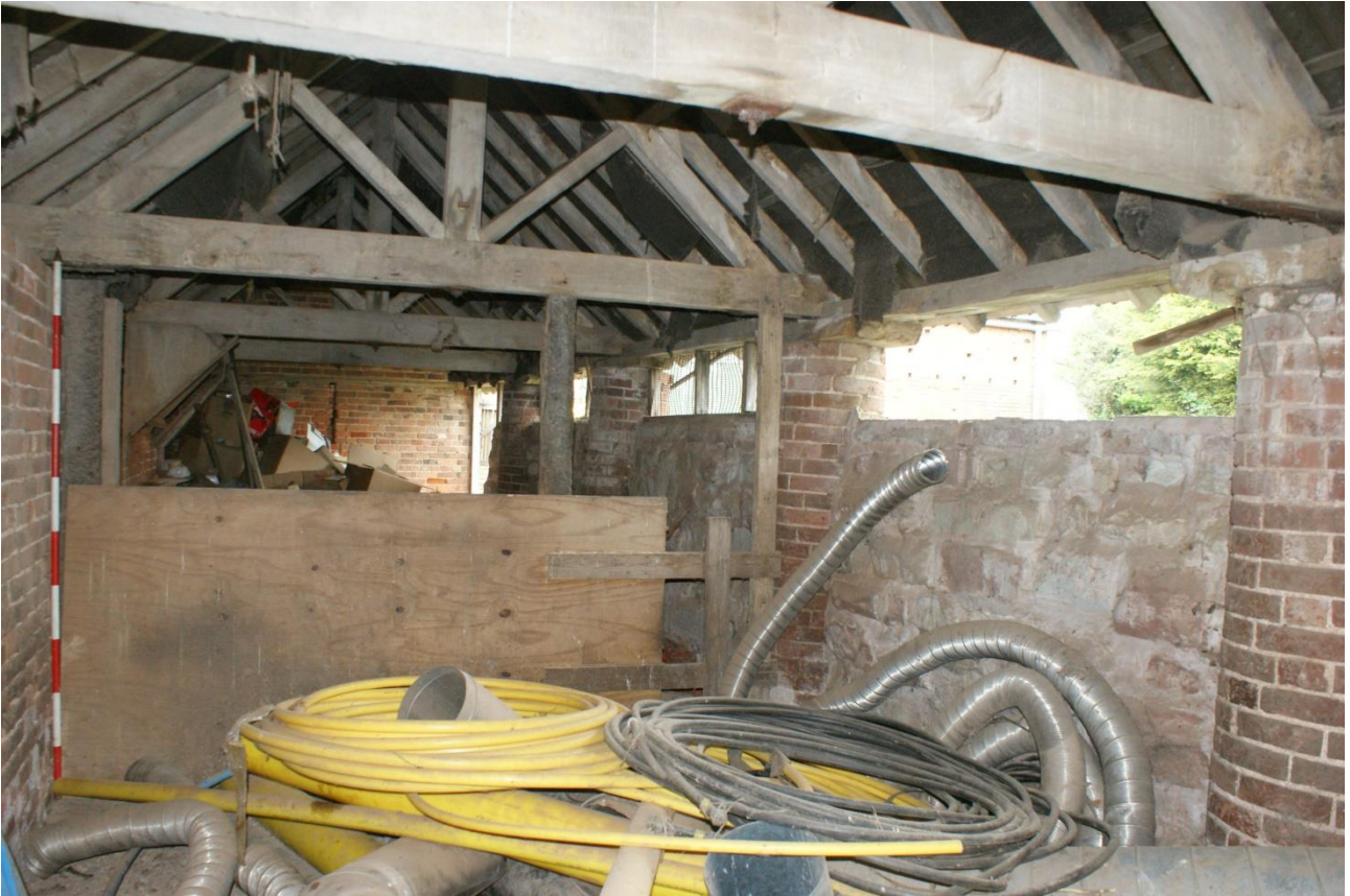
Plate 15 Phase 2 cow shed, looking north
