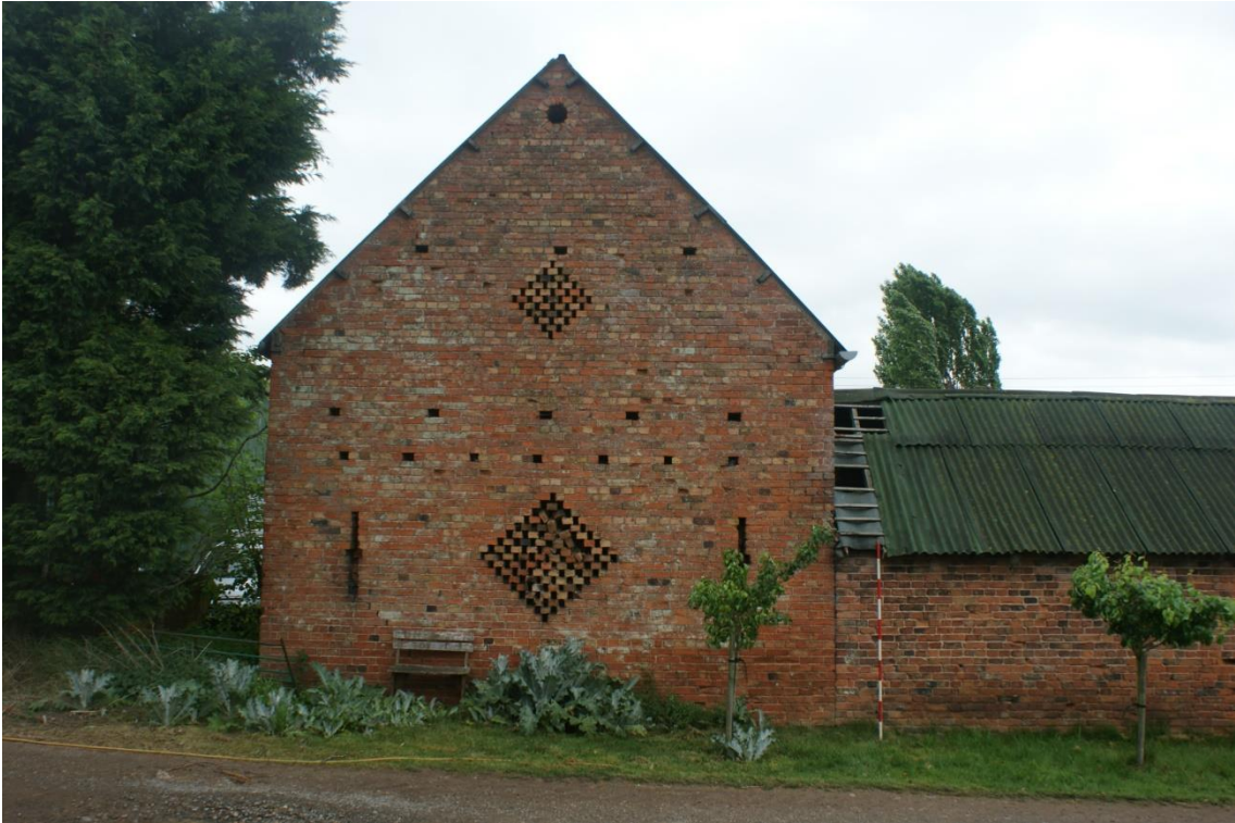
Plate 4 Phase 1 barn, looking east
