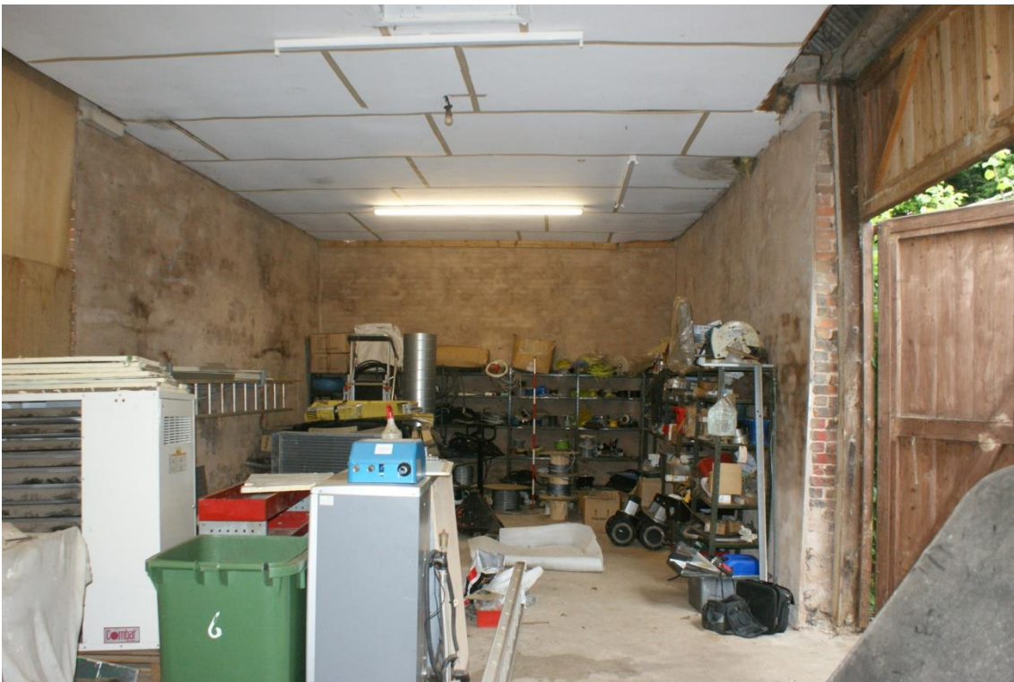
Plate 8 Phase 1 barn, looking west
