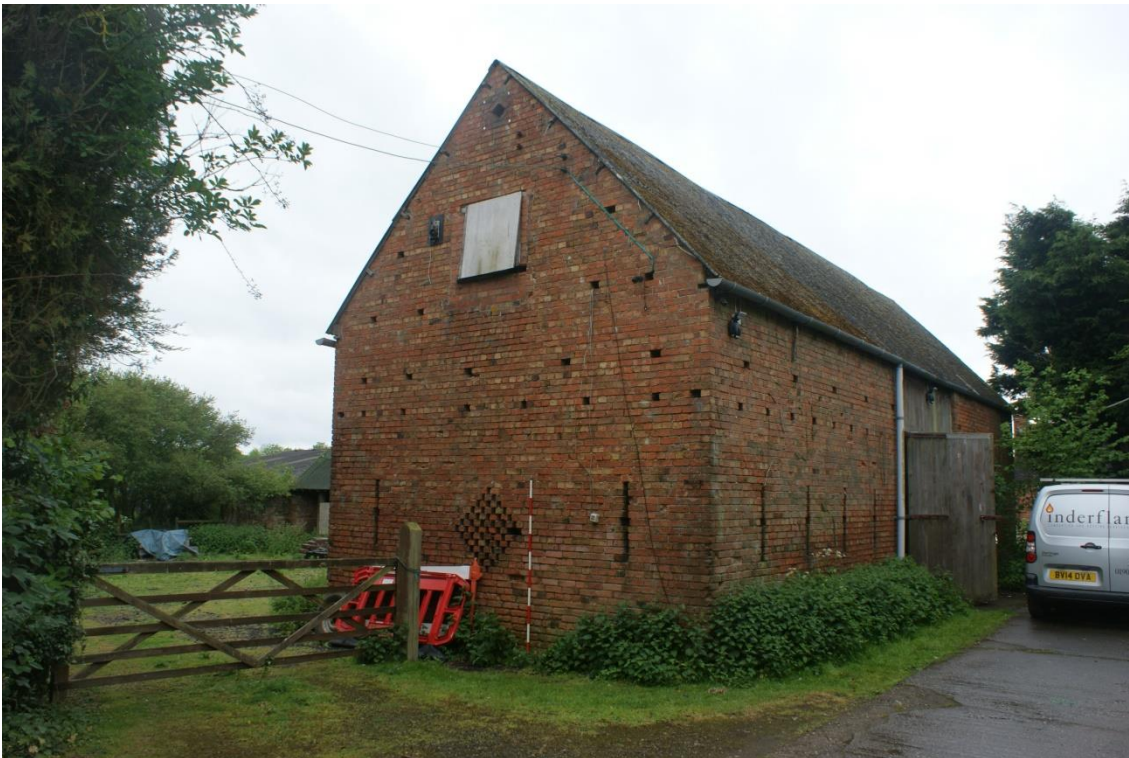
Plate 1 Phase 1 barn, looking south-west
