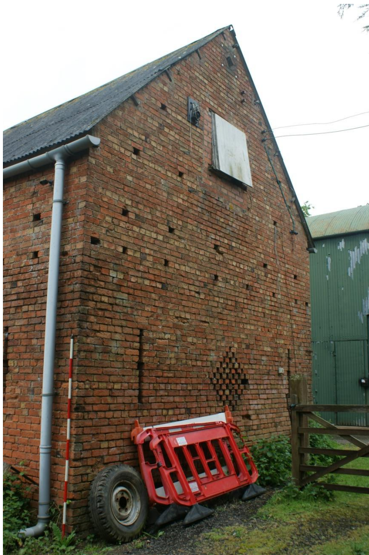
Plate 2 Phase 1 barn, looking south-west
