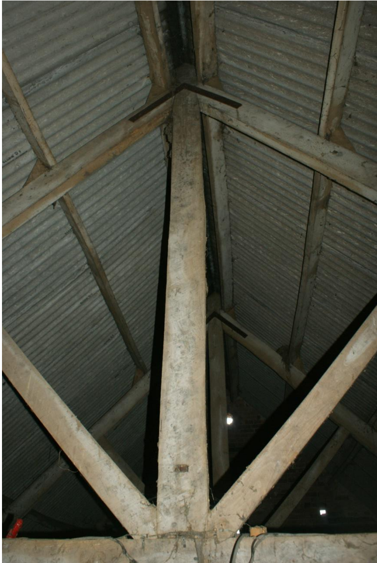
Plate 10 Phase 1 barn, looking east
