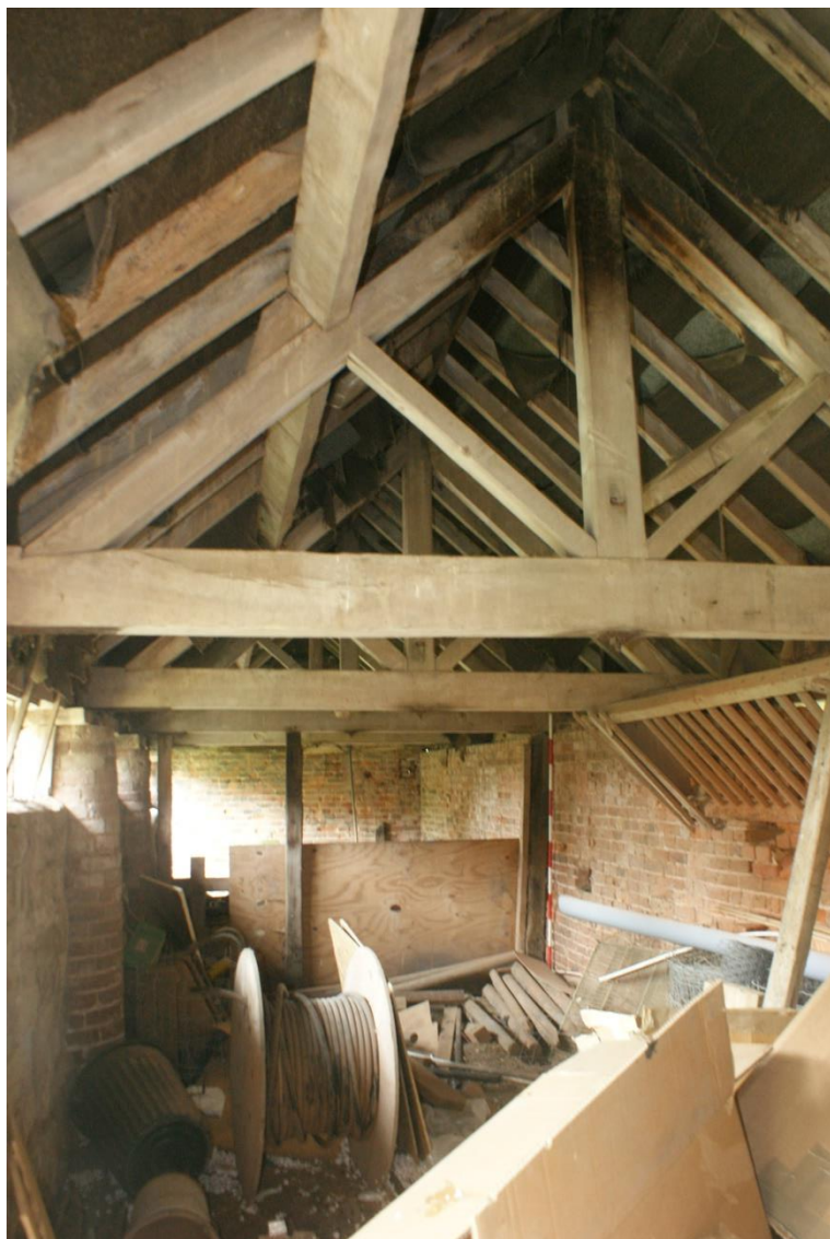
Plate 14 Phase 2 cow shed, looking south
