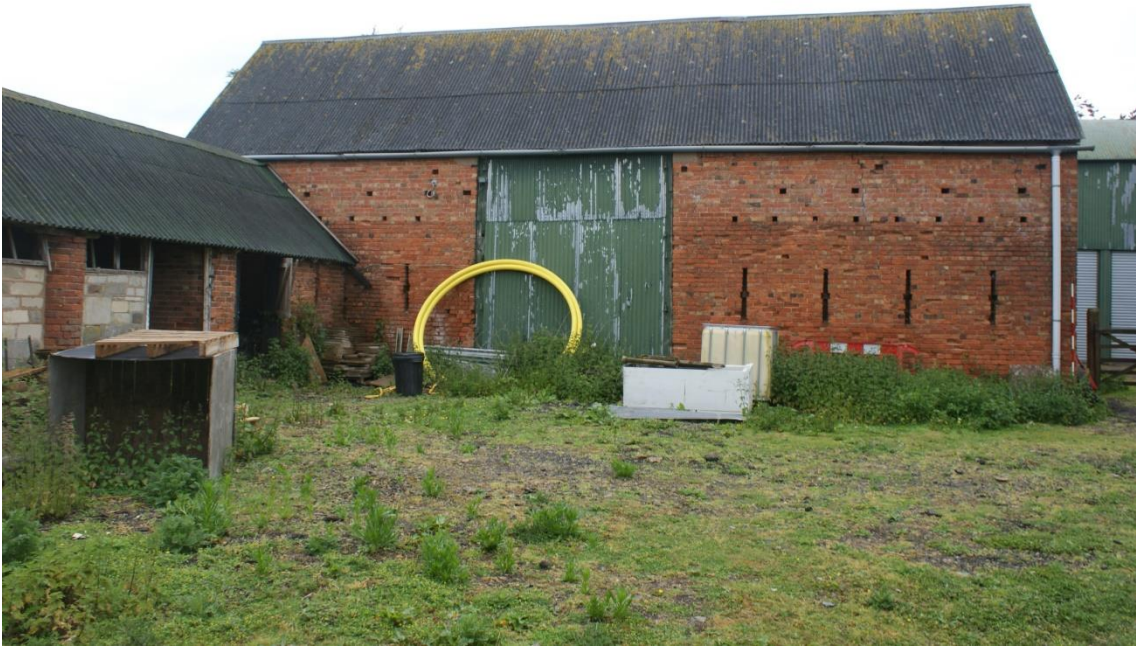
Plate 3 Phase 1 barn, looking north
