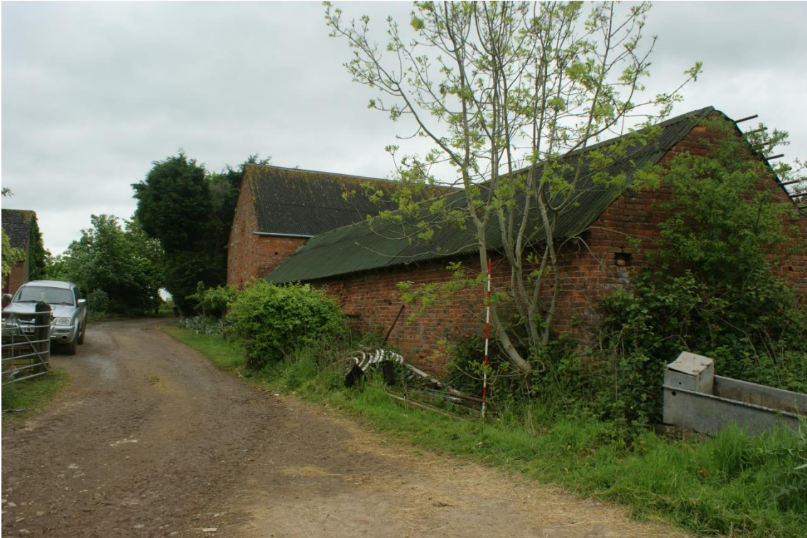
Plate 12 Phase 2 cow shed, looking north-east
