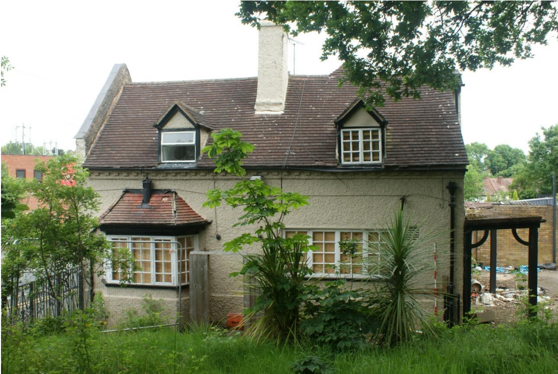
Plate 17 Phase 3 bay window, looking north, scale 2m
