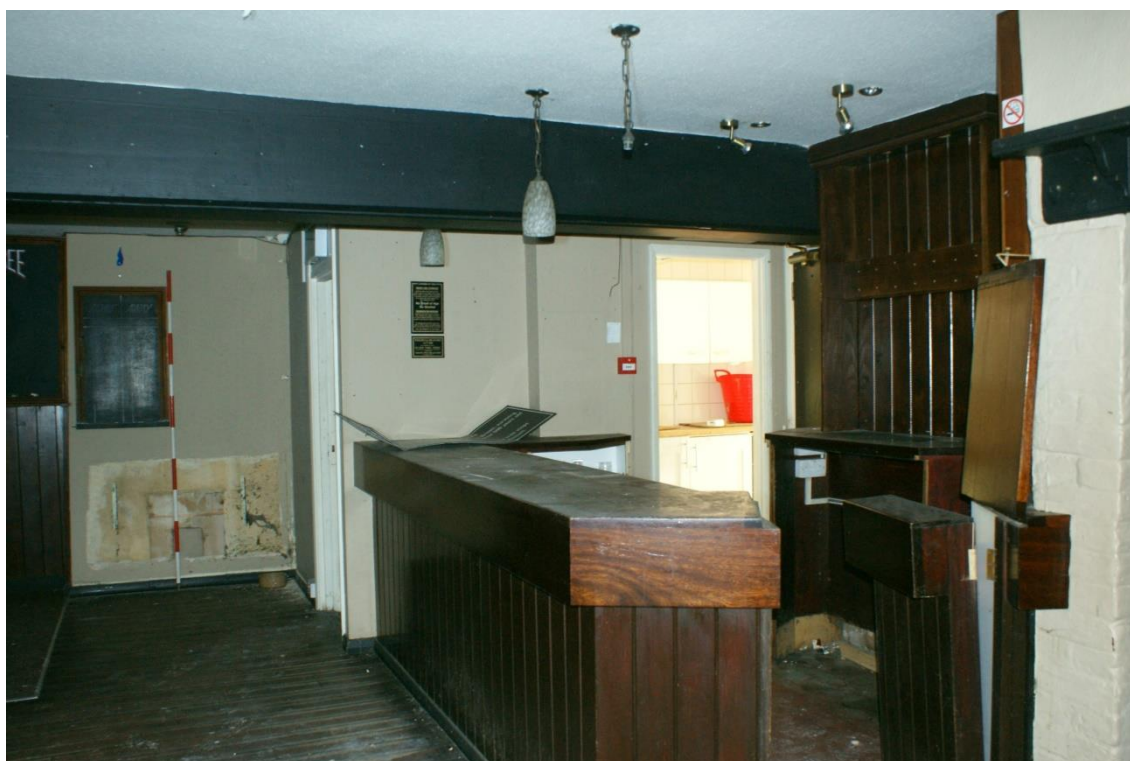
Plate 15 Interior of Phase 2 building, looking north, scale 2m
