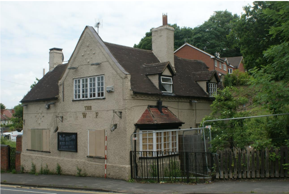
Plate 2 The building, looking north-east, scale 2m
