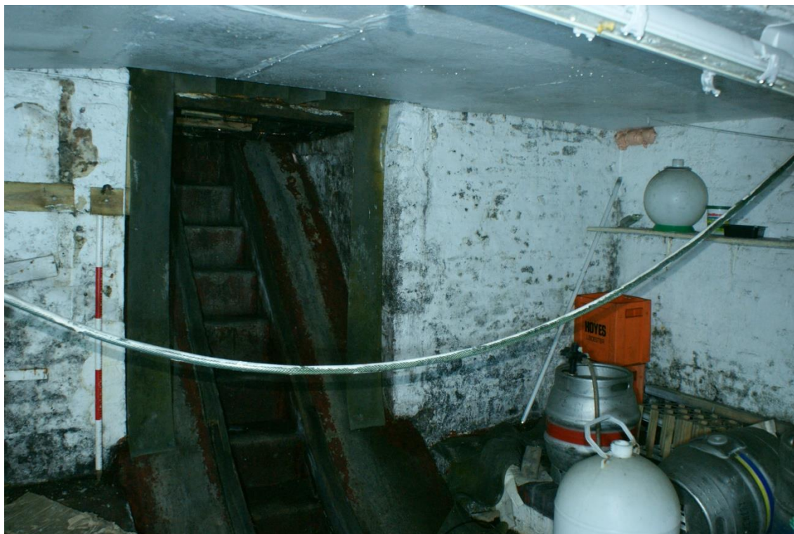
Plate 8 Cellar of Phase 1 building, looking south-west, scale 1m
