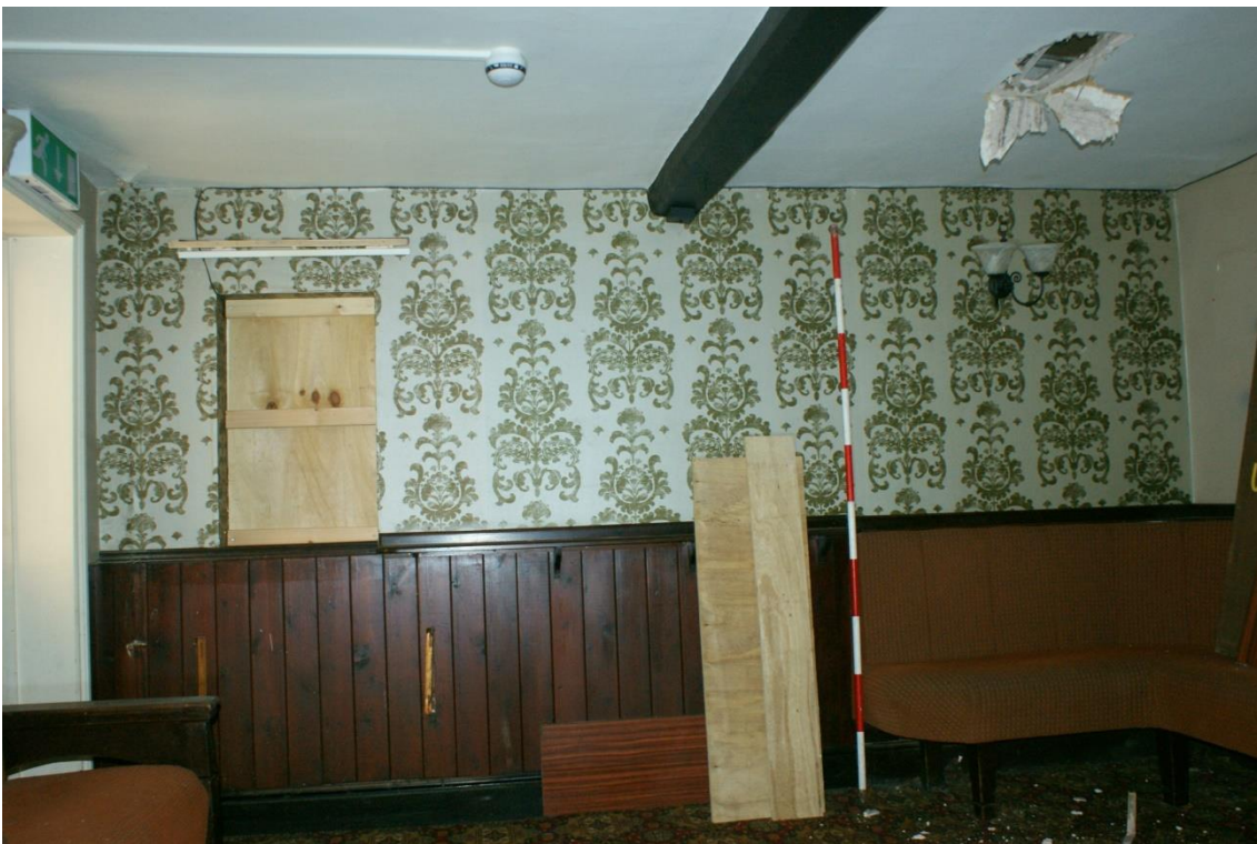
Plate 6 Phase1 building, looking east, scale 2m
