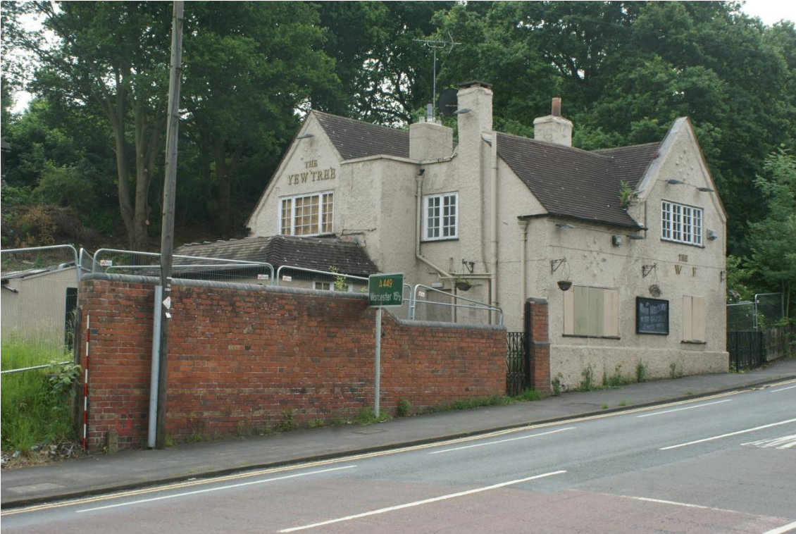
Plate 1 The building, looking south-east, scale 2m
