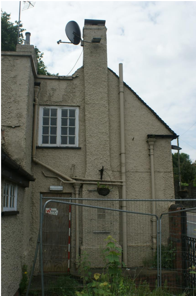
Plate 14 Phase 2 building, looking south, scale 2m
