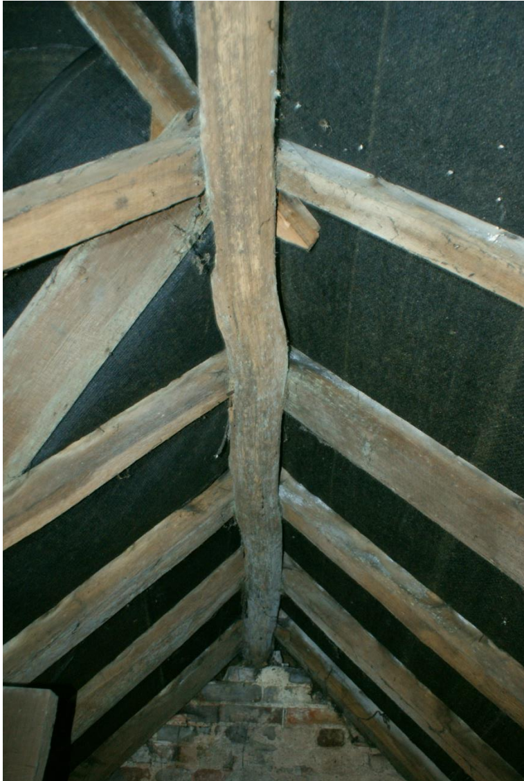
Plate 13 Roof of Phase1 building, looking west
