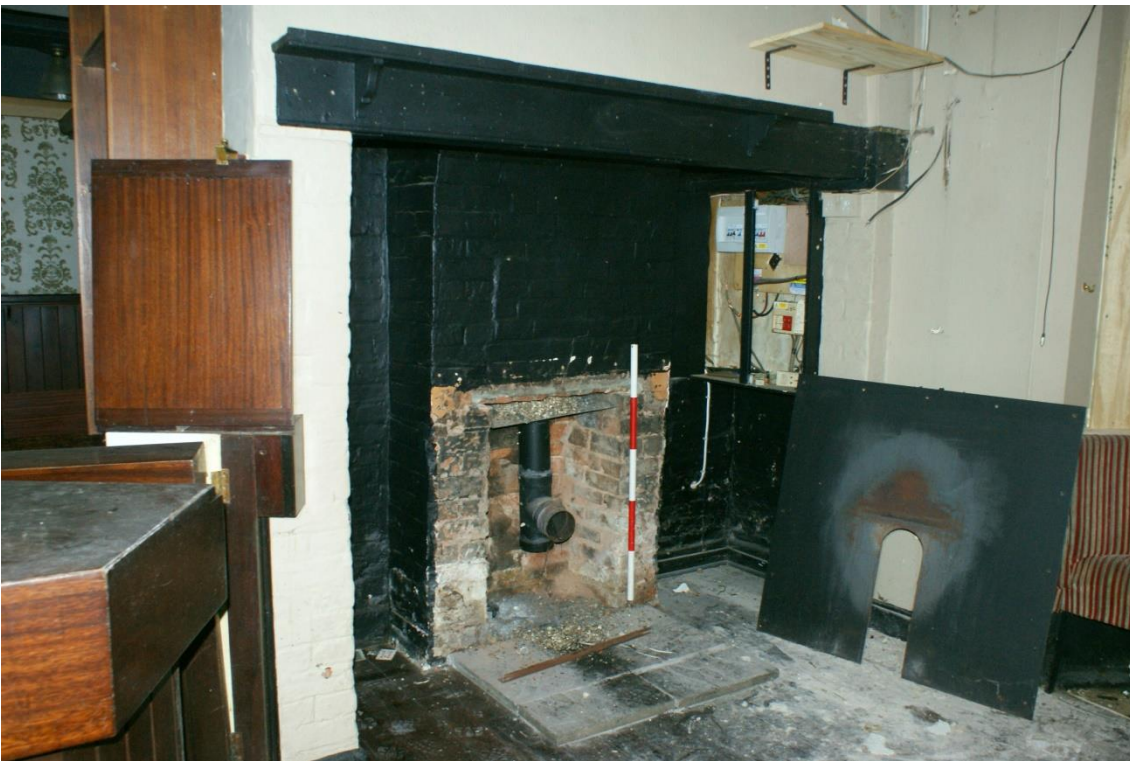
Plate 4 Interior of phase 1 building, looking south-west, scale 1m
