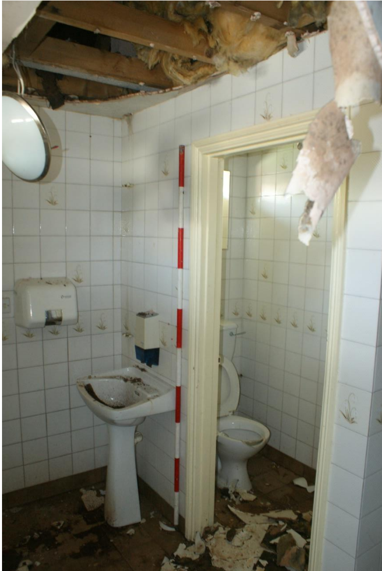
Plate 28 Interior of Phase 5 building, looking north-east, scale 2m
