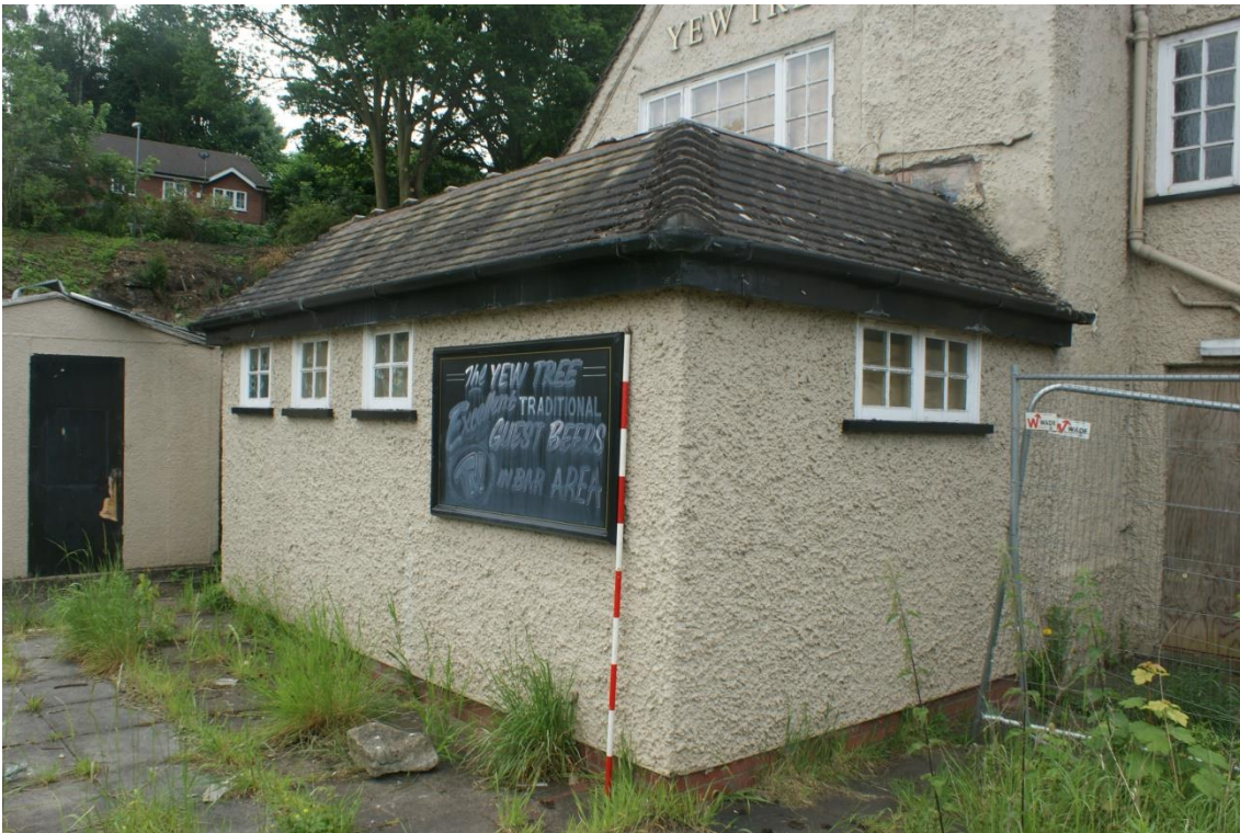
Plate 27 Phase 5 building, looking south-east, scale 2m
