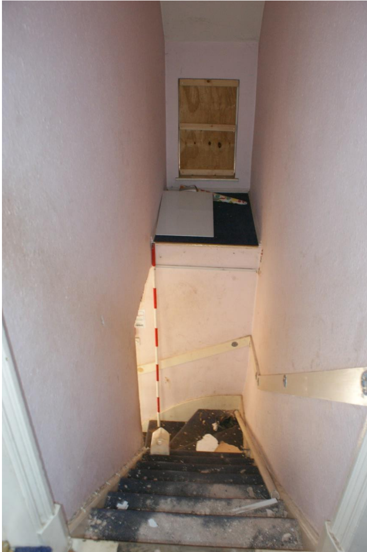
Plate 22 Staircase within Phase 4 building, looking east, scale 2m
