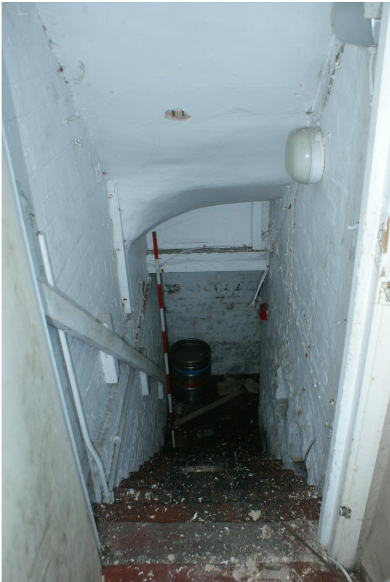
Plate 23 Phase 4 building steps to cellar, looking east, scale 2m
