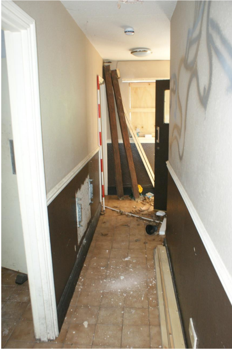
Plate 20 Interior corridor of Phase 4 building, looking east, scale 2m
