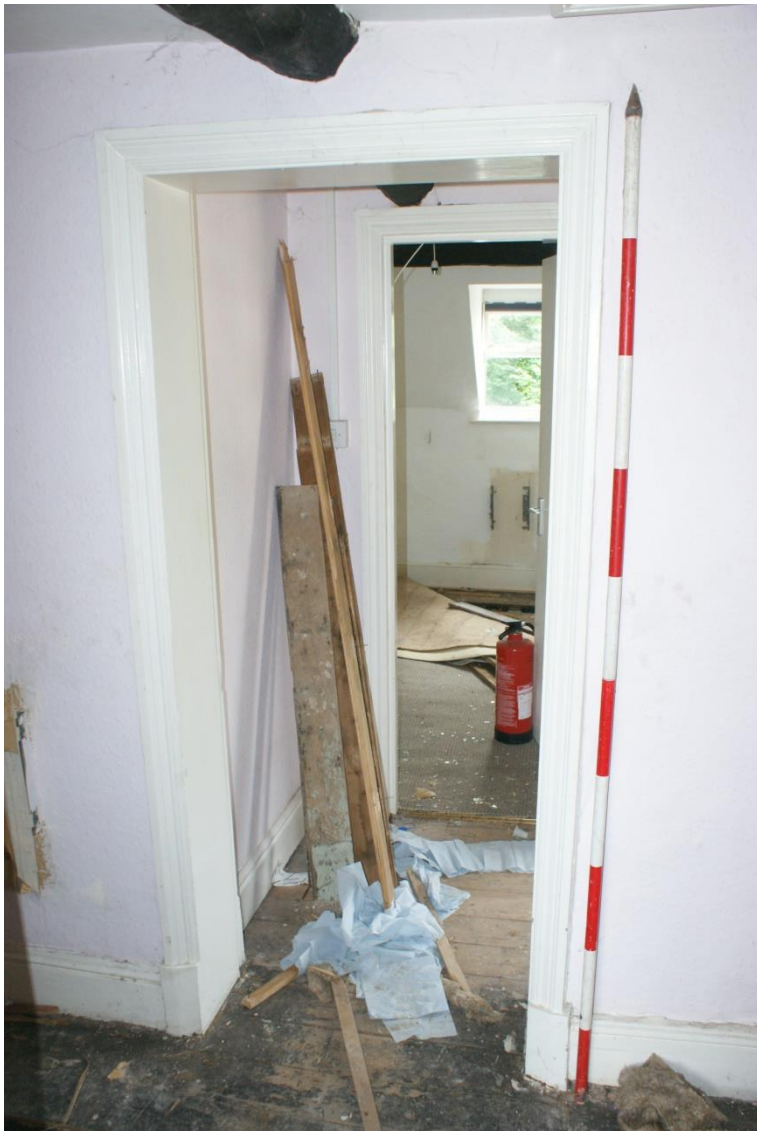
Plate 25 Door surrounds and skirting within Phase 4 building, looking south, scale 2m
