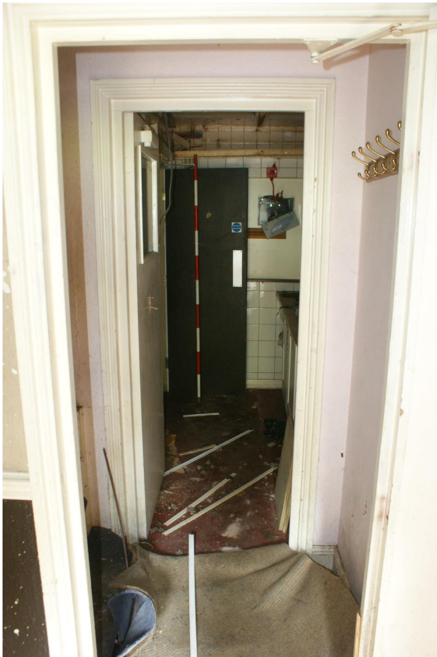
Plate 19 Interior of Phase 4 building, looking west, scale 2m
