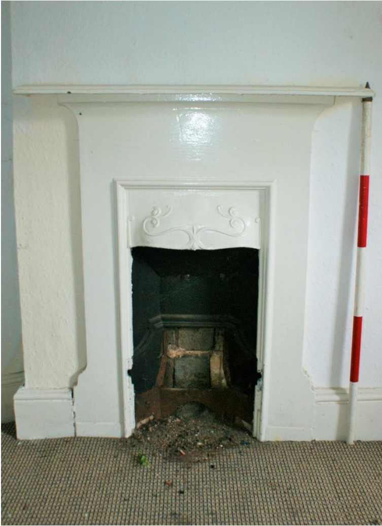
Plate 26 Decorative chimney breast, Phase 4 building, looking east, scale 2m
