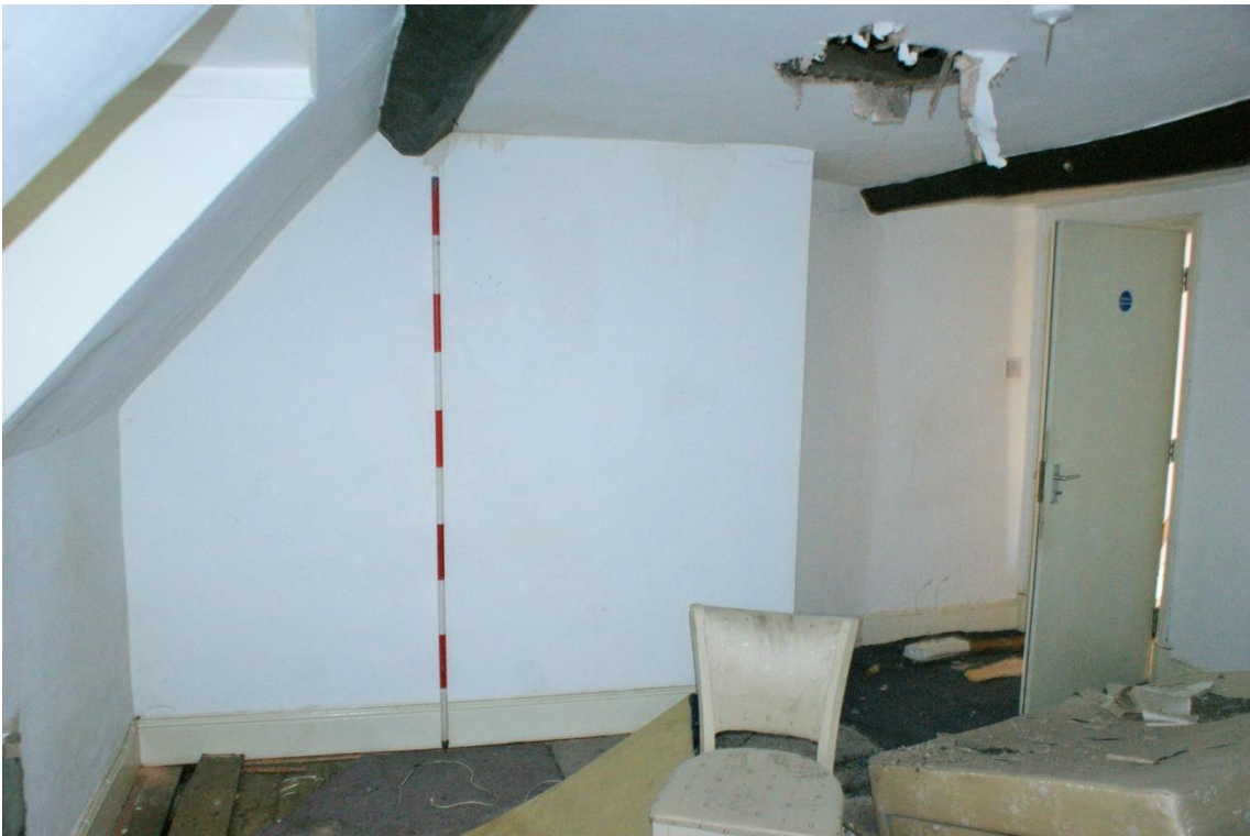
Plate 10 First floor Phase1 building, looking west, scale 2m
