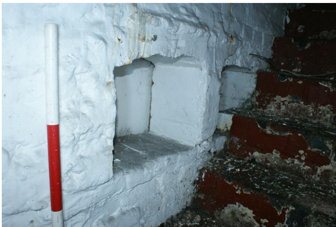
Plate 9 Cellar of Phase 1 building, looking south-west, scale 0.4m
