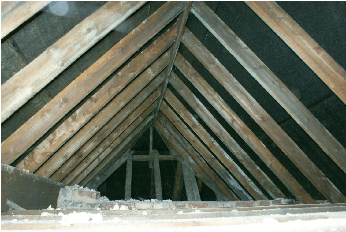
Plate 24 Roof of Phase 4 building, looking south
