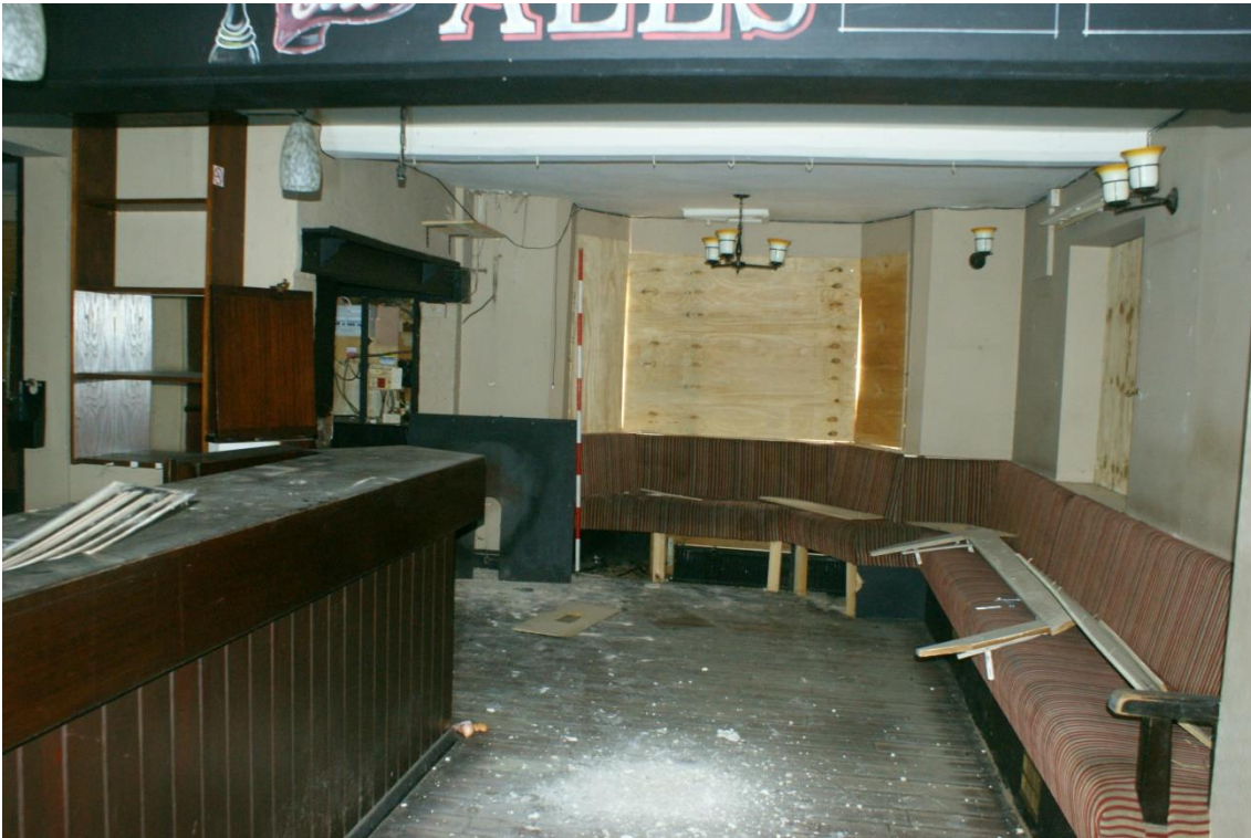
Plate 5 Phase1 building, looking south, scale 2m
