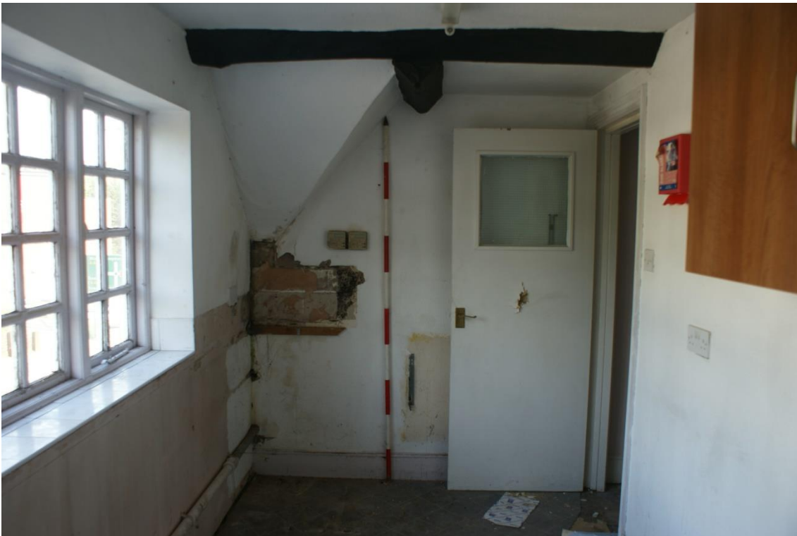
Plate 12 First floor Phase1 building, looking north, scale 2m
