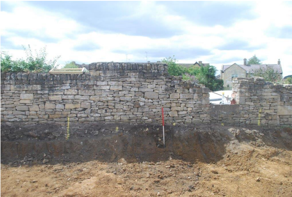
Plate 5 Limestone wall bounding south-west side of site and section showing ground reduction depth, 1m scale
