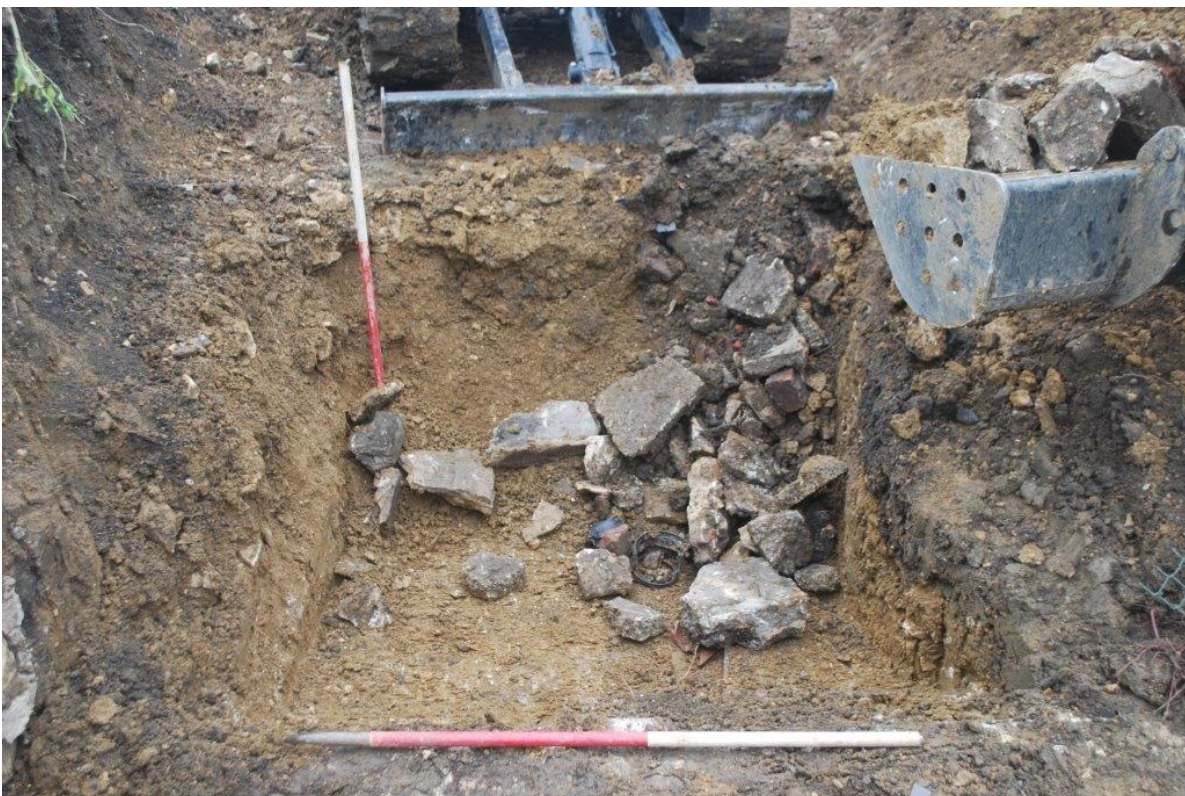
Plate 6 Soakaway pit with modern truncation from an existing soakaway, 2x 1m scales
