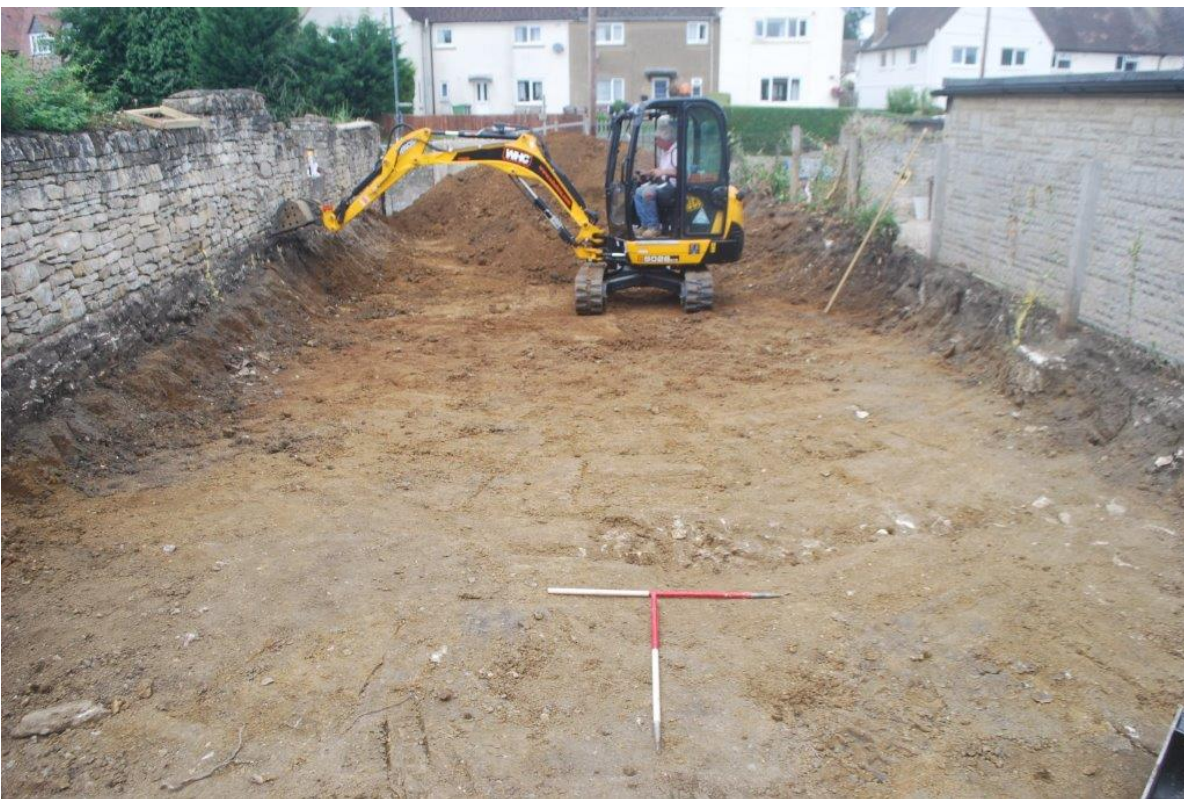
Plate 2 South-east end of site ground reduction, 2x 1m scales
