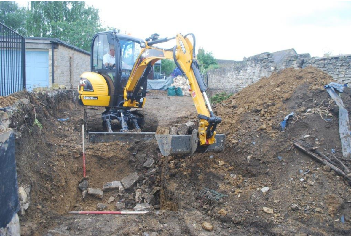
Plate 7 Location of soakaway pit, view south-east, 2x 1m scales
