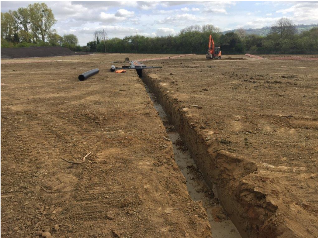
Plate 2: typical drainage pipe cut in eastern field
