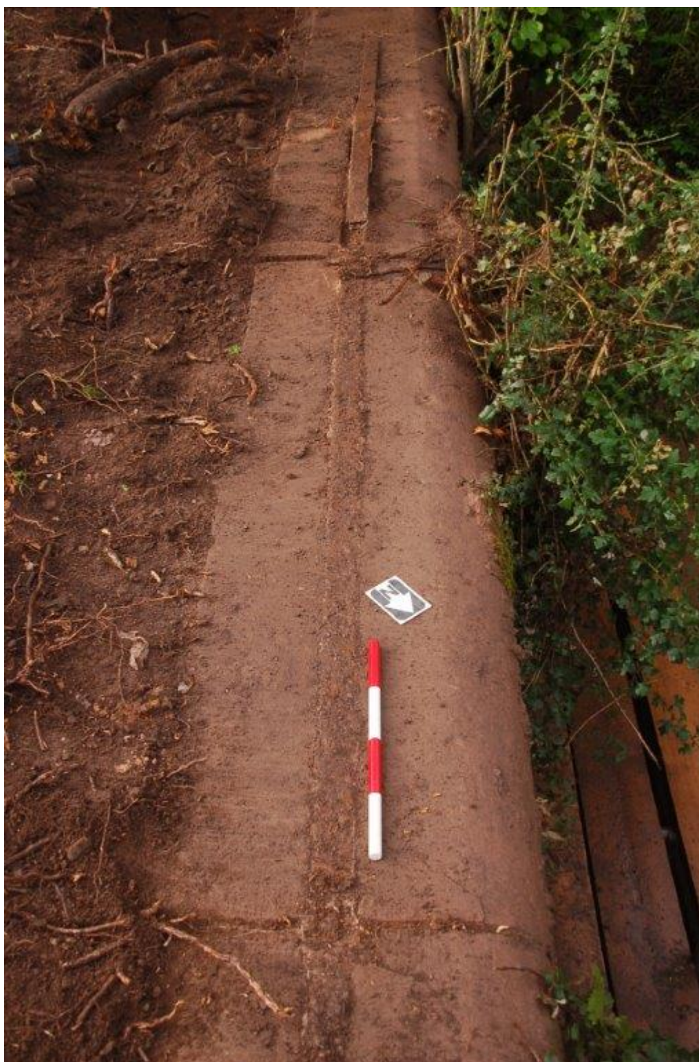
Plate 7. Upper iron strapping which ran the length of the coping stones, led into chiselled-out cavities, view south-west, scale 0.4m
