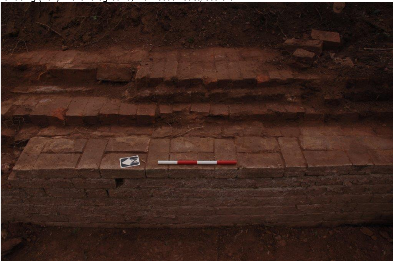
Plate 9. The original flanking wall (104), in the background, abutted by the later engineering brick re-facing (107), in the foreground, view south-east, scale 0.4m
