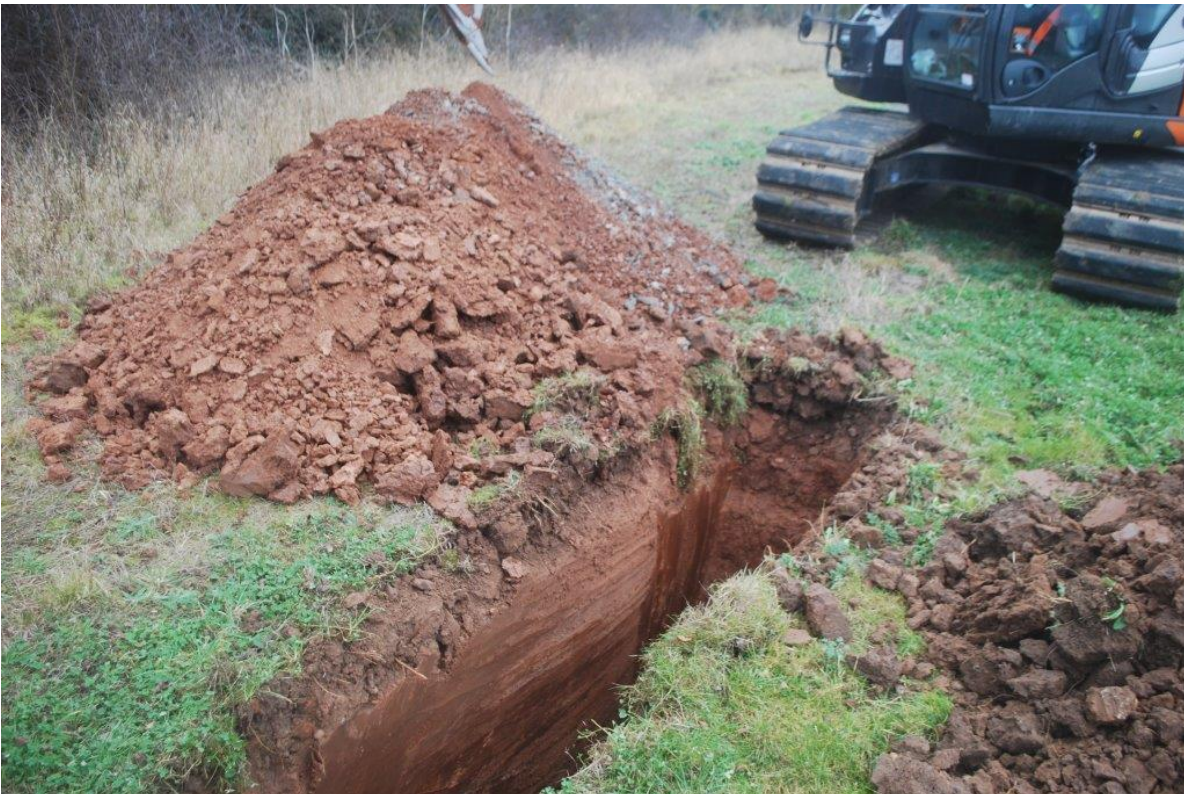
Plate 4 Example of excavation of Trial Pit 23 into deeper Mercian Mudstone geology.
