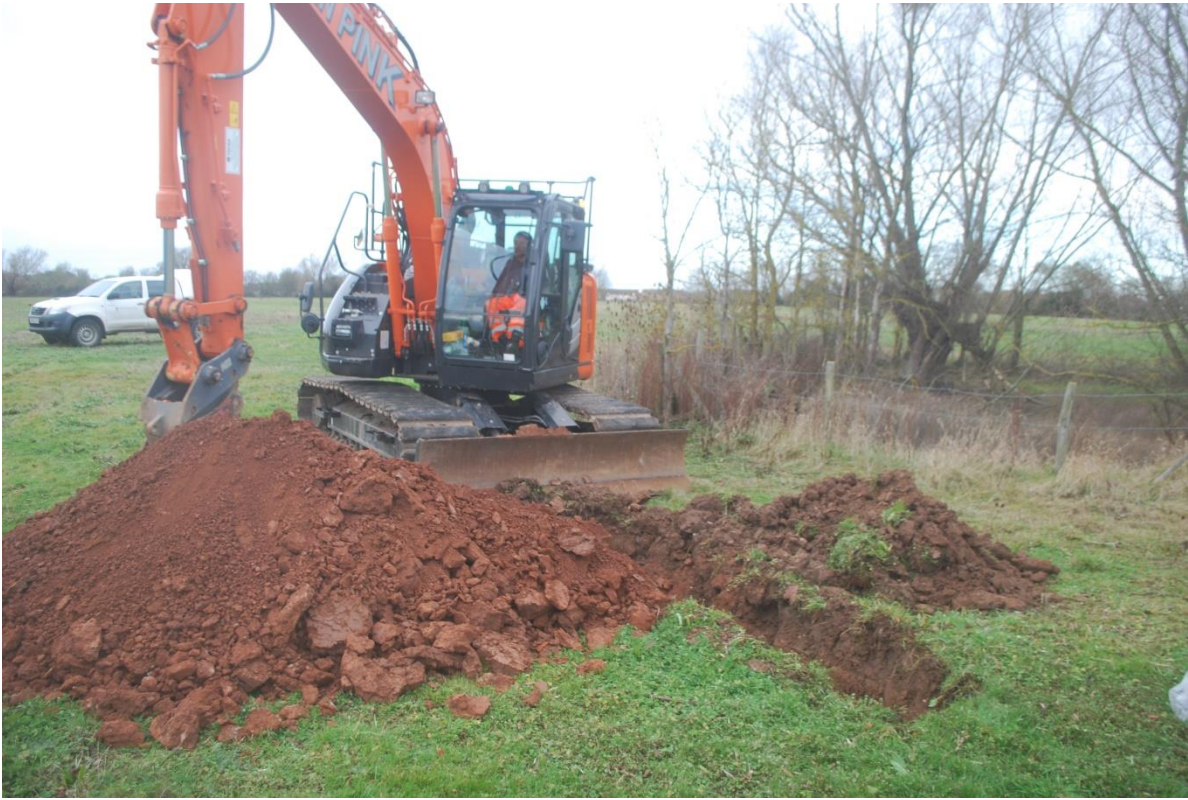
Plate 8 Deeper excavation of TP44 south of former pond.
