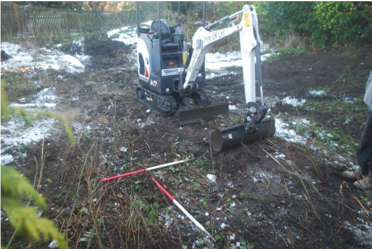
Plate 1 The site prior to excavation; view south-east; 2x 1m scales
