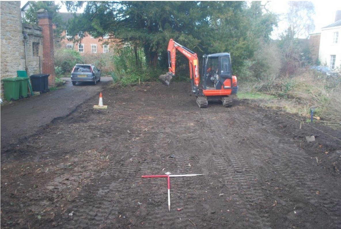
Plate 15 The site after excavation, looking north-west, 2x 1m scales
