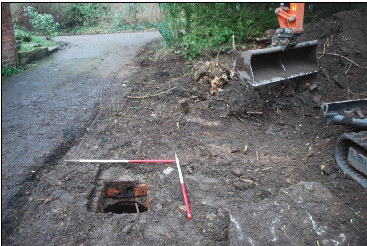
Plate 10 Manhole over capped well (107), view north-west, 2x 1m scales
