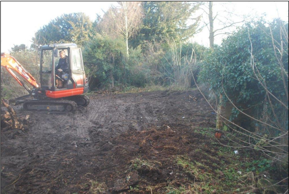
Plate 3 The site following clearance of vegetation, view north-east towards hedgerow
