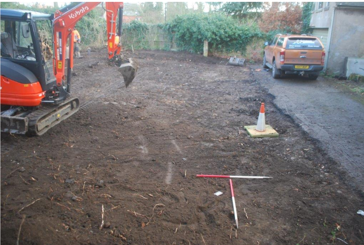
Plate 16 The site after excavation, looking south-east, 2x 1m scales
