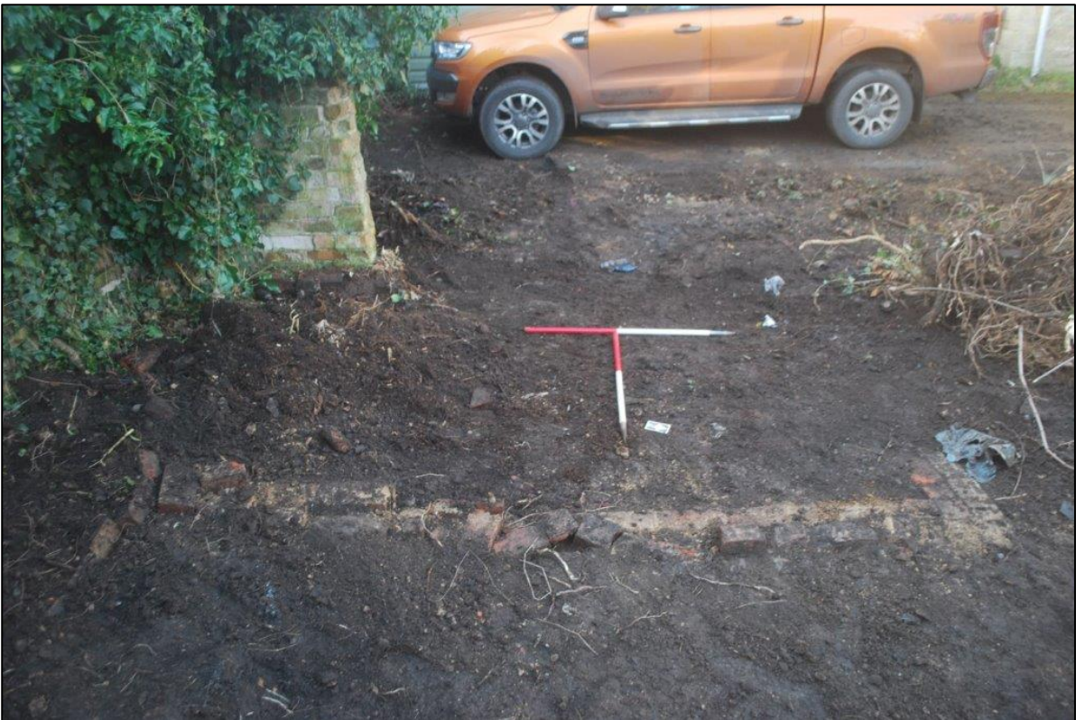
Plate 8 Brick foundations (103), possible cart-shed, view south-west, 2x 1m scales
