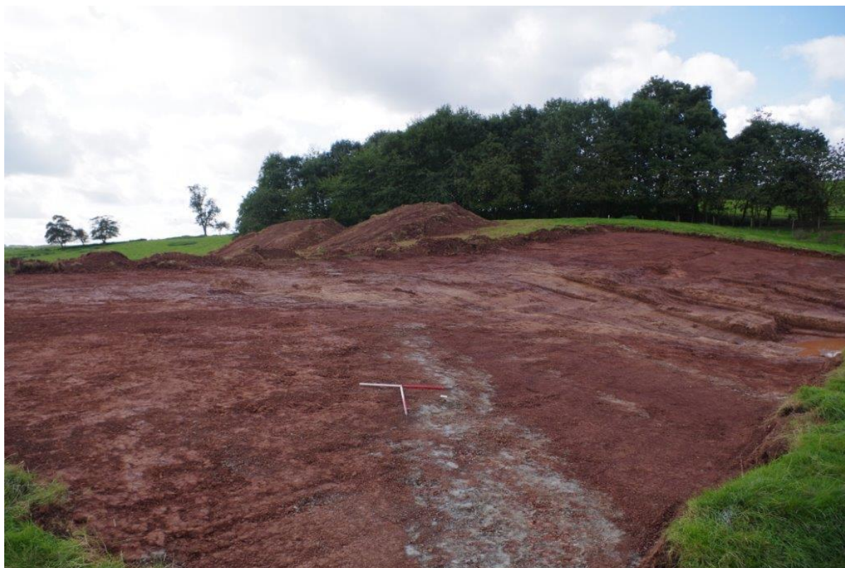
Plate 1 Area 1 looking south-west (1m scales)
