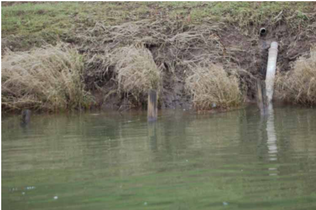
Figure 7 Posts possibly representing the last landing stage of Clevelode ferry (UID 92; west bank)
