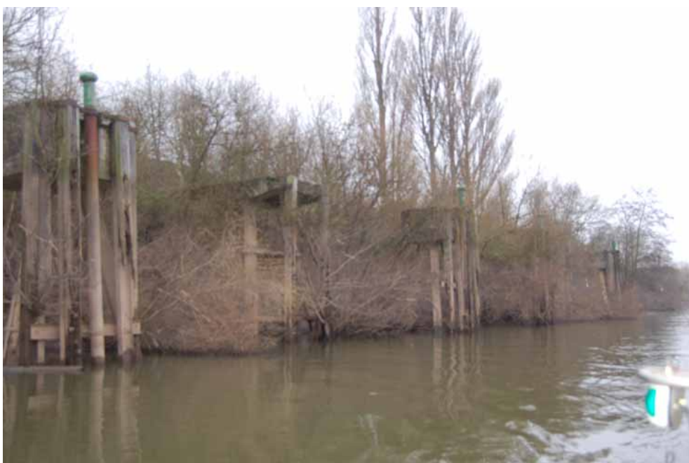
Figure 9 Disused oil storage facility south of Upton-on-Severn (UID 280; east bank). Six wooden towers holding vertical pipes were associated with a World War II fuel depot which was supplied by barges from Avonmouth in Gloucestershire (Wilks 2007, 134-5). A jetty stood beneath the towers but was demolished in the 1970s or 1980s. The fuel tanks were in the compound 350m to the east, although others probably lie beneath the long mound immediately behind the river-bank. A similar complex is also located just south of Worcester (UID 278).
