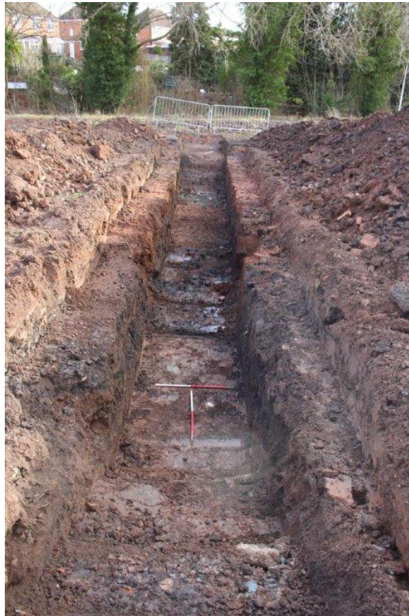
Plate 2: General view of Trench 1, facing south east, with modern deposits visible
