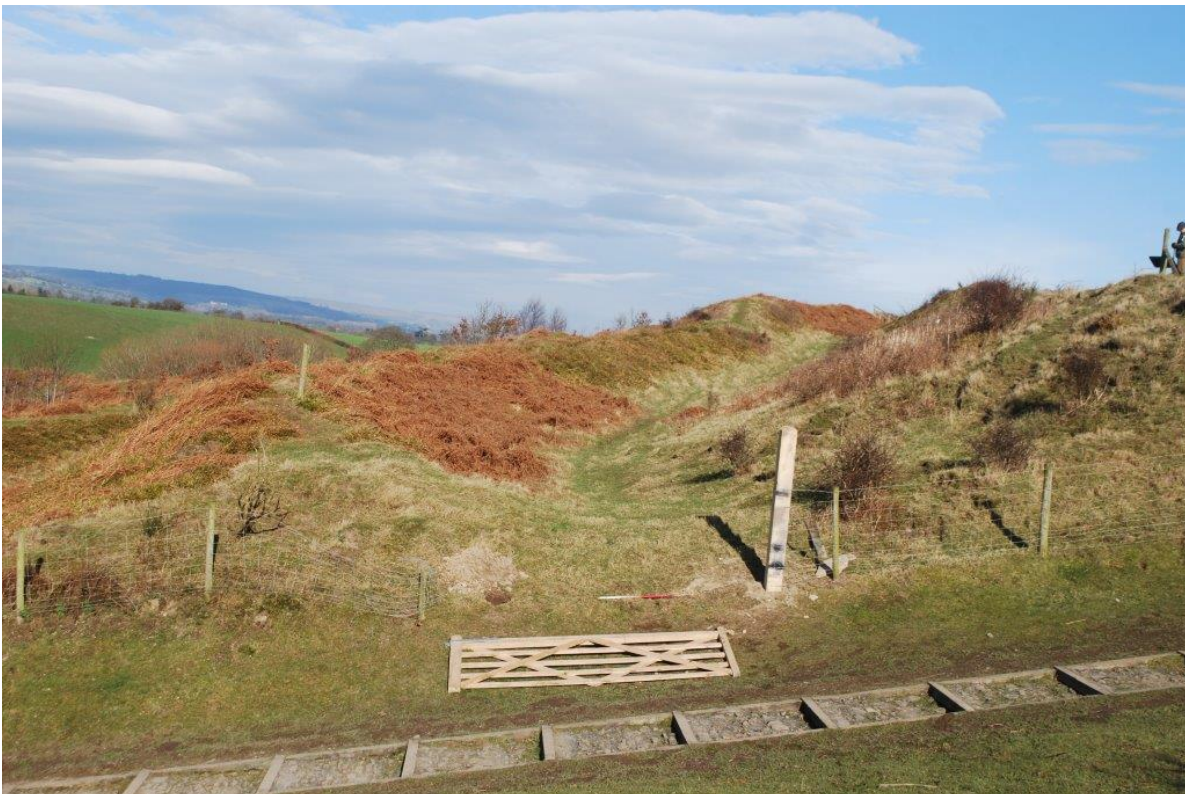
Plate 6: Gate post installed and posthole excavated on west side of hillfort; facing north
