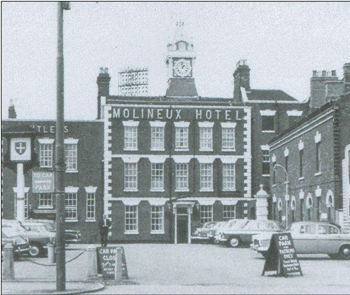
Plate 11: View north of the front façade, c 1960 (WCC 2005)
