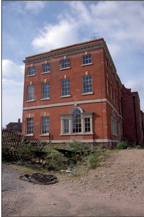
Plate 14: Garden Range east elevation and retaining wall, view south
