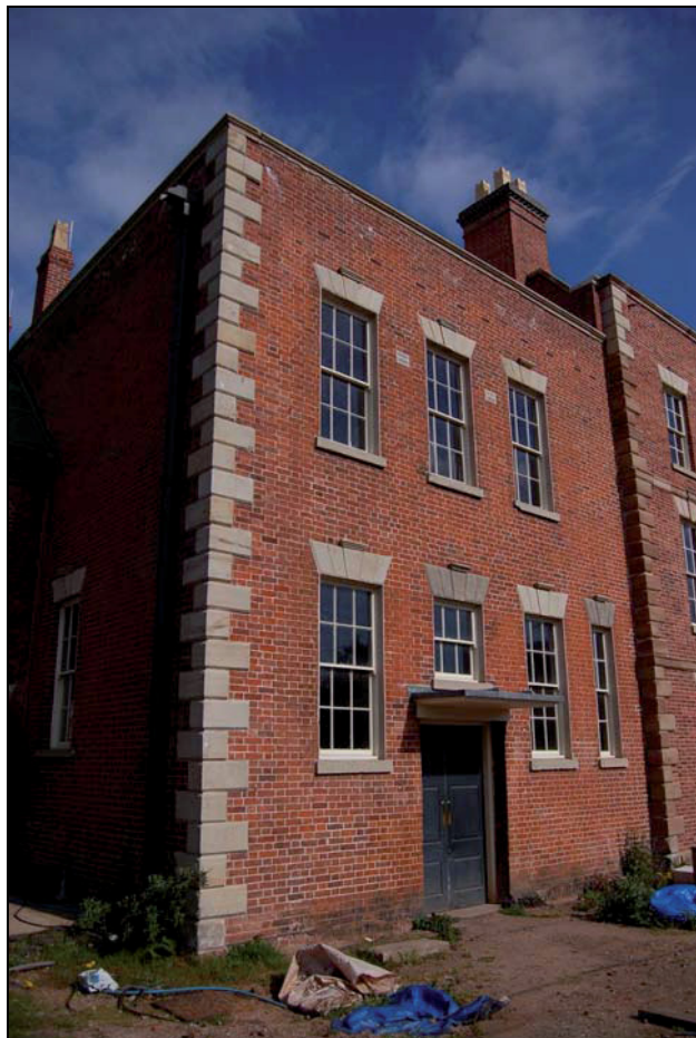
Plate 23: West Range, south elevation, view north
