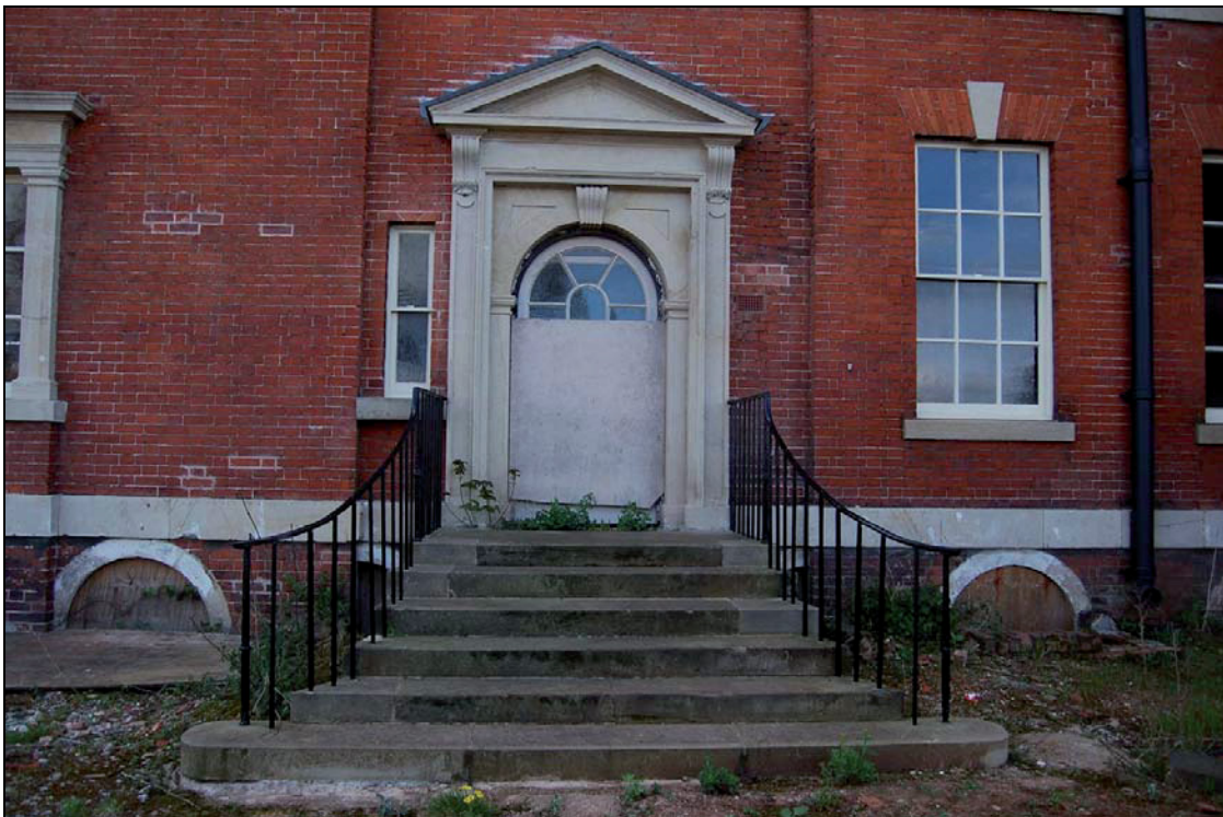
Plate 31: Garden Range north entrance and steps, view south-east
