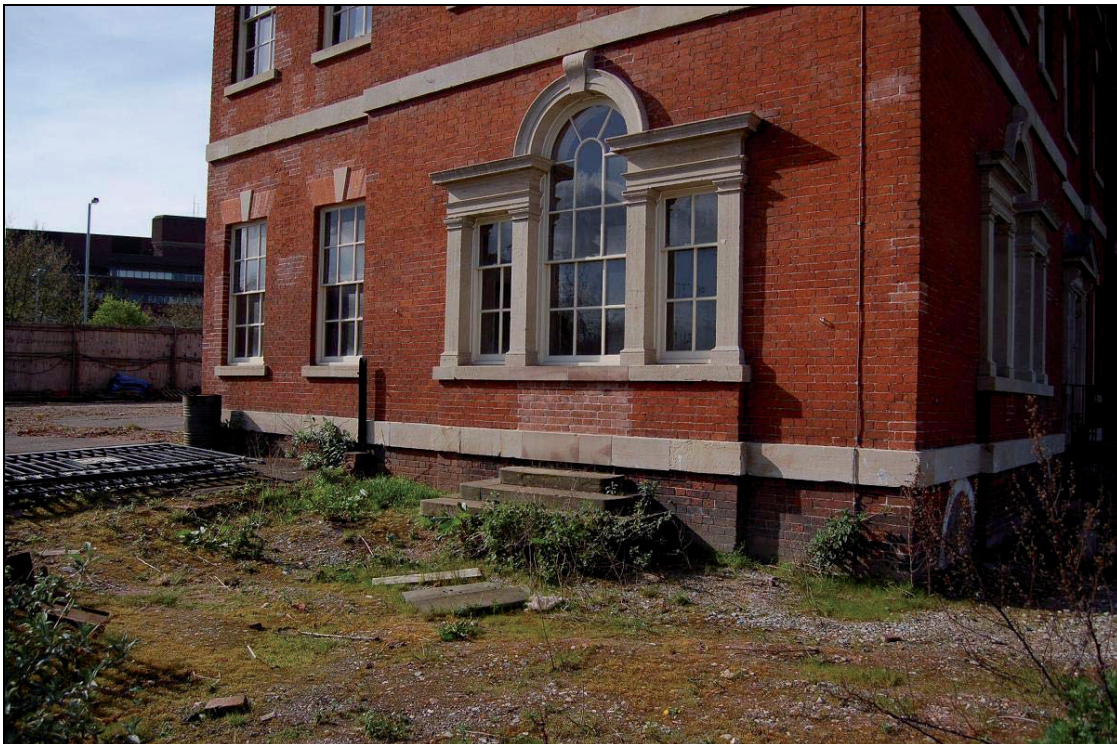
Plate 15: Garden Range, blocked doorway and steps in east elevation, view south
