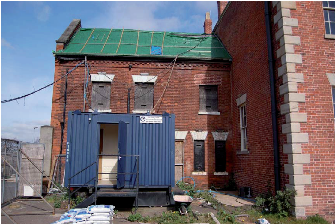
Plate 22: South elevation of North-West range, view north-west
