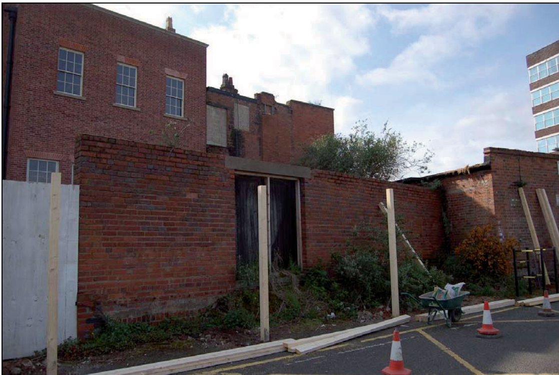
Plate 27: North of house, view south-south-west
