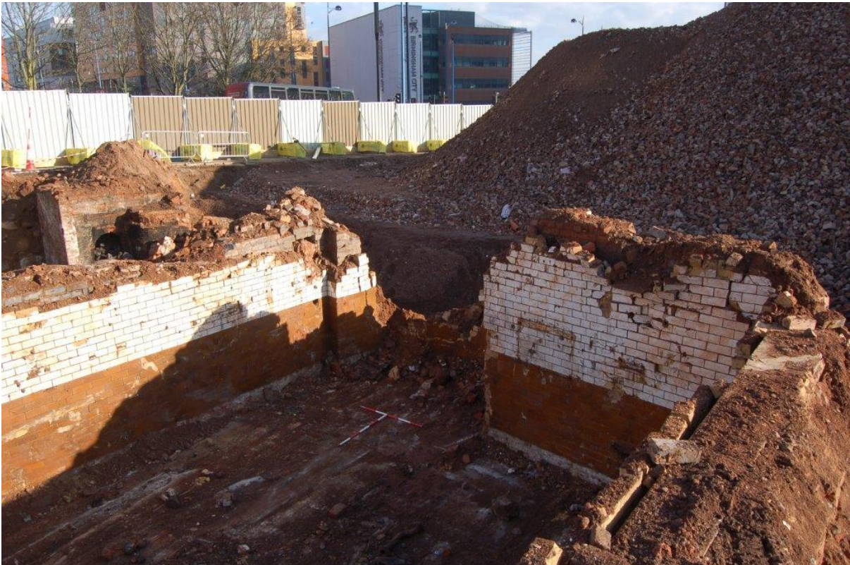
Plate 7: bay in south eastern end of building 2, 2 x 1m scale, facing east.
