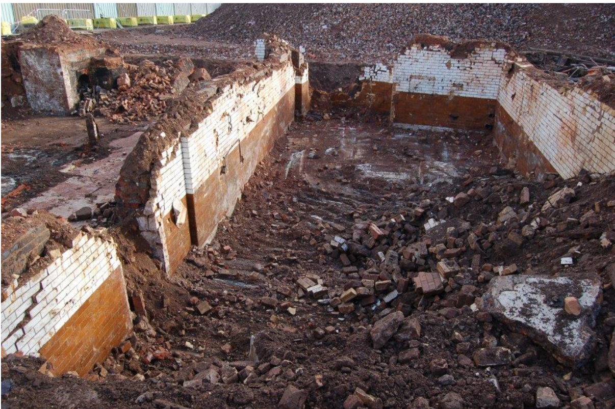
Plate 8: Building 2, facing south east.
