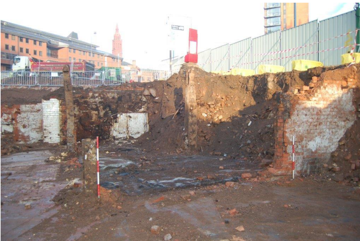
Plate 10: building 1, rooms 1B, 1C and 1D, showing wall (140) and its vertical steels, 2 x 1m scales, facing north.
