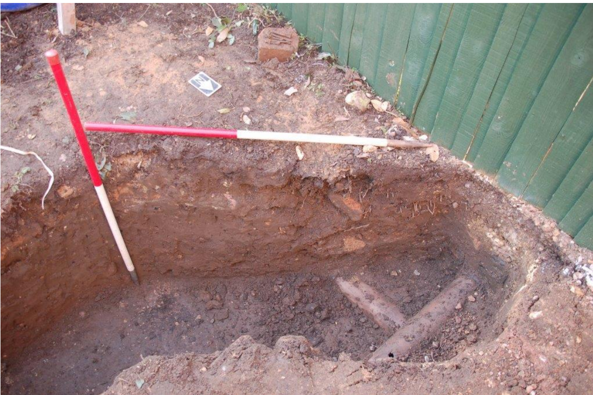
Plate 6 The garden soils and backfill from modern ceramic drains. View southwest. 2x1m scales.
