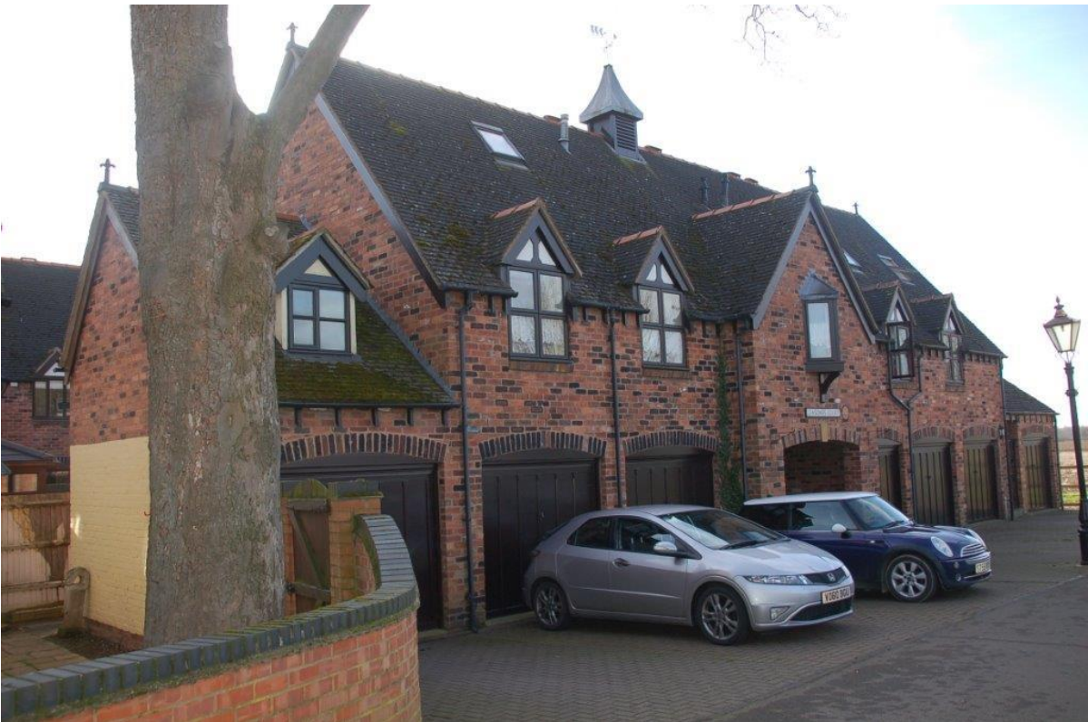
Plate 2 The northern frontage of Leasowes Court looking southwest.
