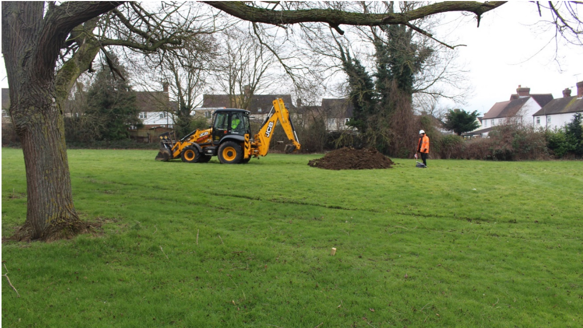
Plate 1: The site during opening of trenches
