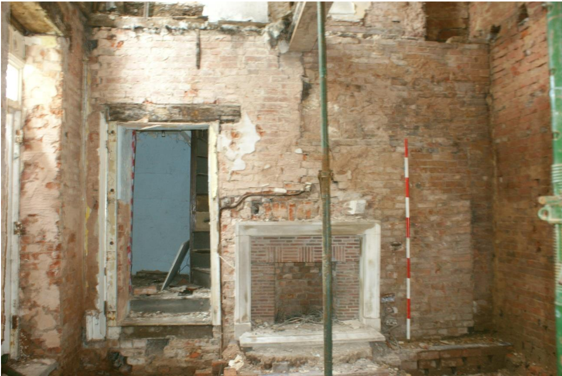
Plate 25 Phase 3 groundfloor parlour, looking north-west (2m scale)
