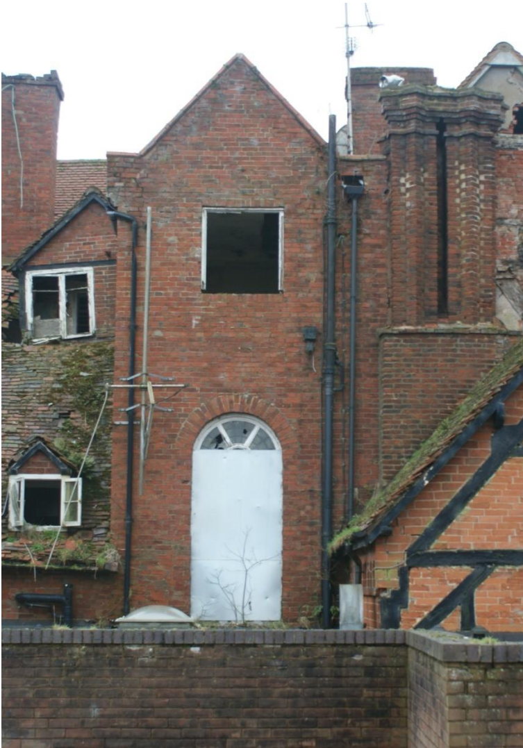
Plate 33 Phase 4 staircase housing structure, looking south-east
