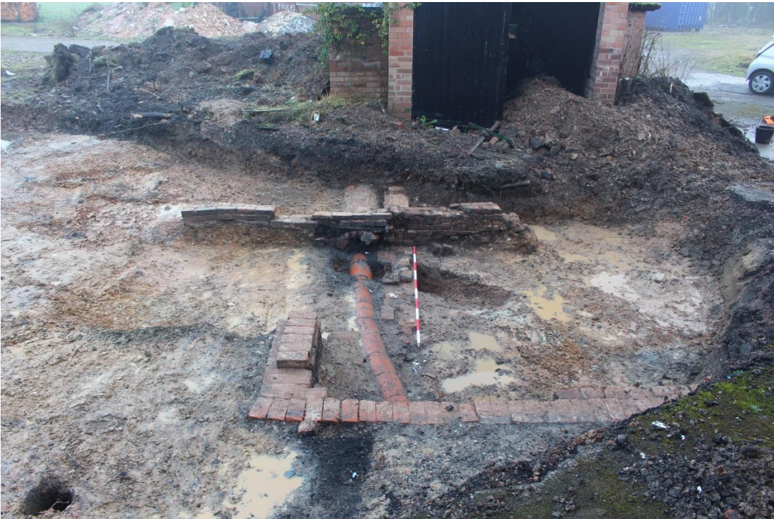
Plate 3 Excavation area overview with wall (1234) in the foreground, looking north-east (2m scale)
