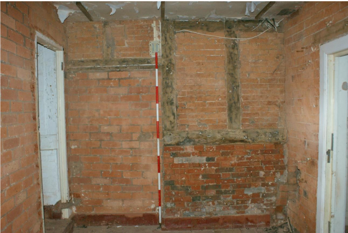
Plate 17 Phase 2 Frame 3, looking north-west (2m scale)
