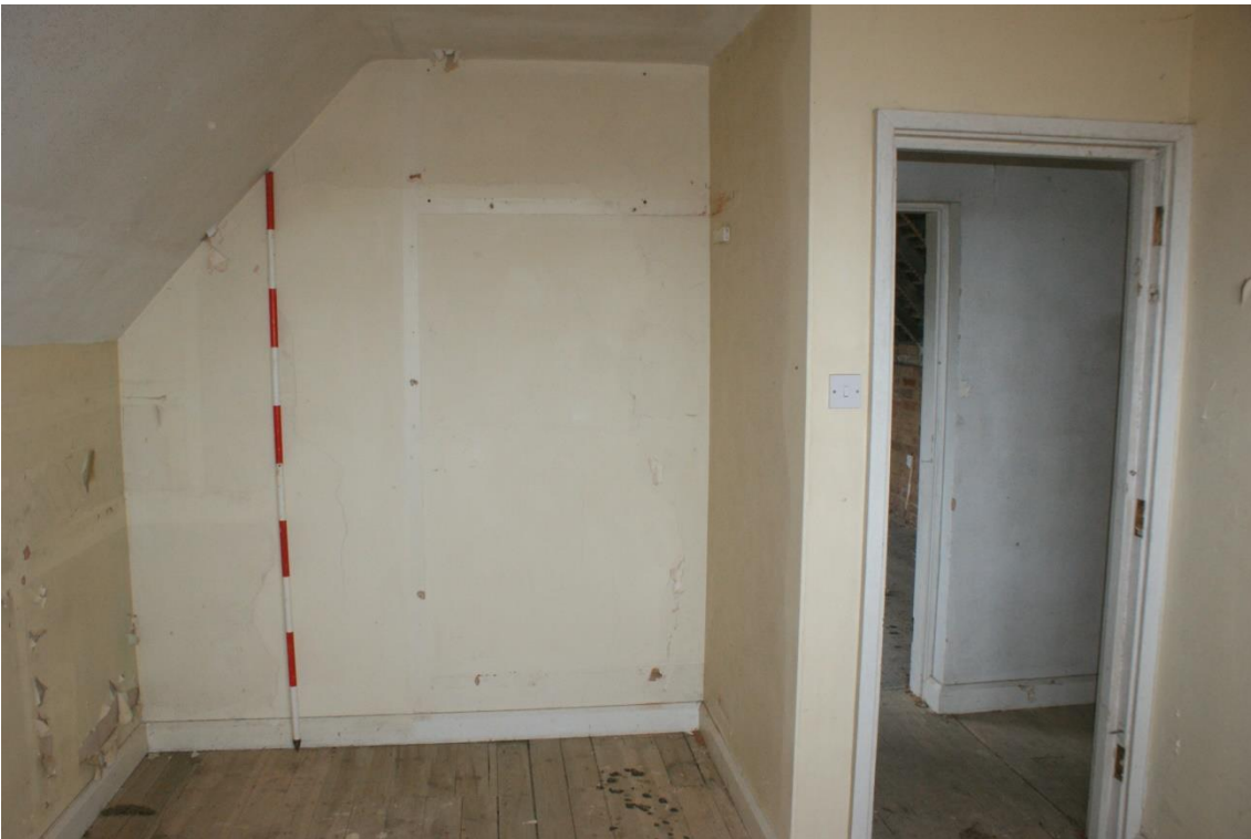
Plate 43 Phase 7 addition first floor, looking south-east (2m scale)
