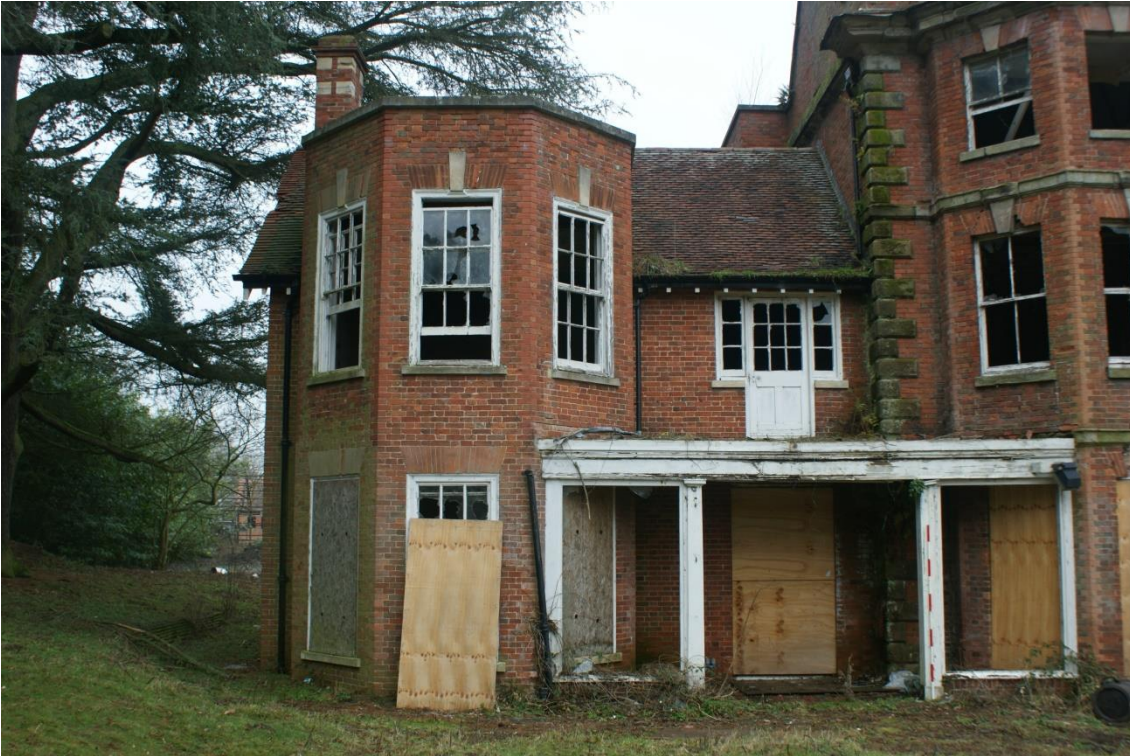
Plate 36 Phase 6 addition, looking north-west (2m scale)
