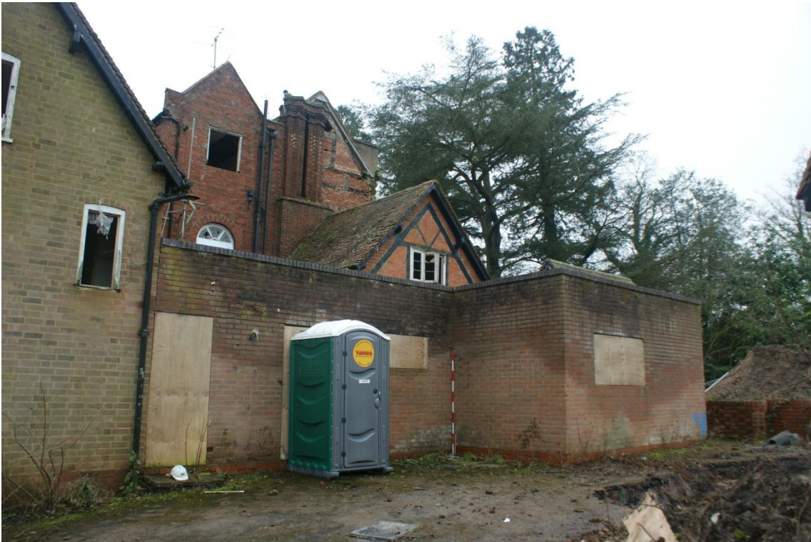
Plate 45 Phase 8 addition, looking south (2m scale)
