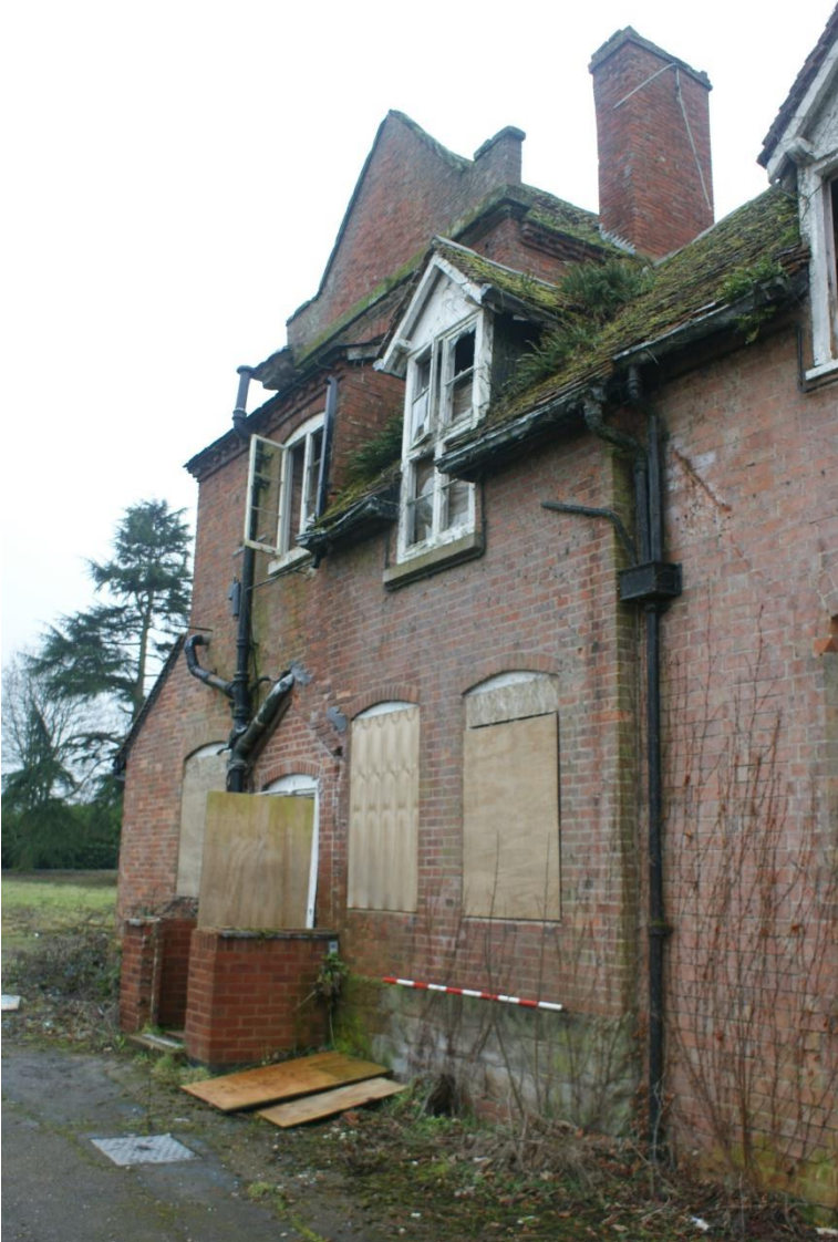
Plate 21 Potetial Phase 3 structure, looking south (2m scale)
