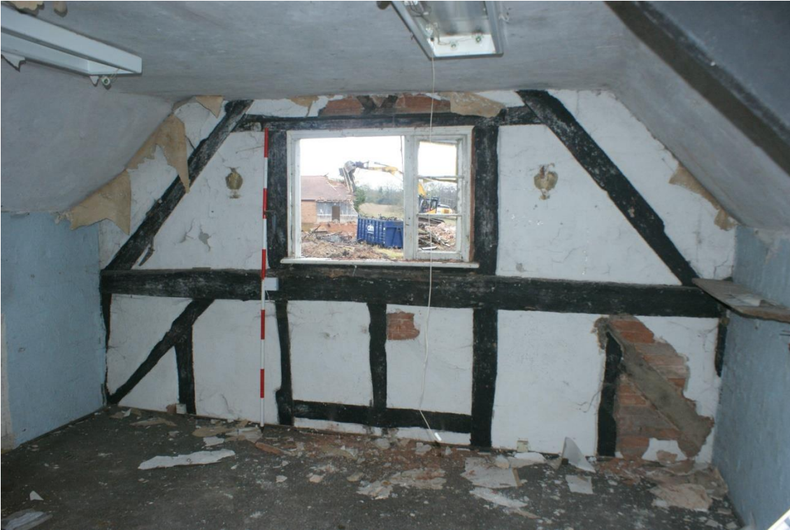
Plate 16 Phase 2 Frame 3, looking north-west (2m scale)
