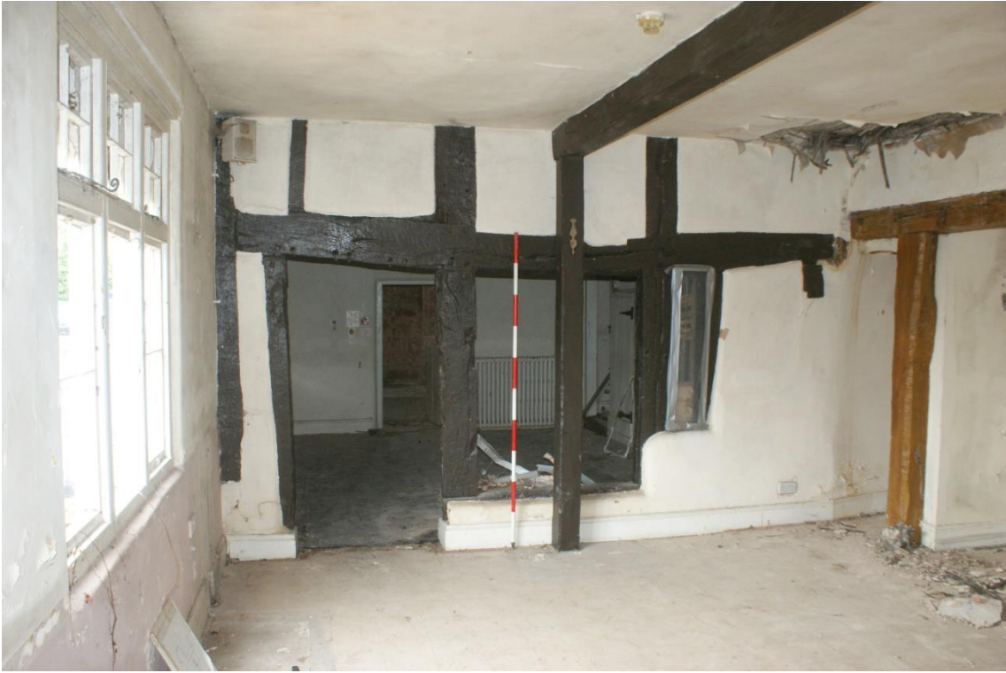
Plate 15 Phase 1 Frame 2, looking south-east (2m scale)
