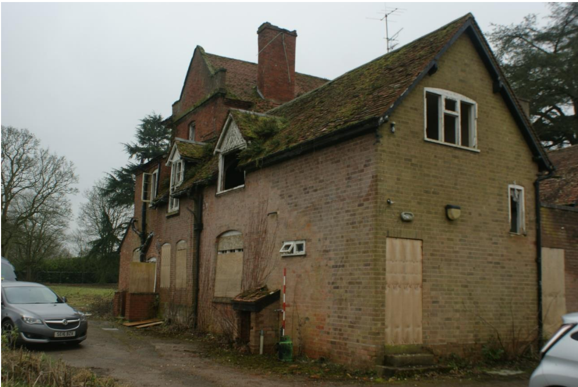
Plate 41 Phase 7 addition, looking south (2m scale)
