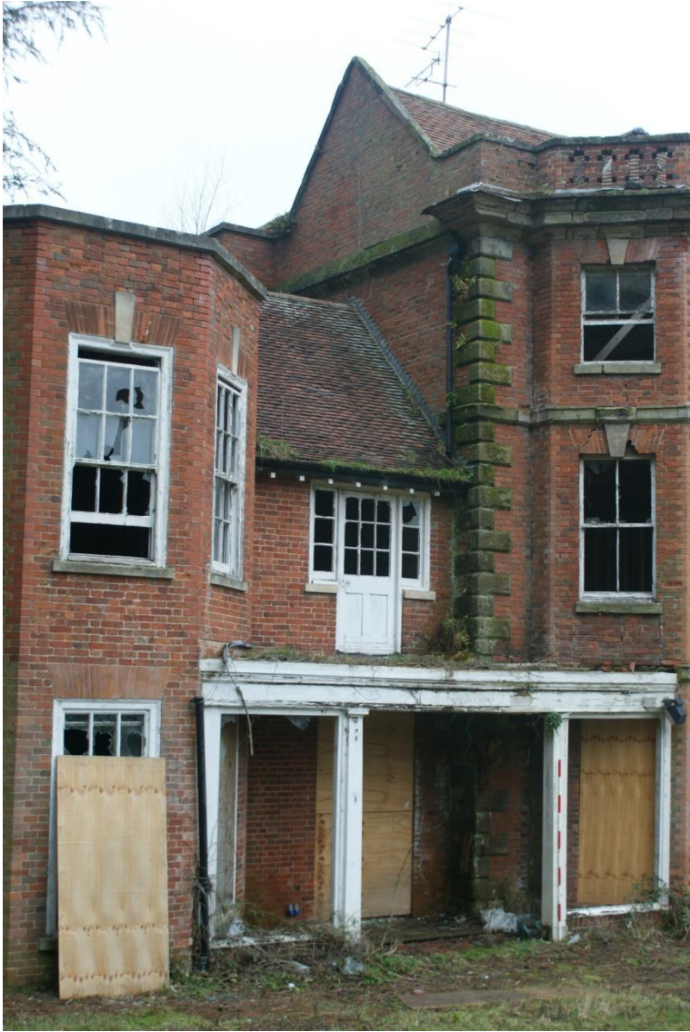
Plate 19 Phase 3 gable end, looking north (2m scale)
