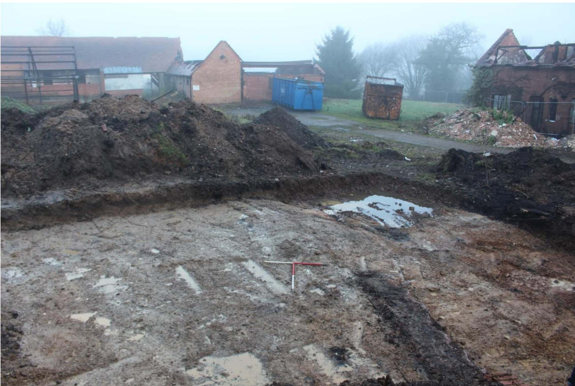
Plate 2 Excavation area with natural deposits visible, looking north (2x1m scale)
