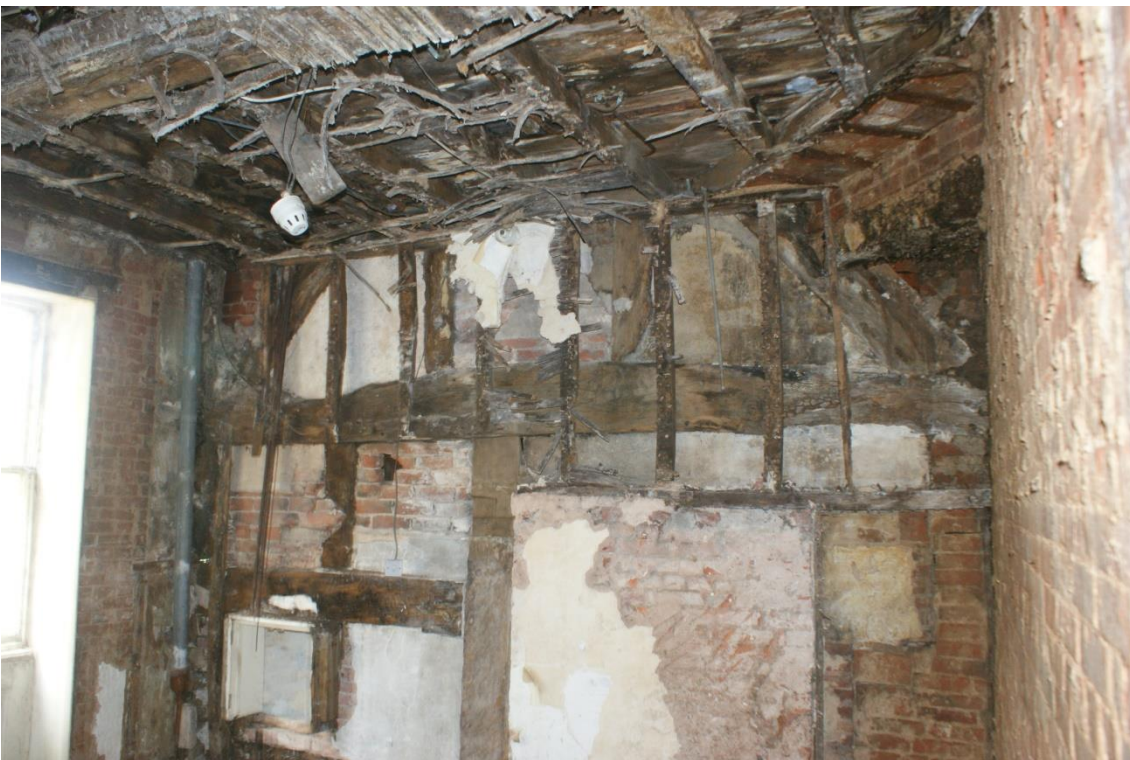
Plate 12 Phase 1 Frame 1 rear, looking north-west
