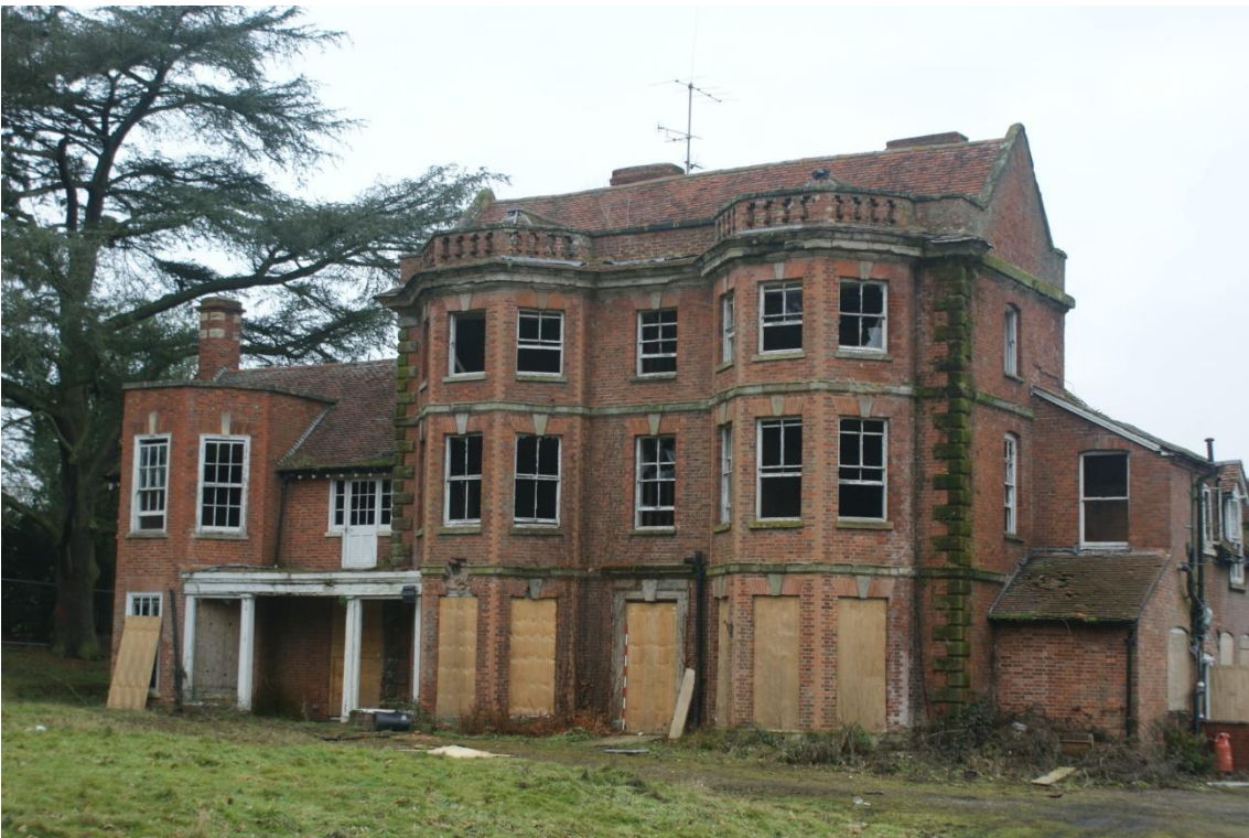
Plate 8 Aylesbury House facade, looking north-west (2m scale)
