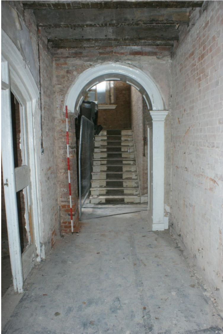
Plate 22 Phase 3 groundfloor hallway, looking north-west (2m scale)
