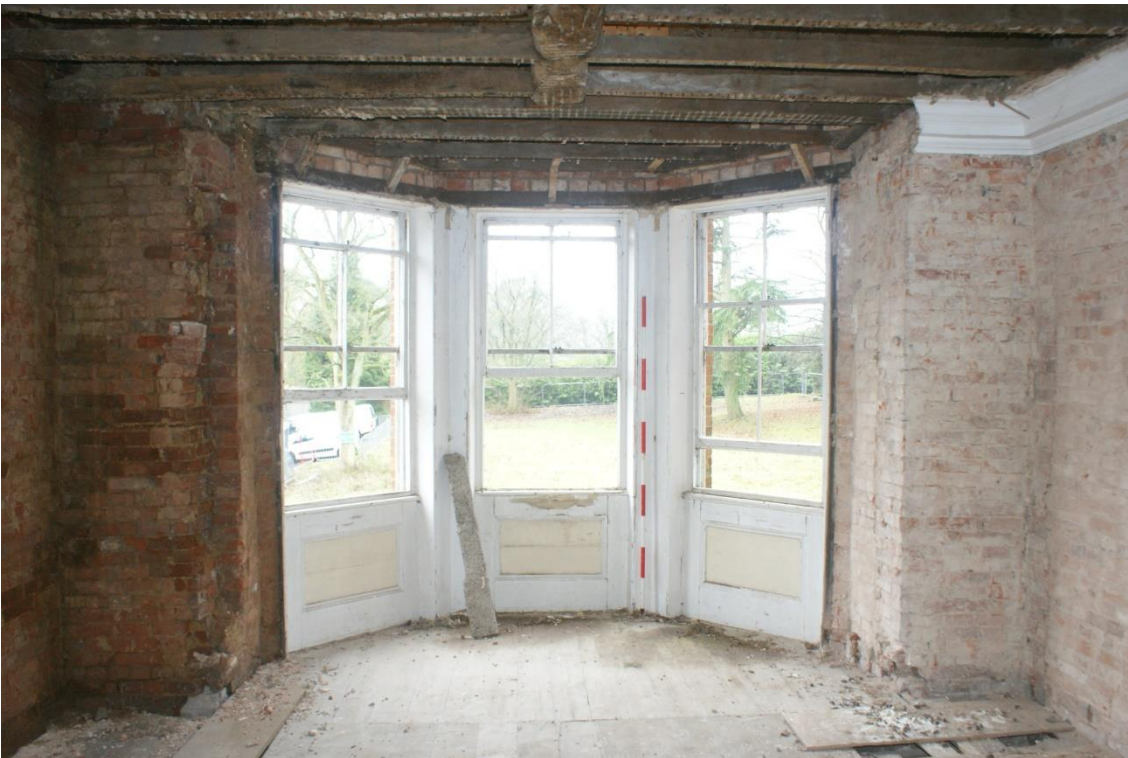
Plate 28 Phase 3 first floor chamber, looking south-east (2m scale)
