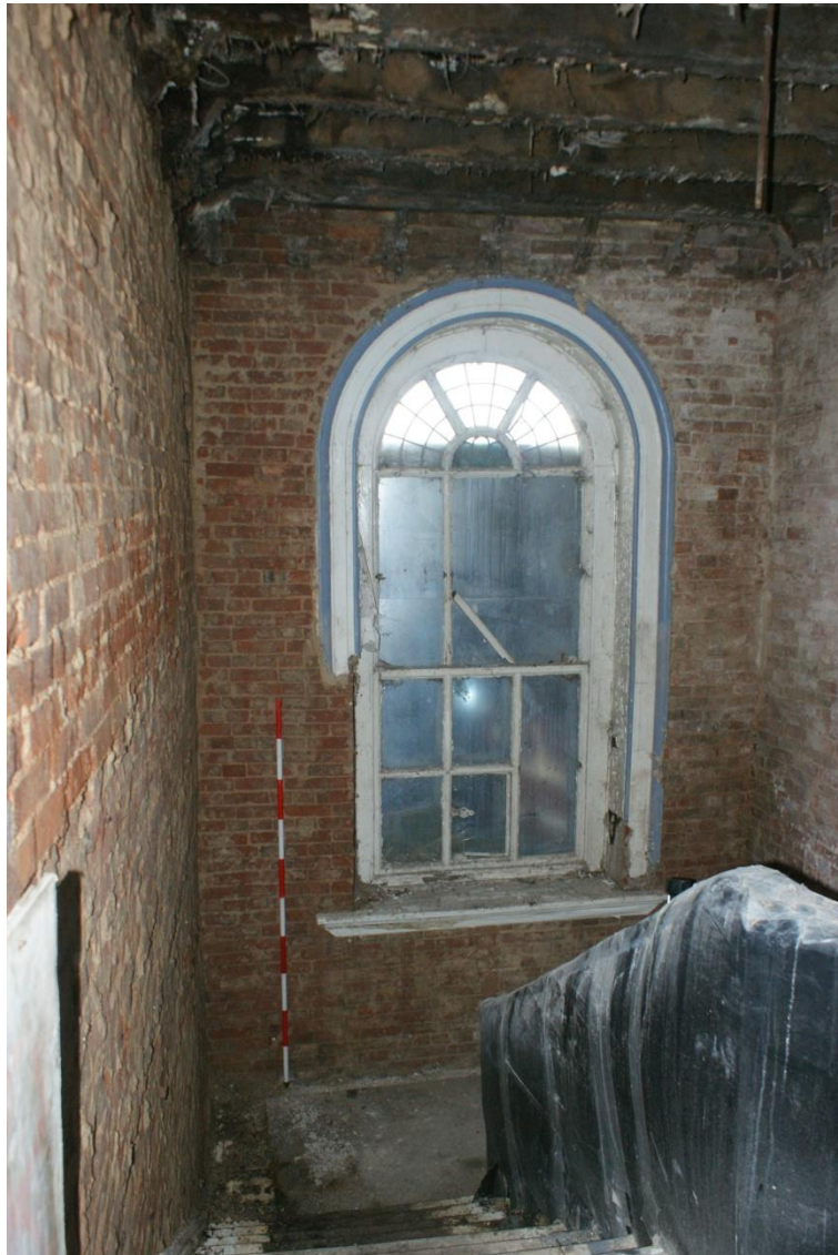
Plate 35 Phase 4 staircase, looking north-west (2m scale)
