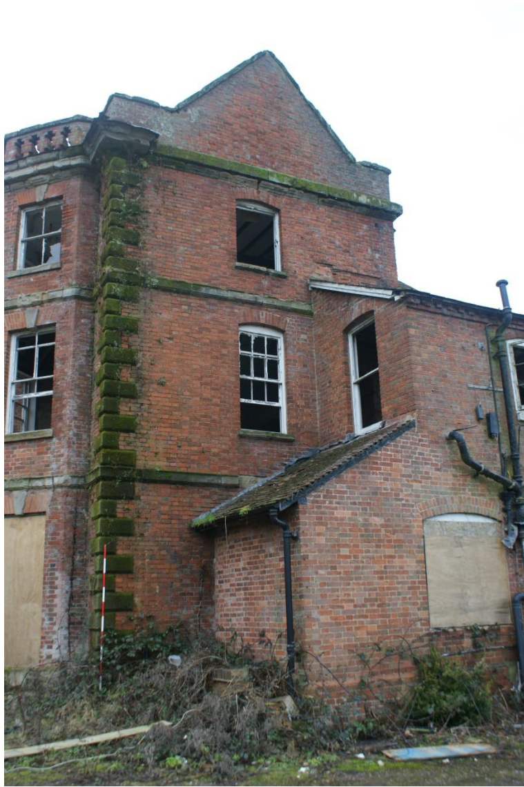
Plate 18 Phase 3 gable end, looking west (2m scale)
