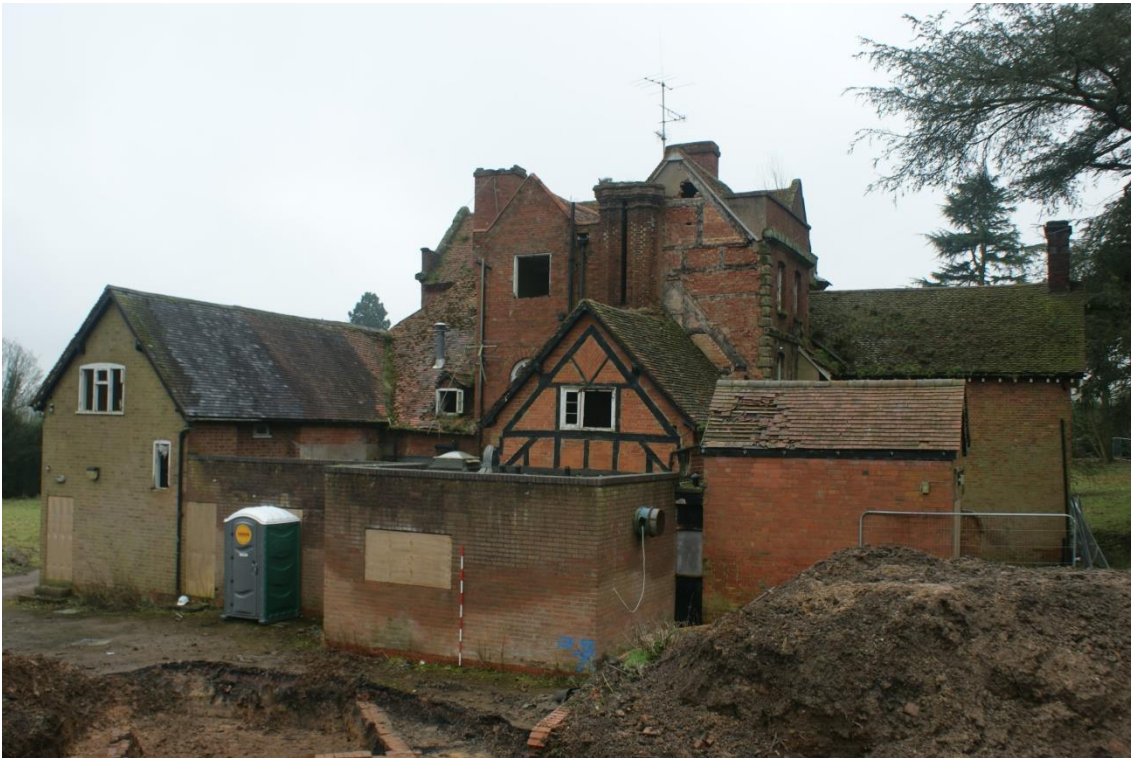
Plate 9 Aylesbury House rear view, looking south-east (2m scale)
