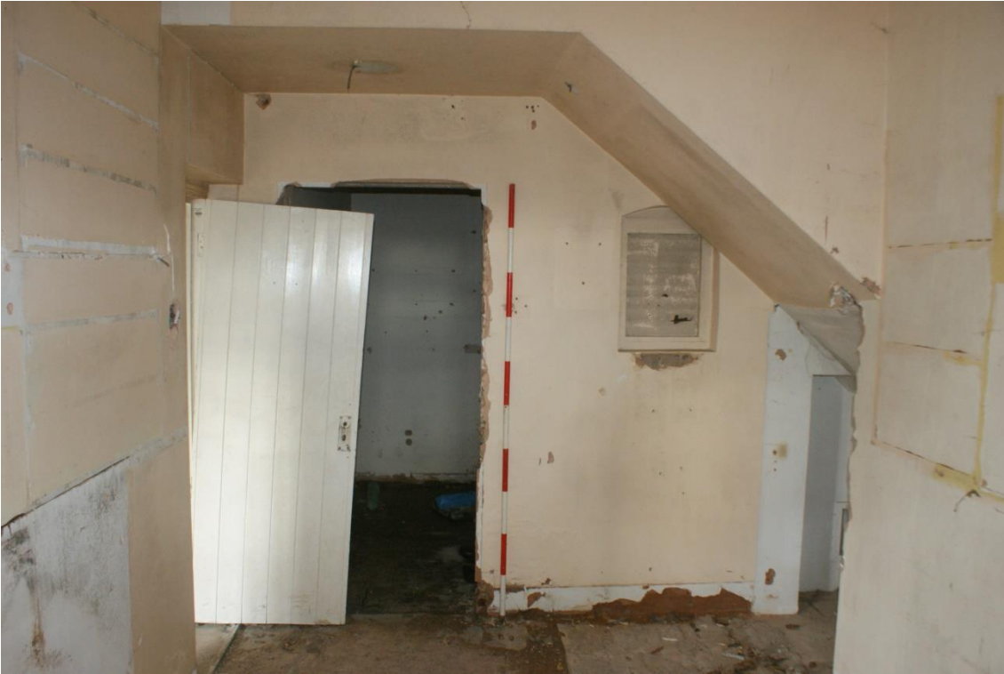
Plate 42 Phase 7 addition ground floor, looking south-west (2m scale)
