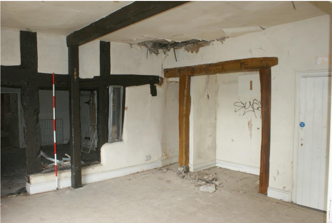
Plate 27 Phase 3 brewhouse, looking south-west (2m scale)
