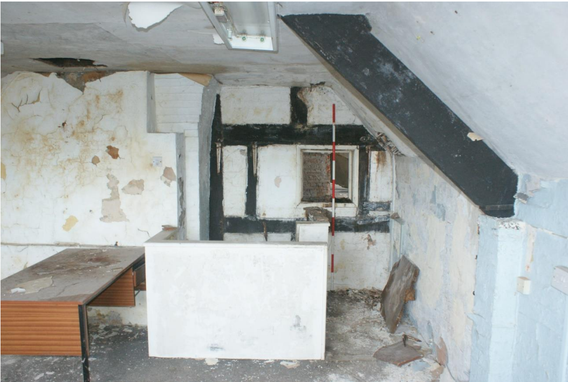
Plate 11 Phase 1 Frame 1, looking south-east (2m scale)
