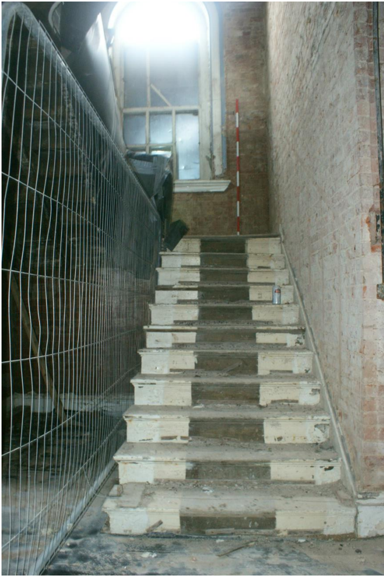
Plate 34 Phase 4 staircase, looking north-west (2m scale)
