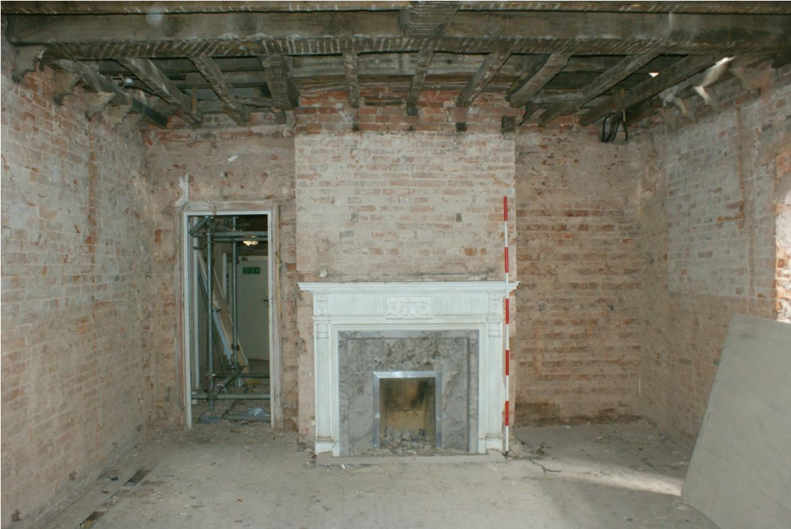
Plate 23 Phase 3 groundfloor dining room, looking north-west (2m scale)
