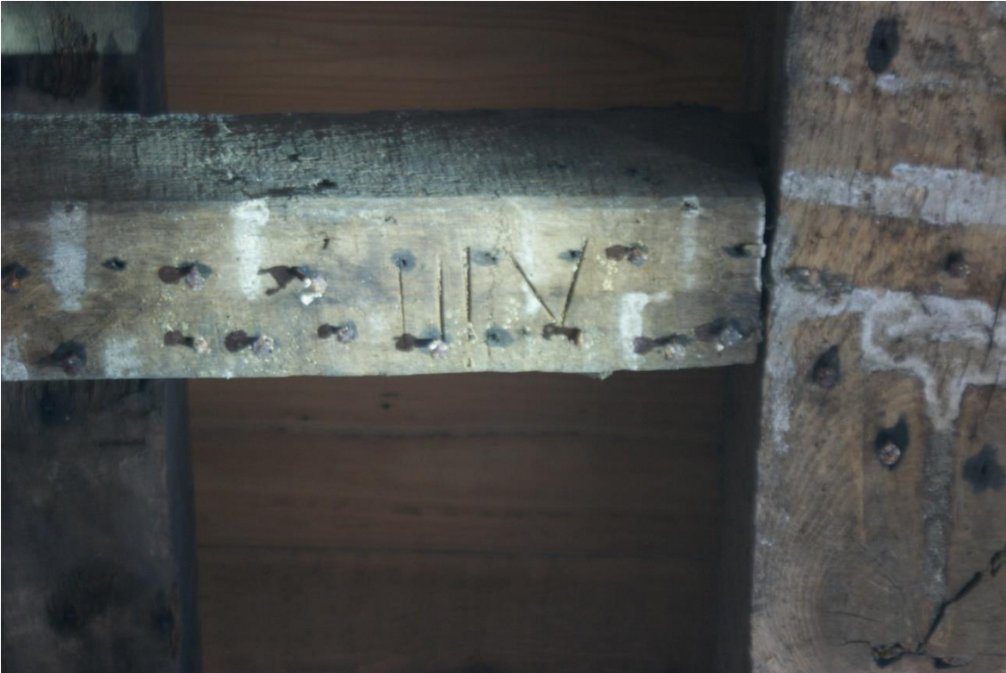
Plate 31 Phase 3 carpenters mark on a floor joist
