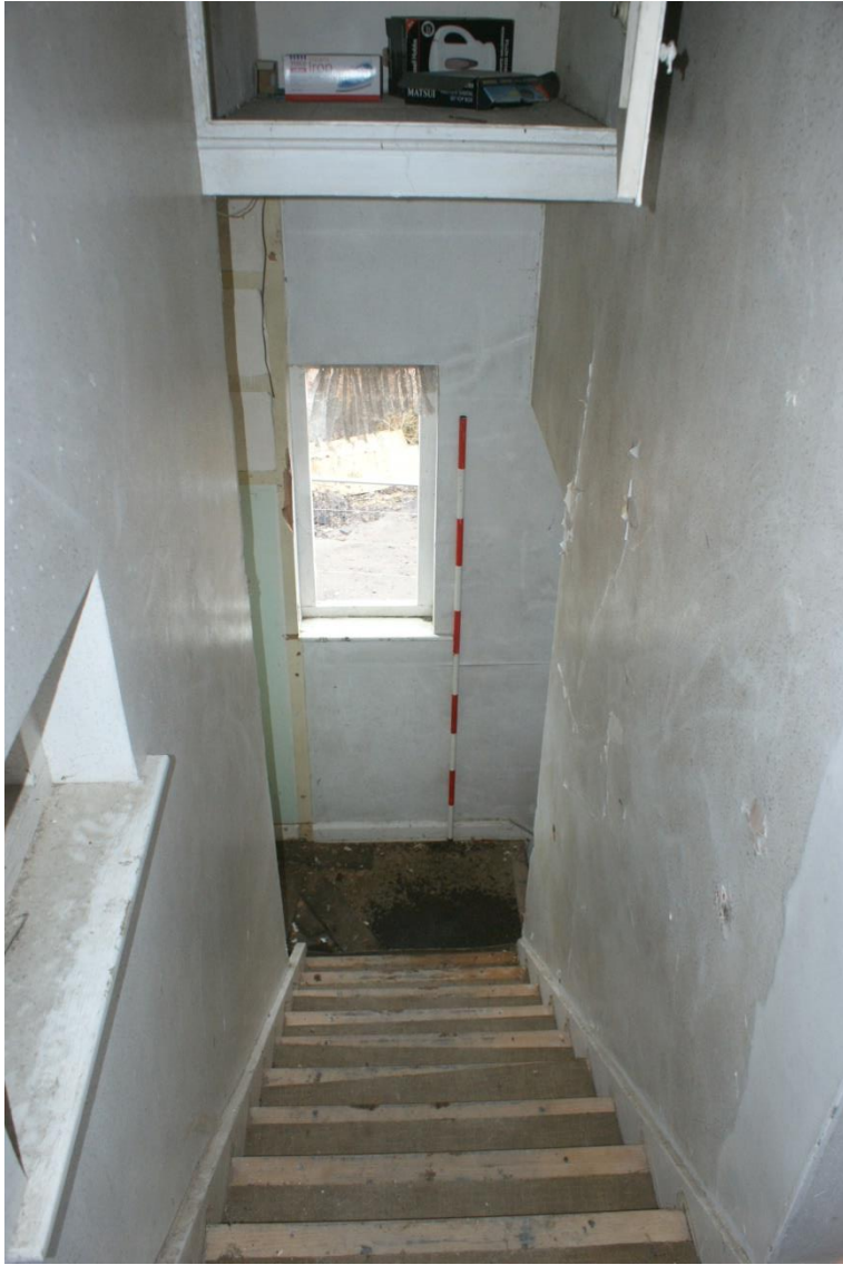
Plate 44 Phase 7 addition stairs, looking north-west (2m scale)
