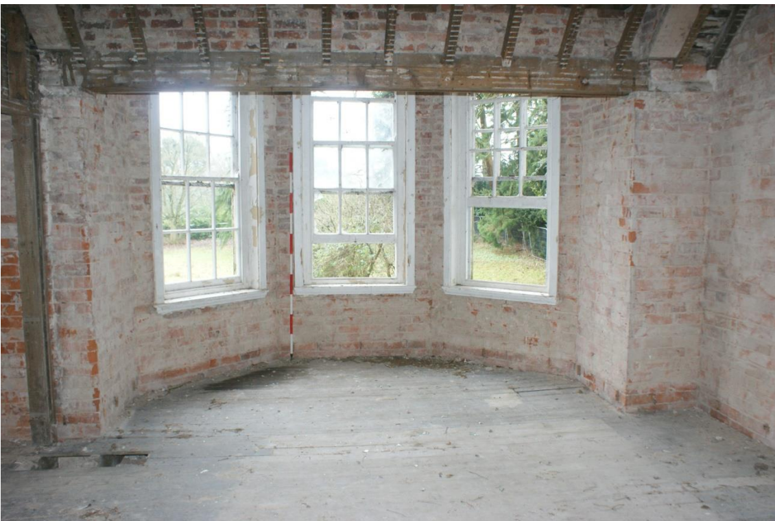
Plate 39 Phase 6 addition first floor, looking south-east (2m scale)
