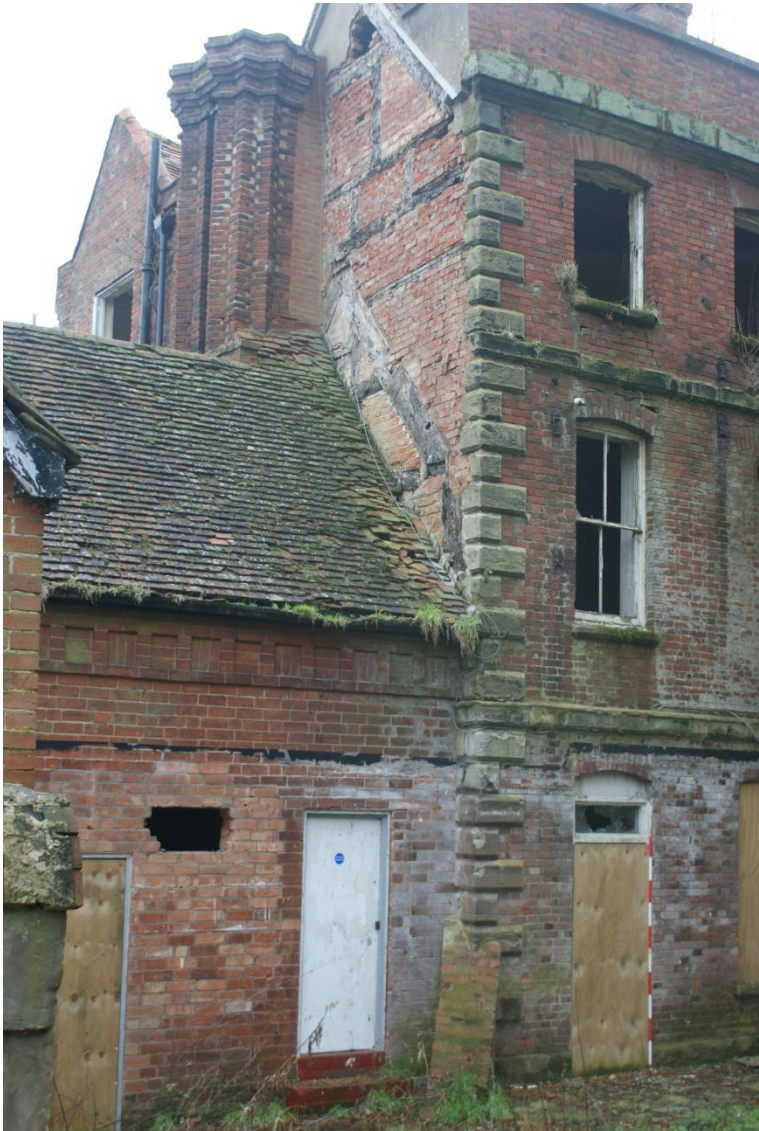
Plate 10 Phase 1 Frame 1, looking east (2m scale)
