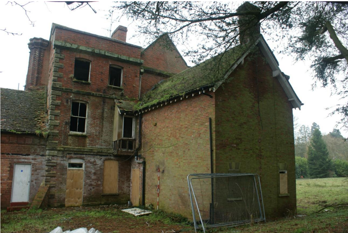
Plate 37 Phase 6 addition, looking east (2m scale)
