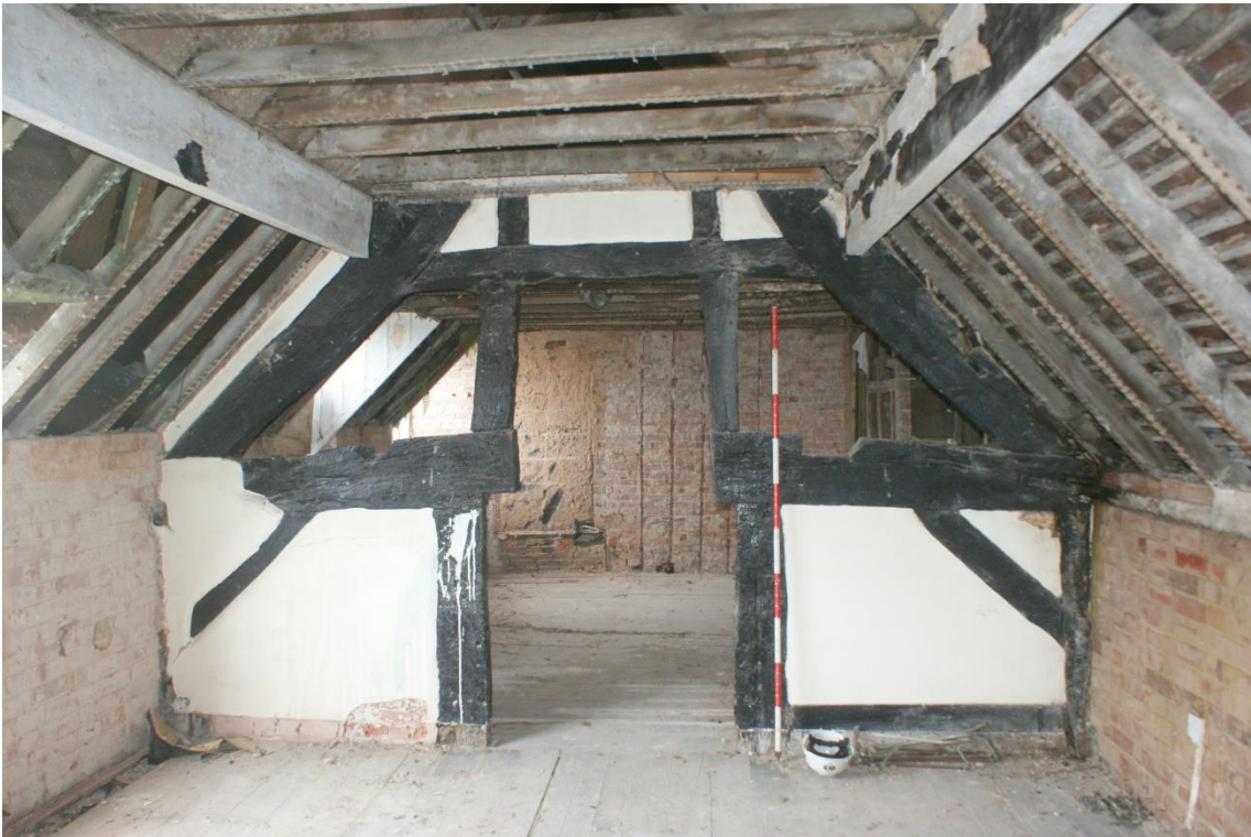
Plate 14 Phase 1 Frame 2, looking south-east (2m scale)
