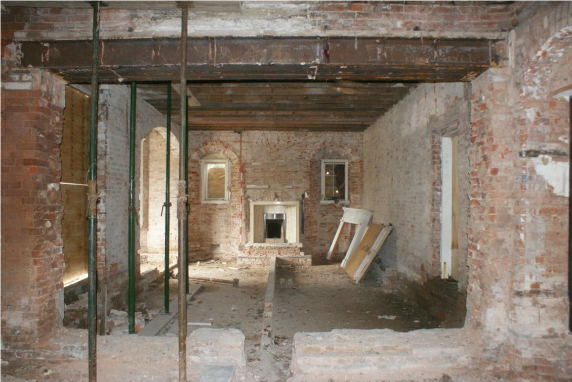
Plate 38 Phase 6 addition ground floor, looking south-west (2m scale)
