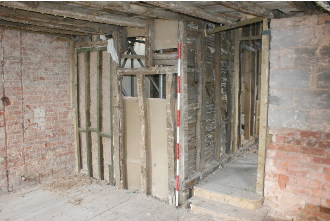
Plate 32 Possible Phase 3 light stud division, looking south-west (2m scale)
