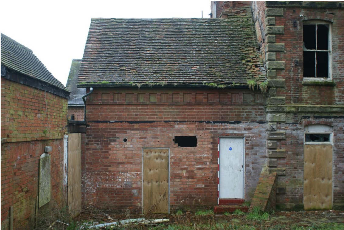
Plate 40 Phase 6 rebuild of the Phase 2 structure, looking north-east (2m scale)
