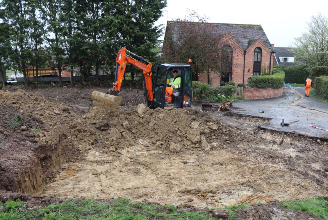
Plate 1 The site, looking south east
