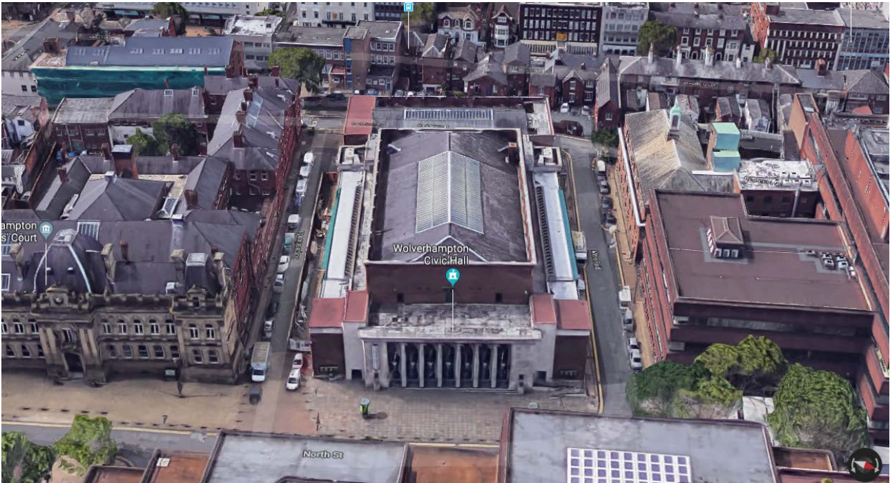
Plate 1 A 3D view of the Civic Hall, looking west (Google Maps https://www.google.co.uk/maps/@52.5870048,-2.1286965,94a,35y,250.88h,54.99t/data=!3m1!1e3 accessed 1 June 2018)
