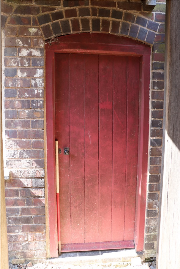
Plate 12 Exterior ground door detail, view south-west, 1m scale
