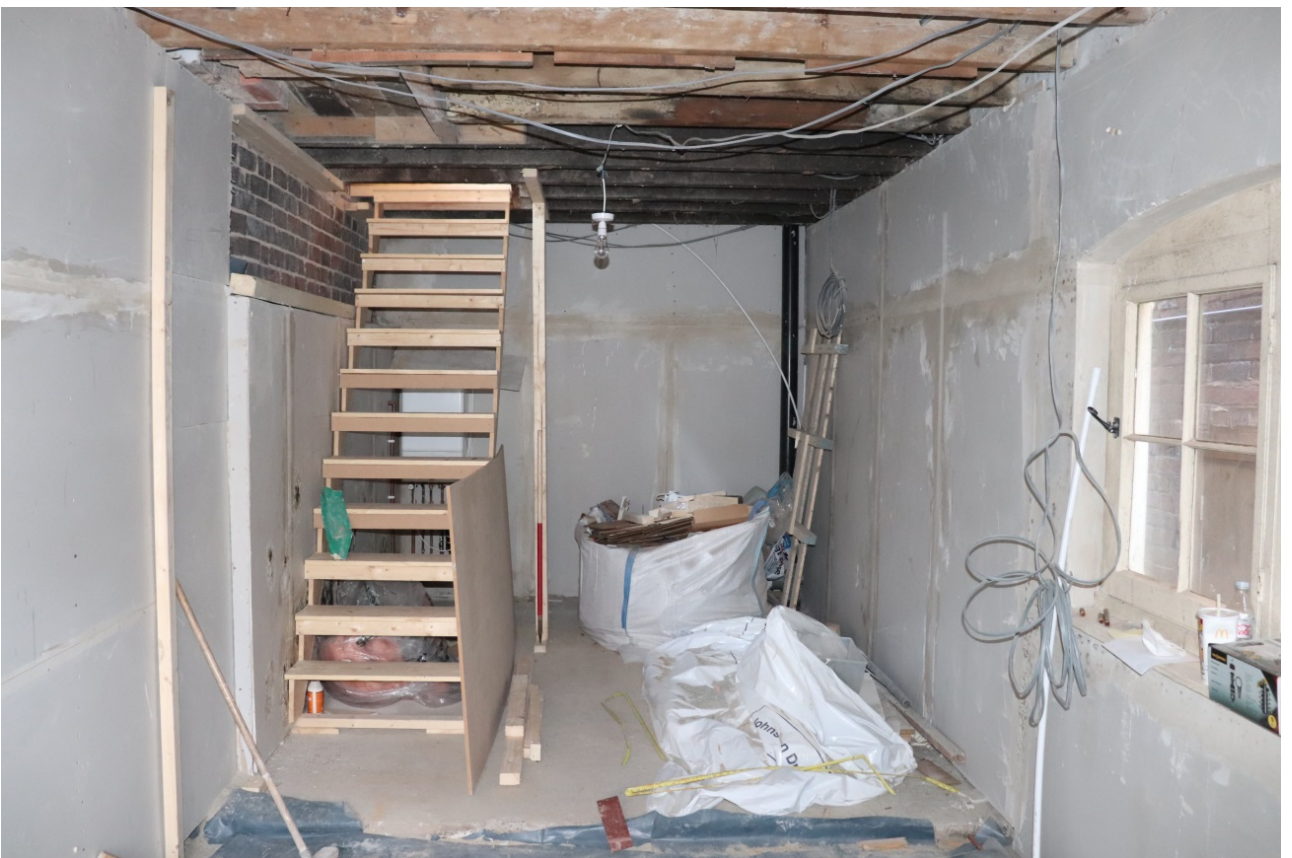
Plate 4 Ground floor interior, view south-west, 1m scale
