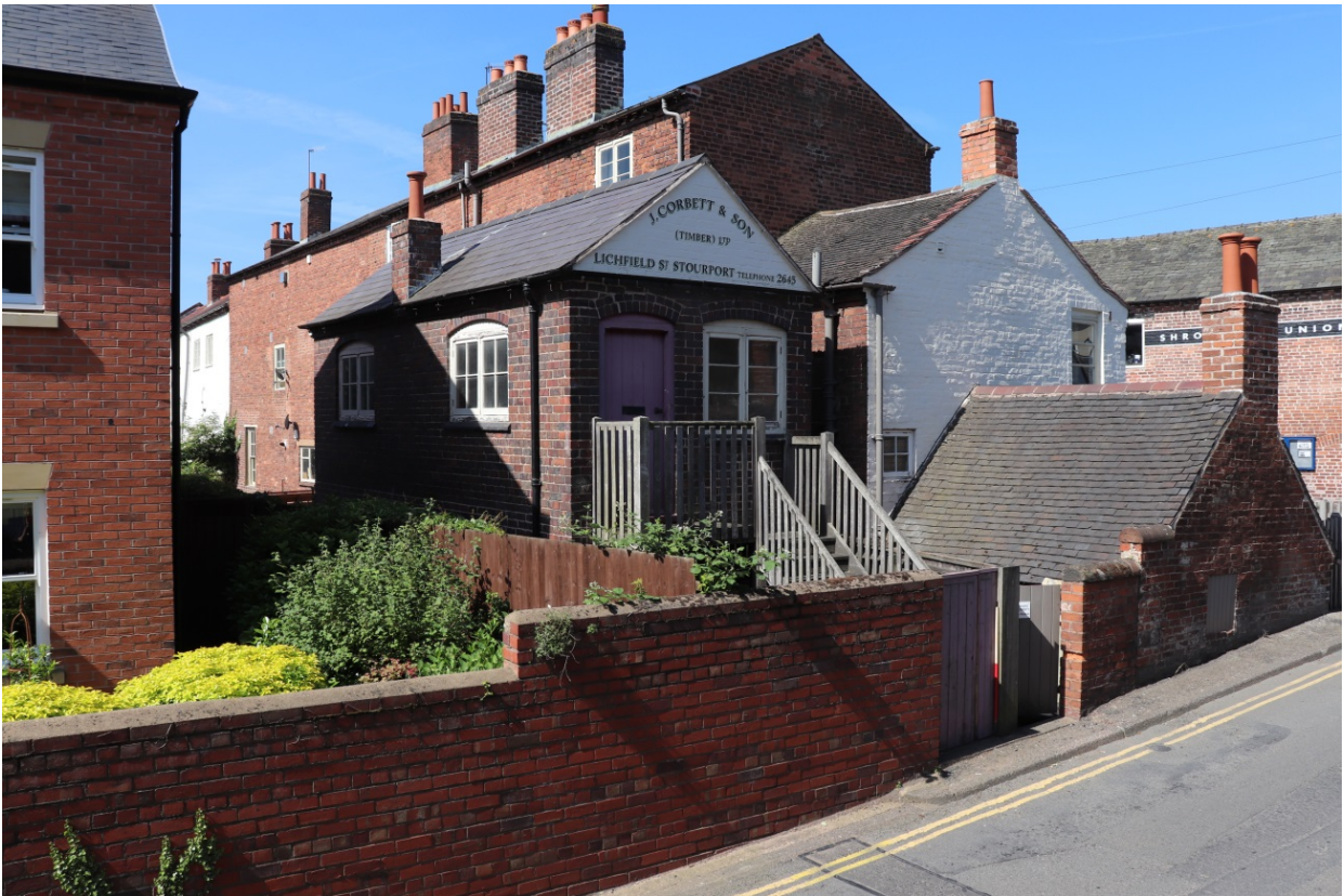
Plate 1 General view south-west, 1m scale
