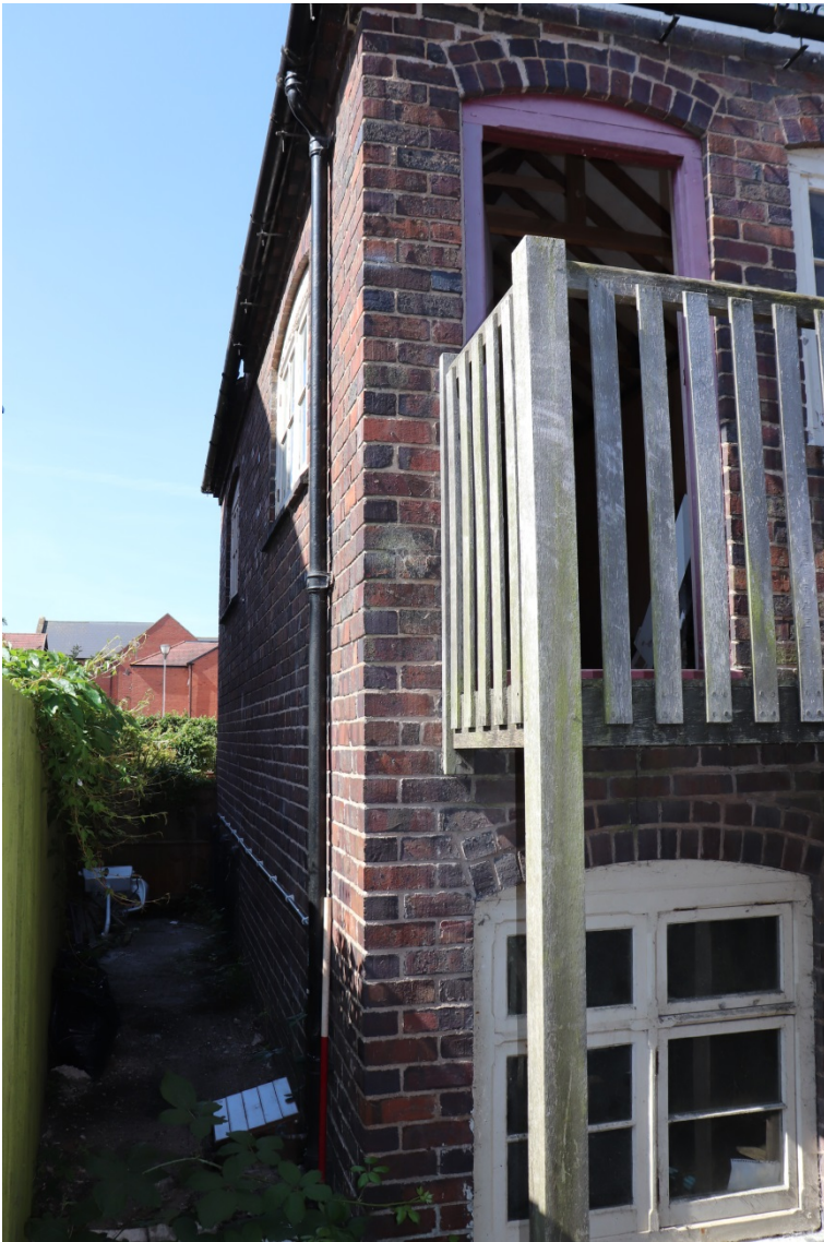
Plate 15 Exterior ground floor, looking south-west (left), 1m scale
