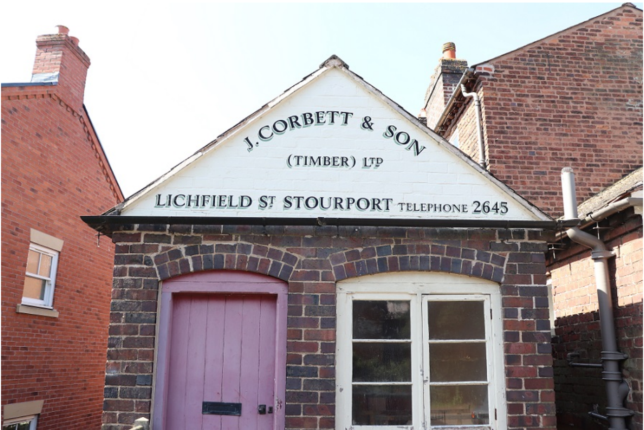
Plate 10 J Corbett and Son (Timber) Ltd sign on the north gable end, no scale
