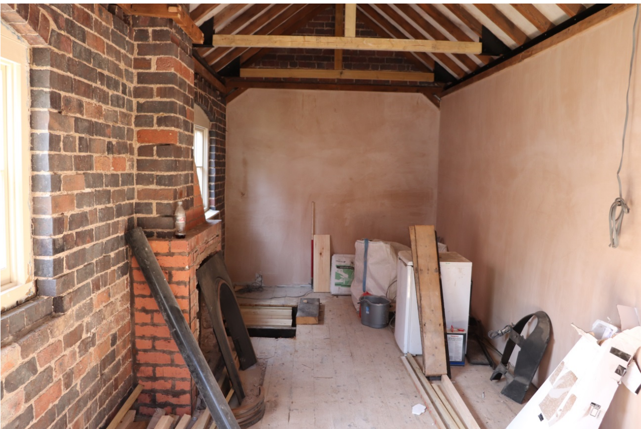
Plate 6 First floor interior, view south-west, 1m scale
