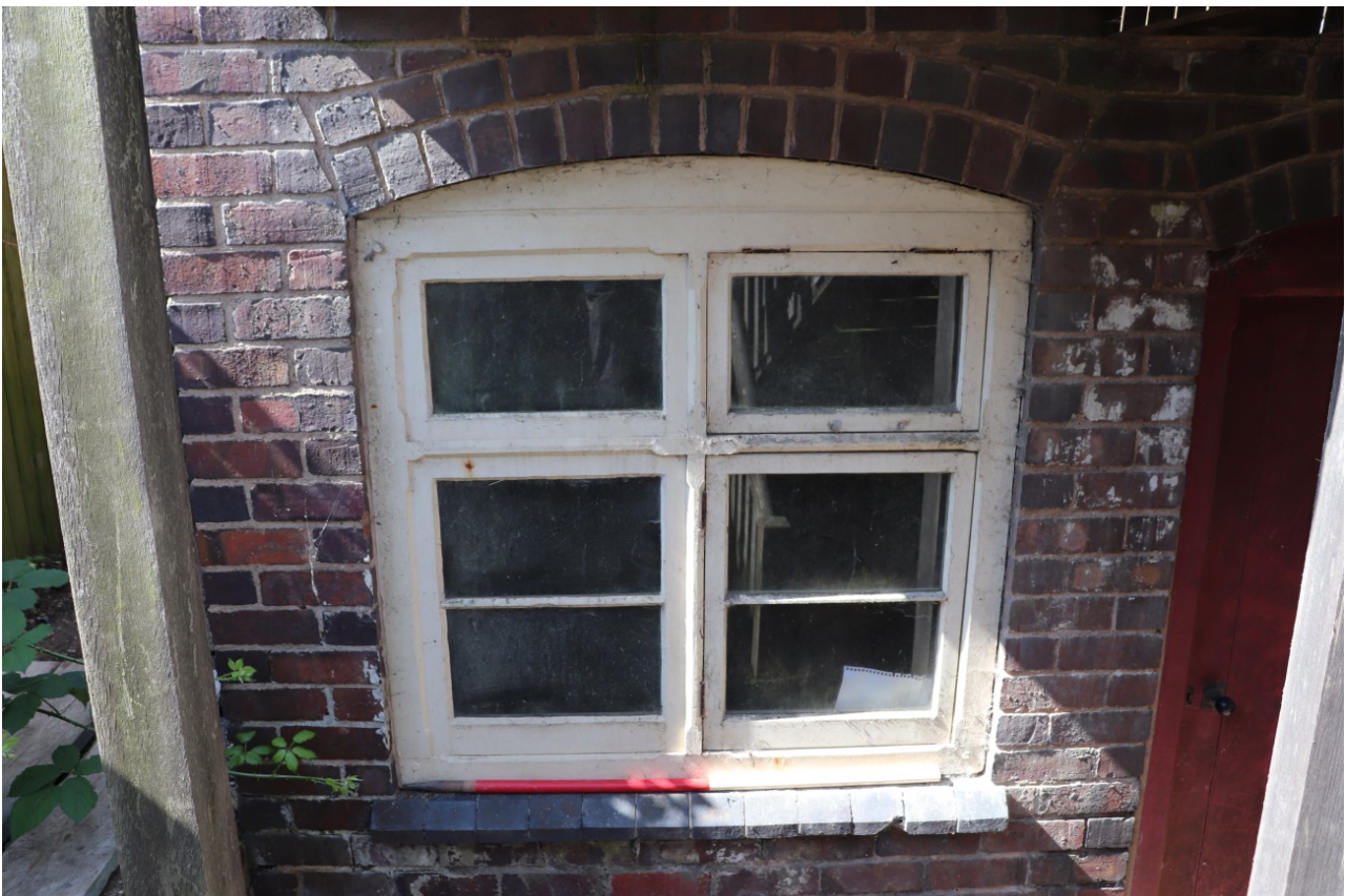
Plate 11 Exterior ground floor window detail, view south-west, 1m scale
