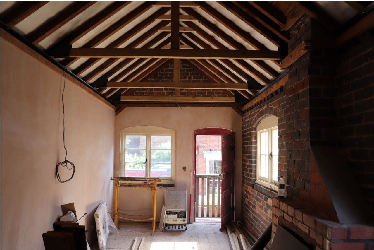
Plate 5 First floor interior, view north-east, 1m scale
