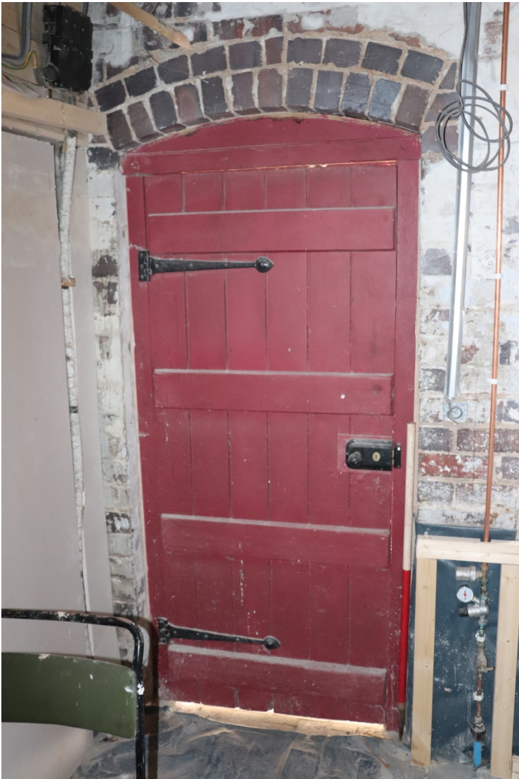
Plate 13 Interior ground floor door detail, view north, 1m scale
