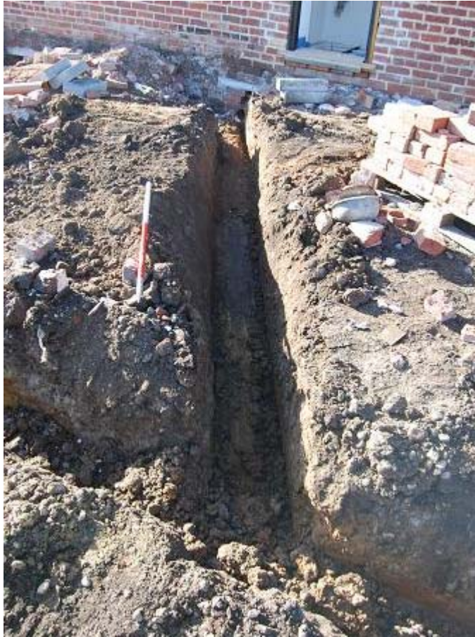
Plate 18: Detailed view of Trench 17, looking south west
