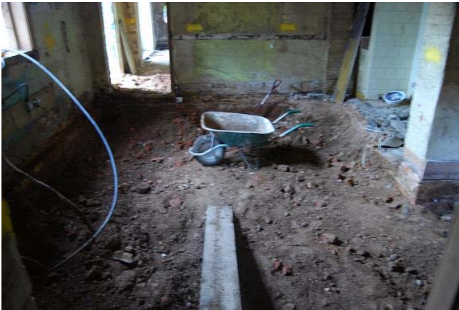
Plate 2: Trench 2 in Grove House, looking south west
