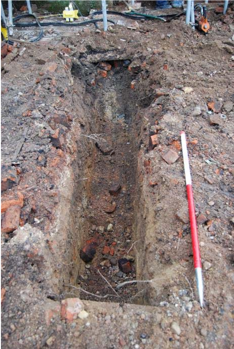
Plate 15: Detailed view of Trench 15, looking west
