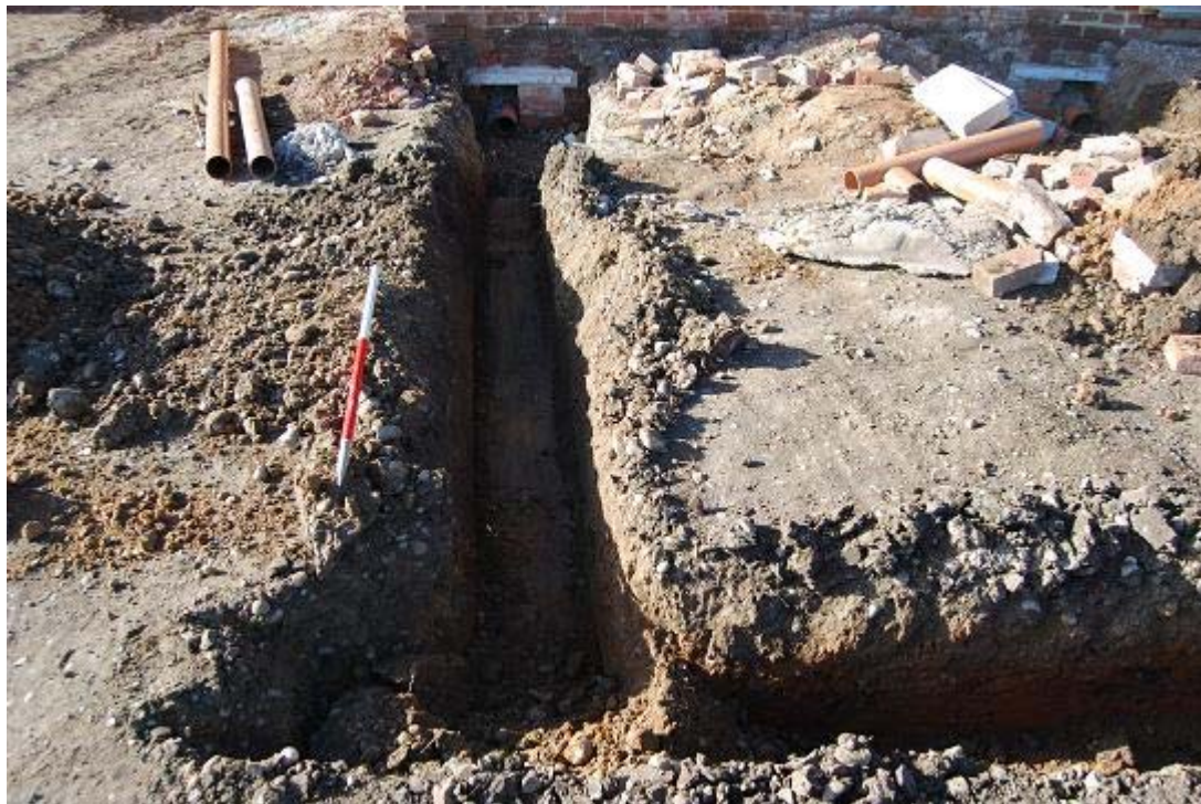
Plate 17: Detailed view of Trench 16, looking south west
