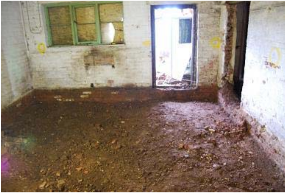
Plate 1: Trench 1 in Grove House, looking north
