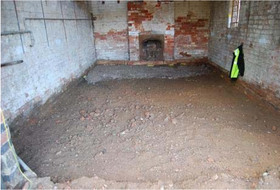
Plate 7: Trench 8 in the Coach House, looking west
