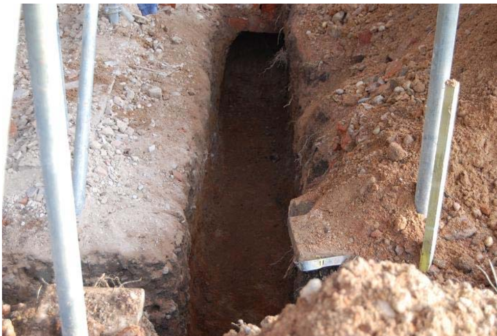
Plate 14: Detailed view of Trench 13, looking south
