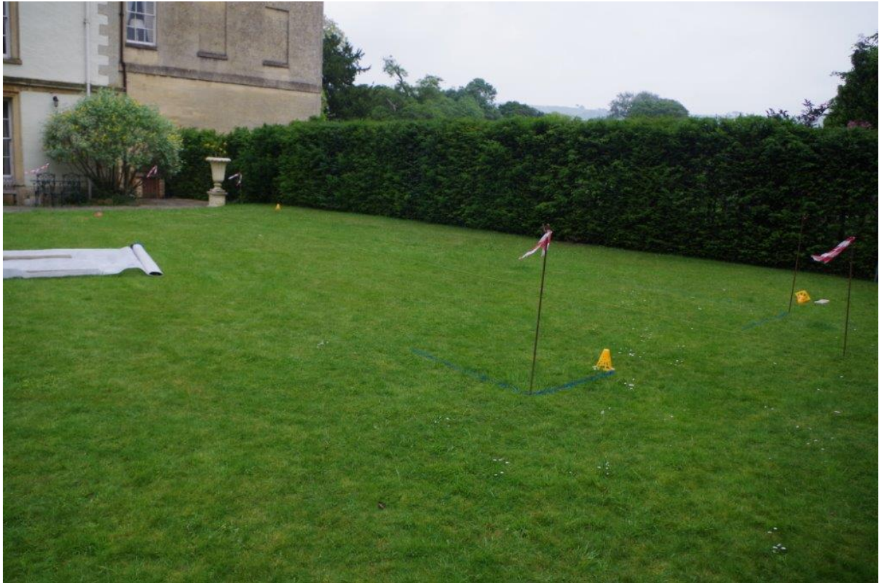
Plate 1: The marked out area of the groundworks, looking north-east, no scale
