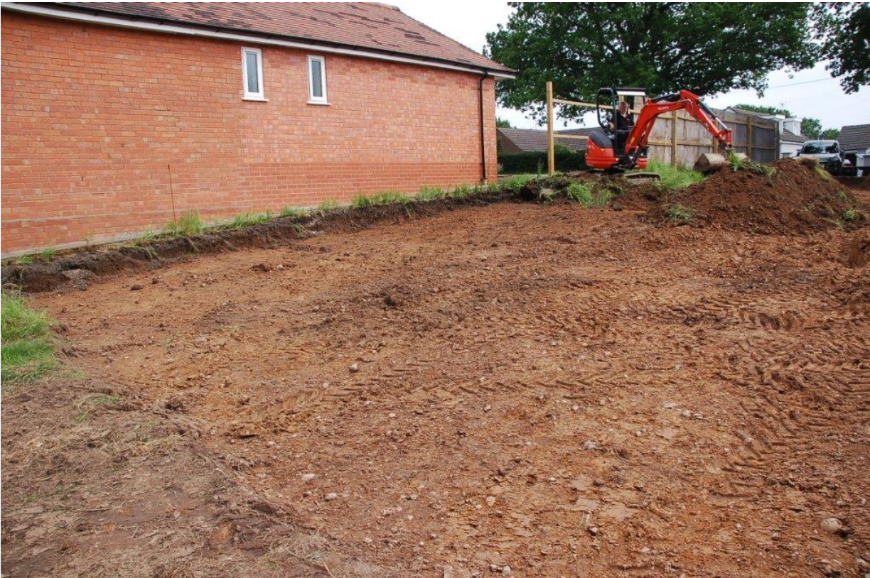
Plate 3: General site strip facing south-east, no scales
