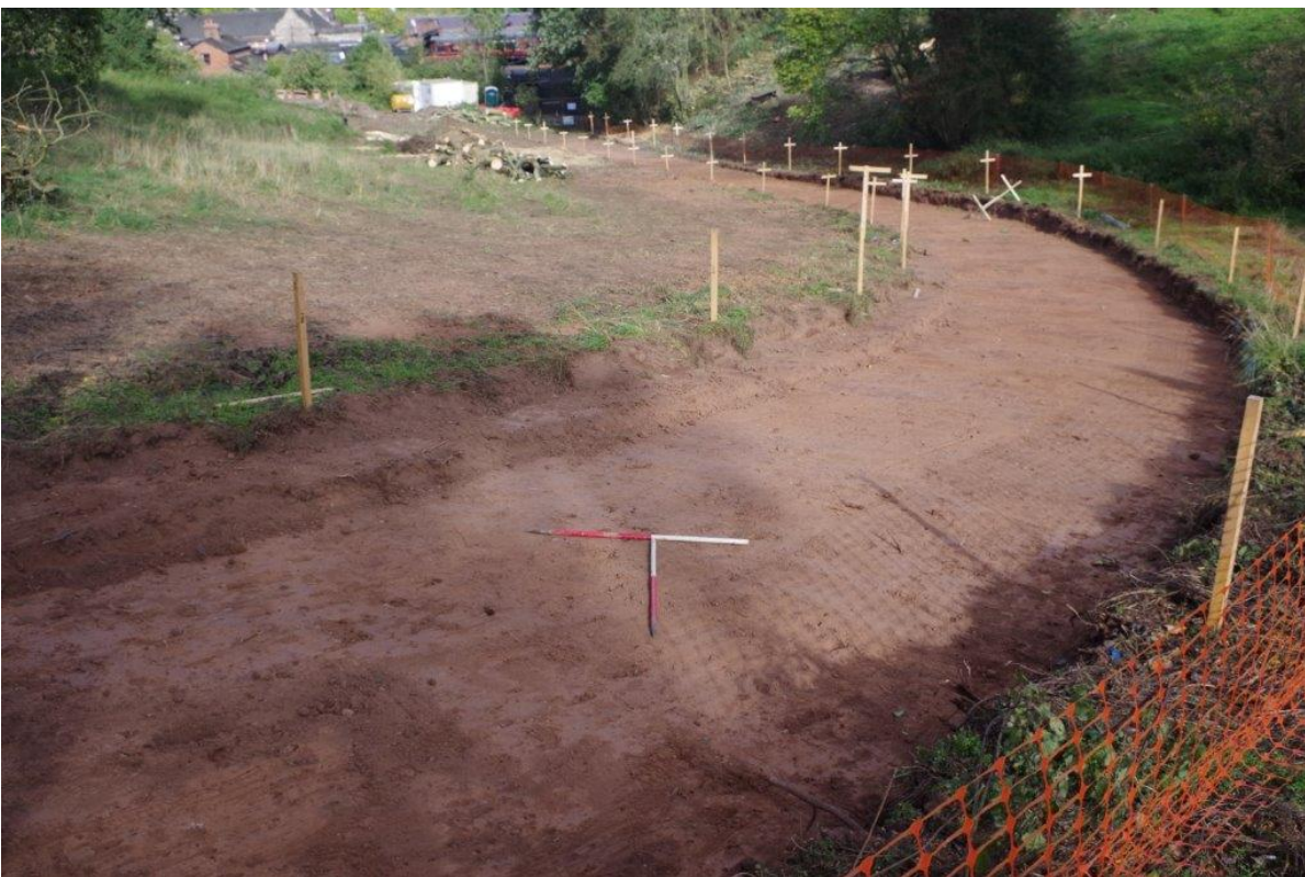
Plate 2 The access road stripped, view south, 2x 1m scales
