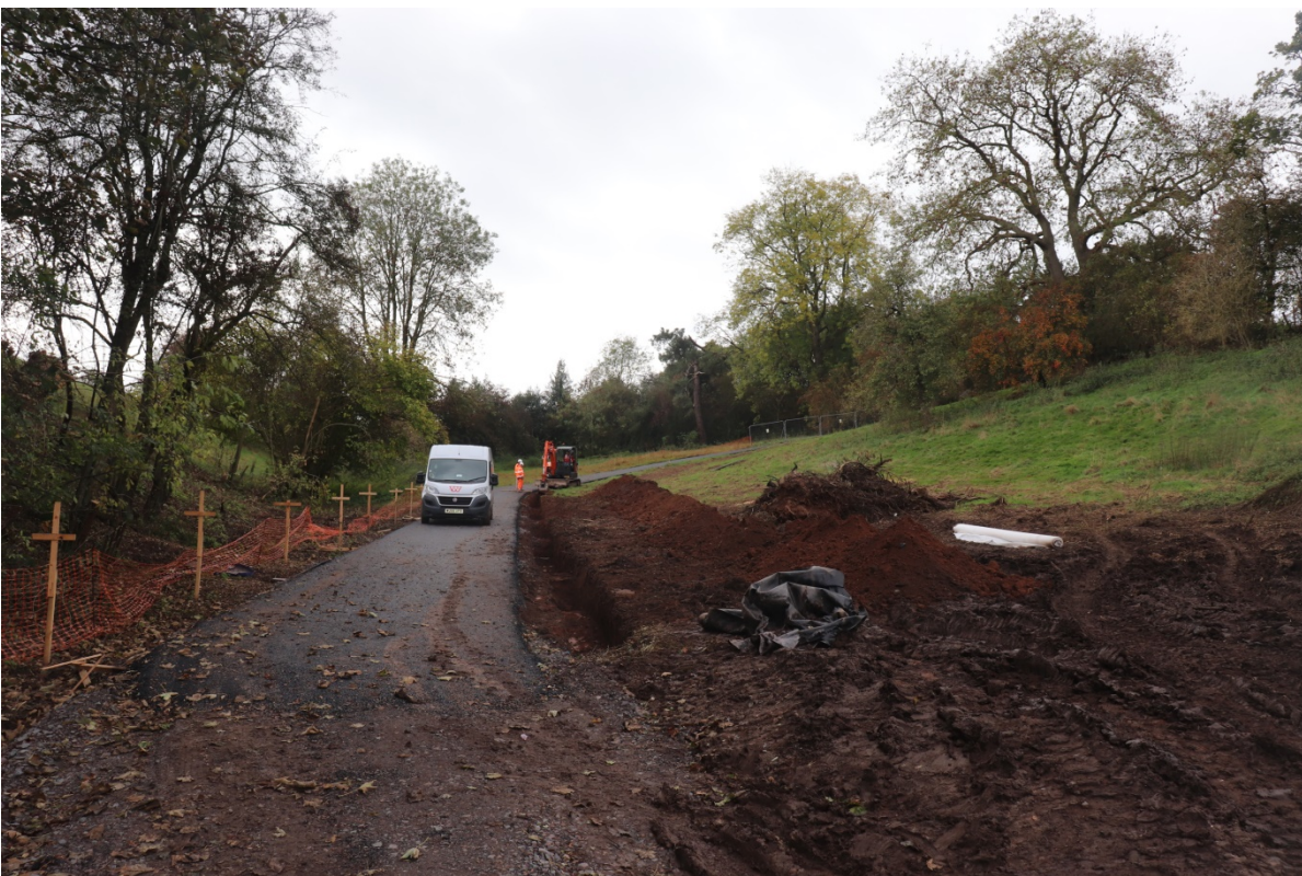
Plate 4 The drainage trench during excavation, view north-west, no scales
