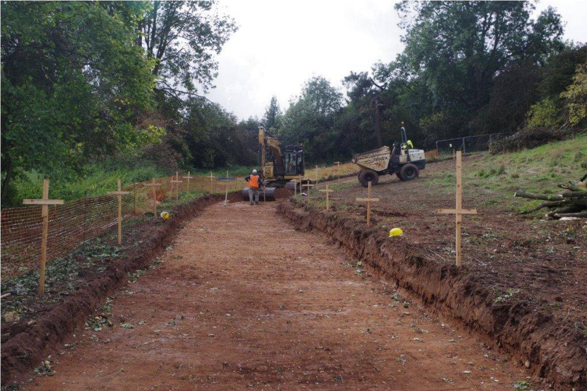
Plate 1 The access road under excavation, view north-west, no scales
