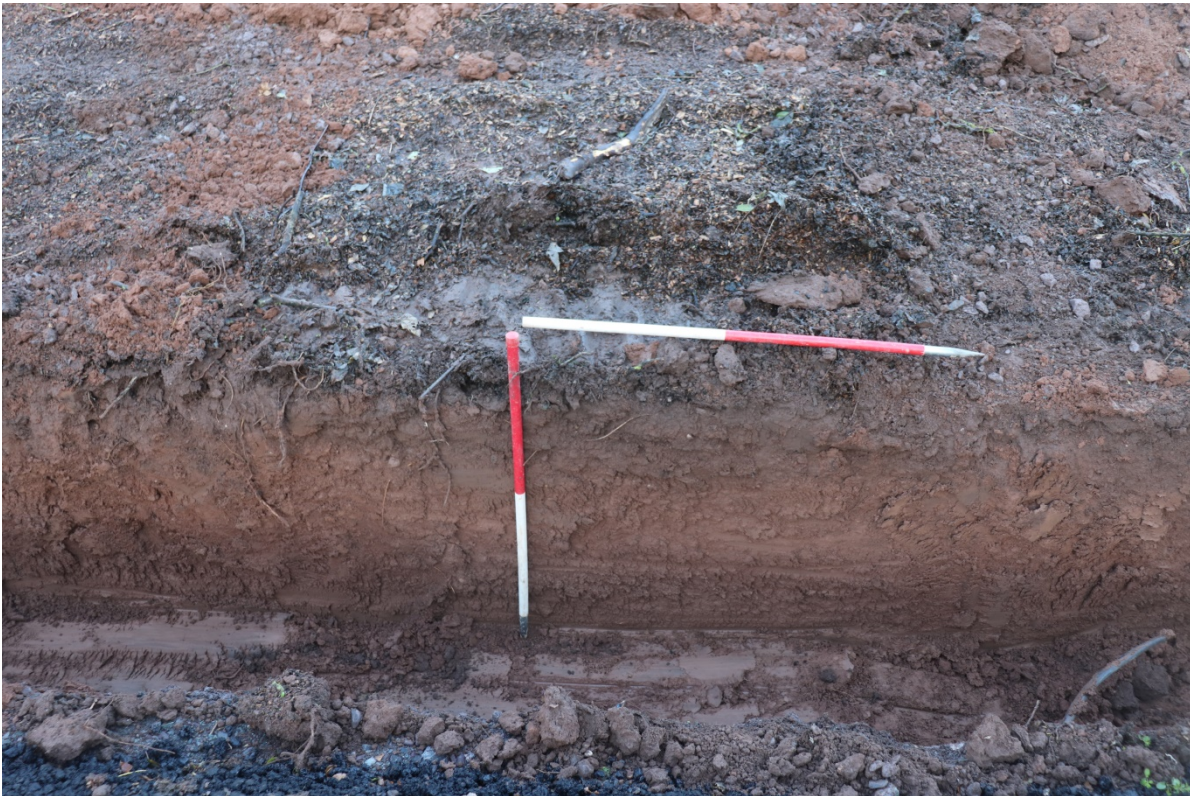
Plate 7 Sample section of drainage trench in the south end of the site, view east, 2x 1m scales
