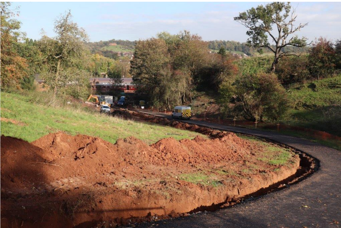
Plate 6 View south of the completed drainage trench, no scales
