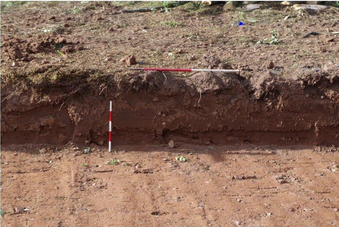
Plate 3 Sample section of access road showing topsoil and subsoil observed in strip, 0.5m and 1m scales
