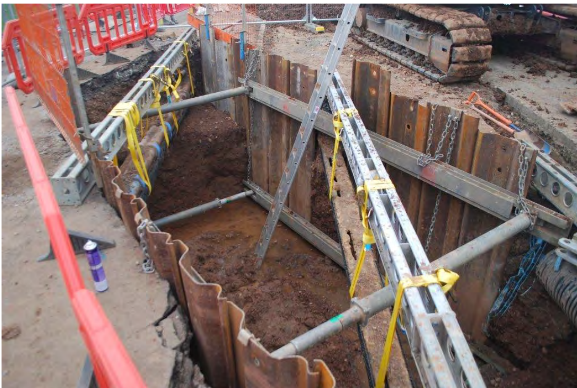
Plate 2: General shot showing working conditions
