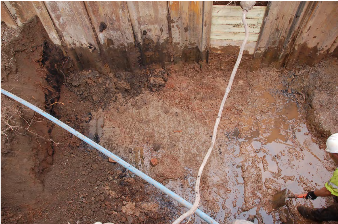
Plate 5: Cut of ditch [479] as revealed in plan at culvert base
