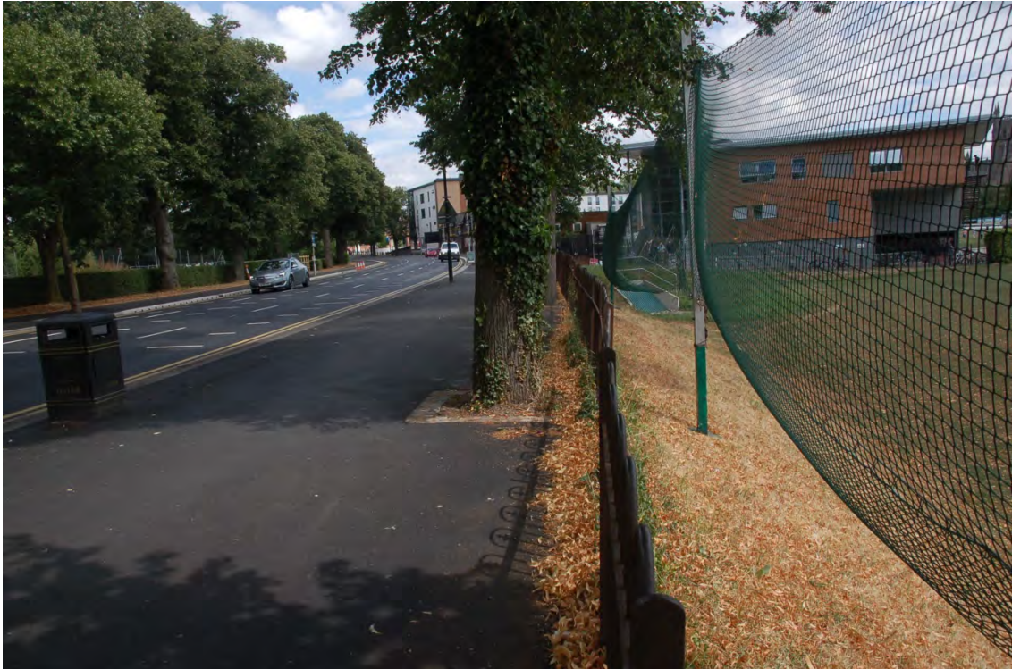
Plate 1: Shot showing the drop from made ground under New Road to adjacent playing fields (facing east)
