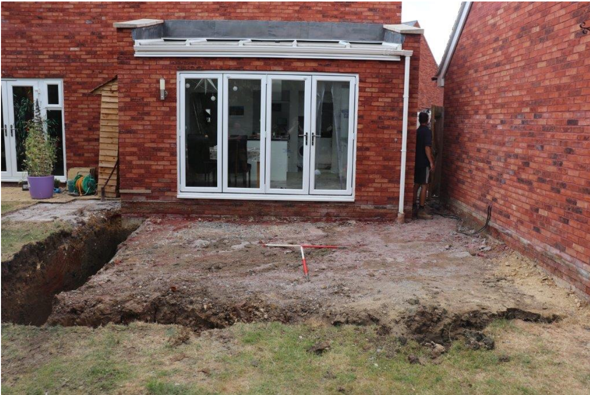
Plate 3 Ground reduction and foundation trenches, view north-west, 2x 1m scales
