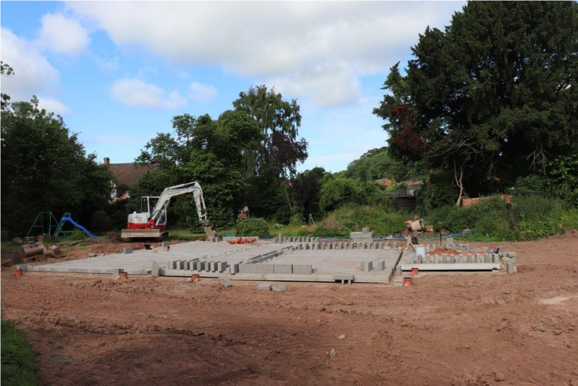
Plate 1 Modern house footings, looking south-west towards areas archaeologically monitored
