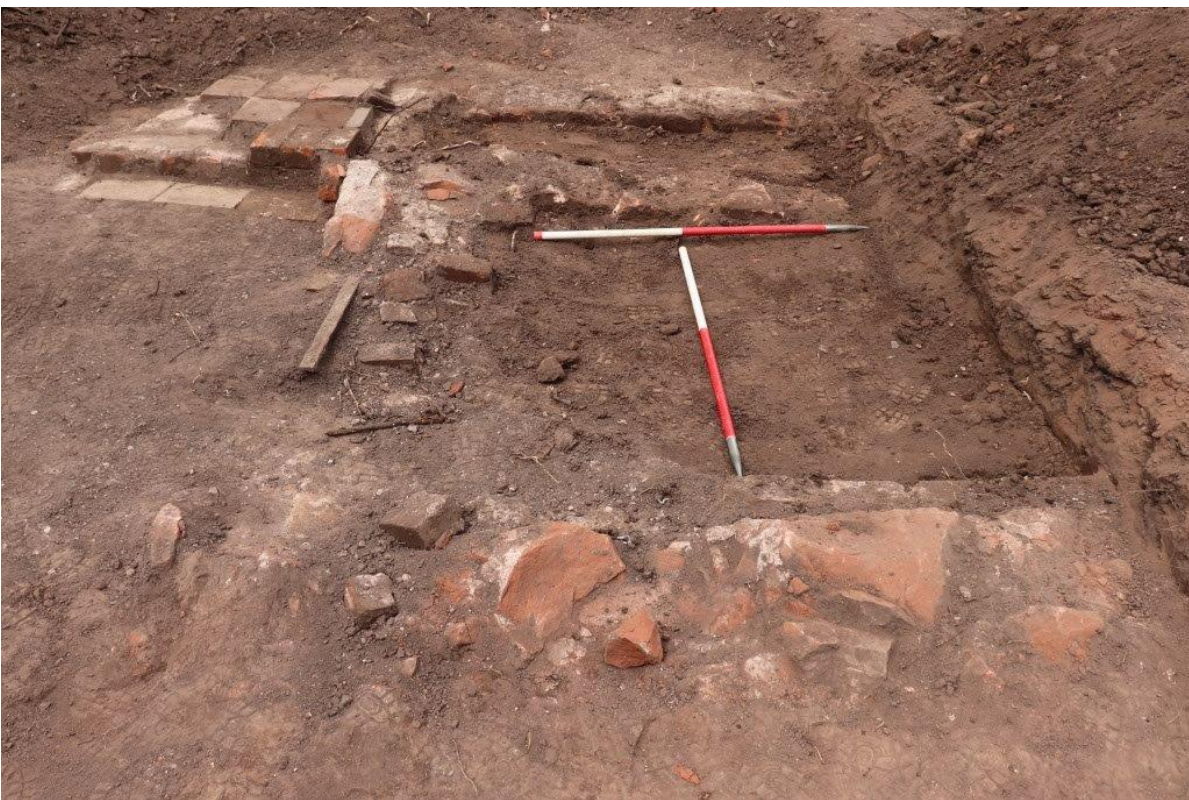
Plate 10 Building foundation structure [207] and [209] after excavation, view north, 2x 1m scales
