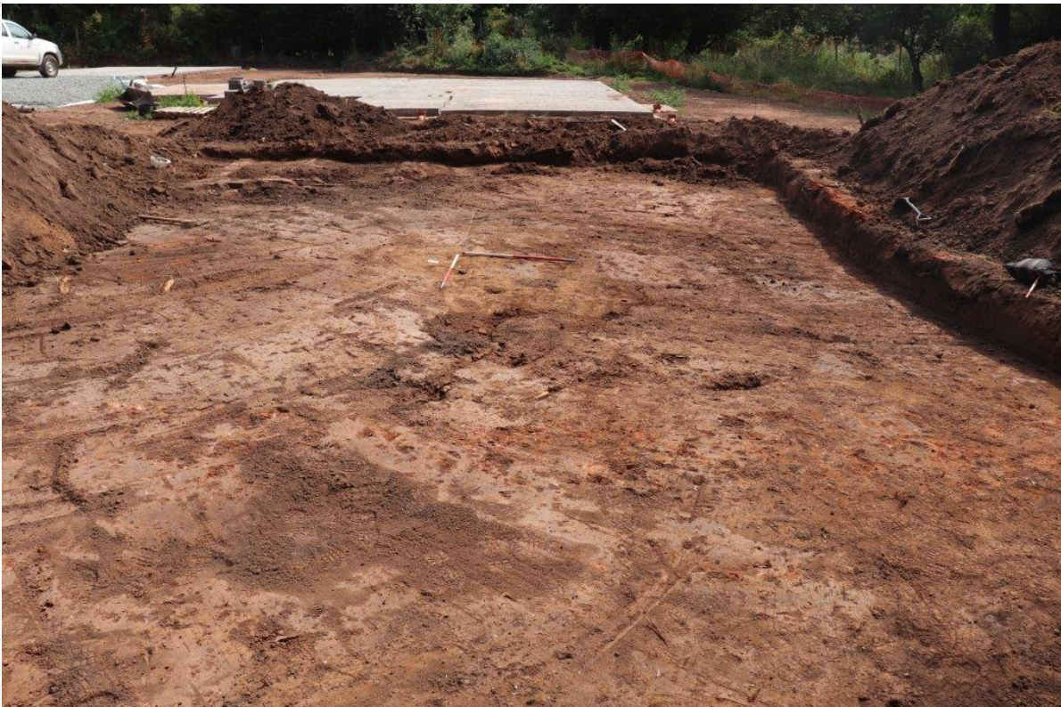
Plate 6 Trench 2 after stripping to natural, view east, 2x 1m scales
