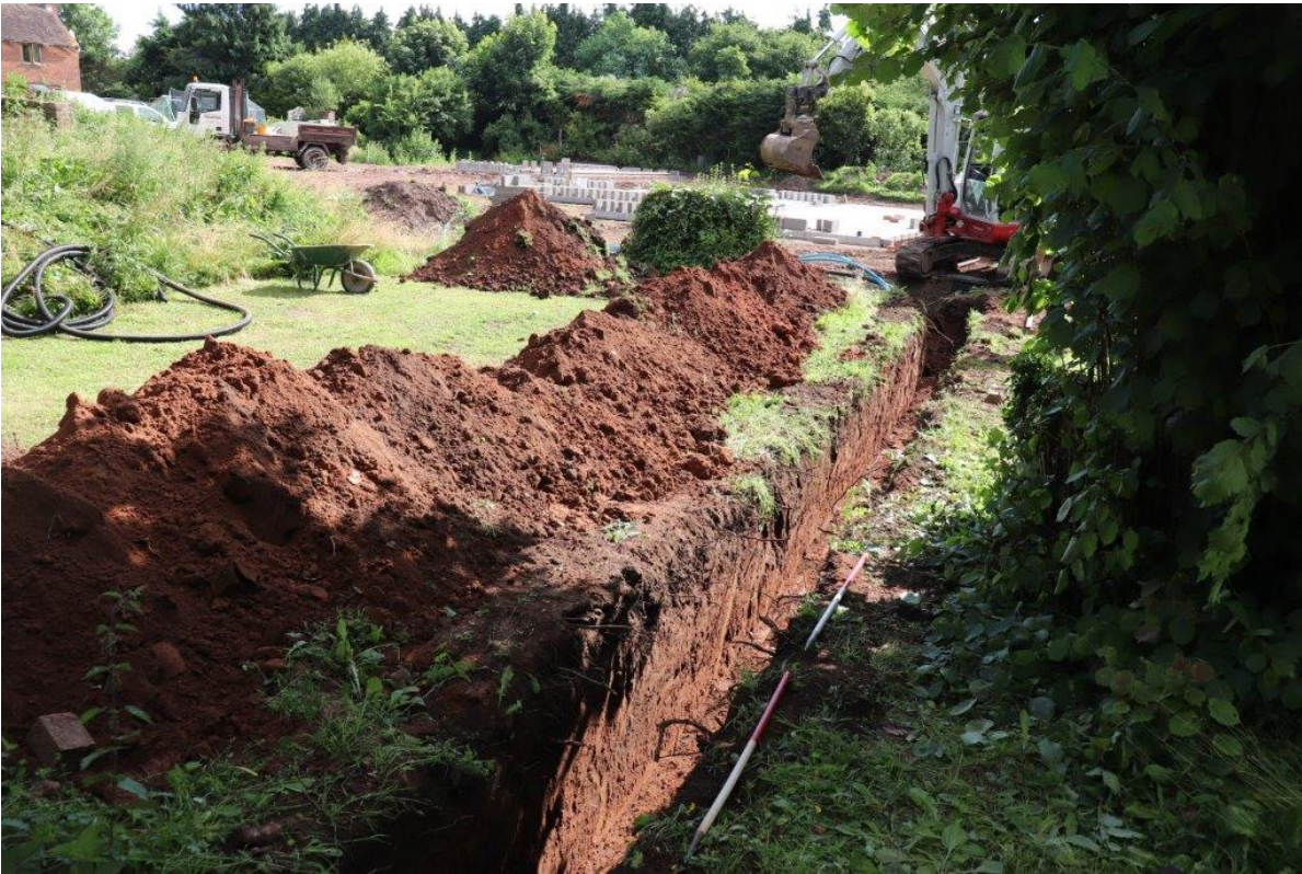
Plate 3 Drainage Trench (Trench 1) looking north-east, 2x 1m scales
