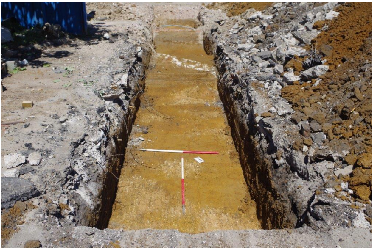
Plate 2: Trench 2, facing north-west (scales 1m)
