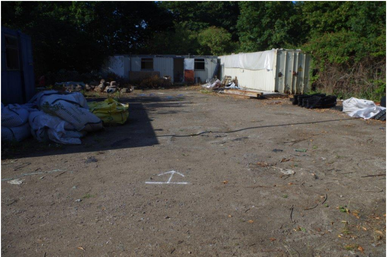
Plate 1: General site conditions before excavation of Trench 3, facing south-west
