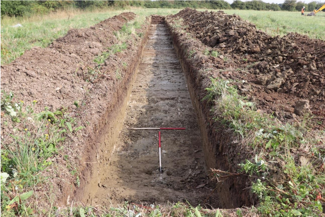
Plate 3 Trench 5, facing north
