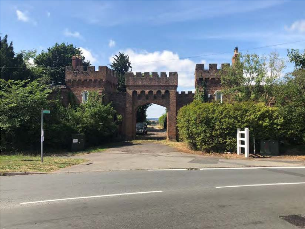
Plate 5: The Grade II listed North Lodges and Gateway of Lea Castle
