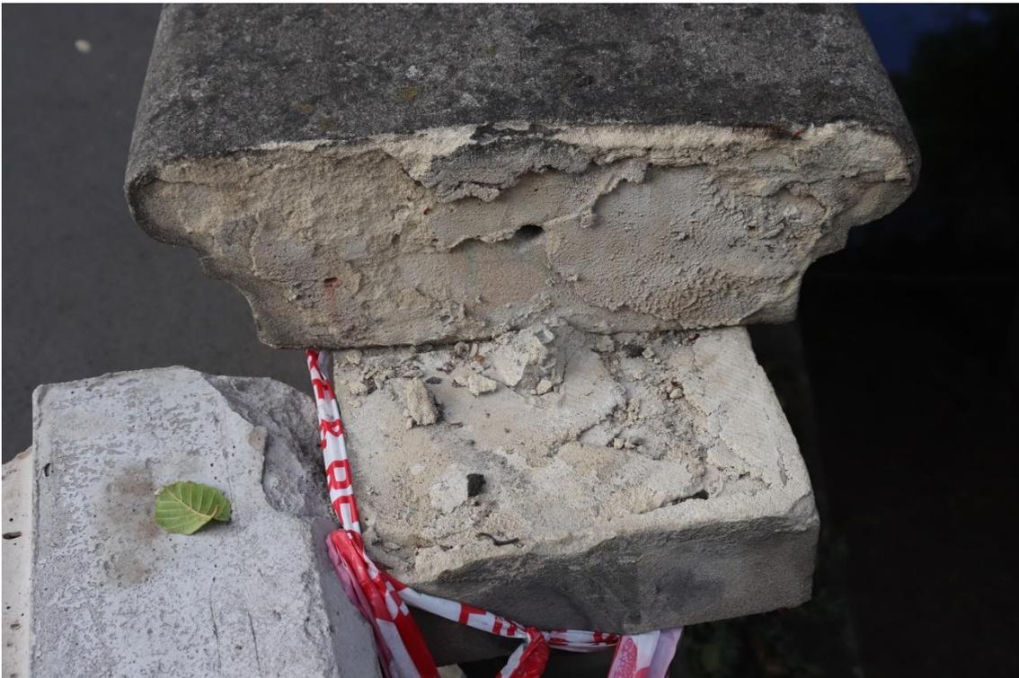
*Plate 15 Damaged area of the north parapet, rail detail with central drill hole for a stainless steel dowel and acrylic resin bonding, looking south-west*
