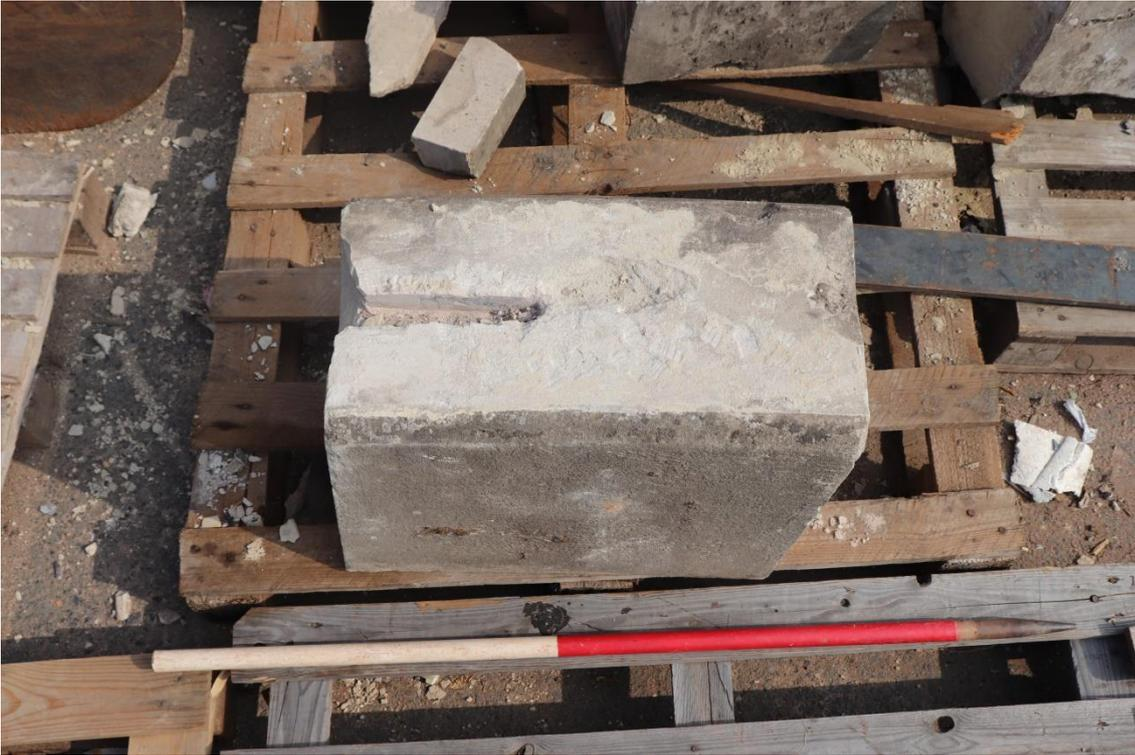
*Plate 18 Mortise for a slate dowel as specified in the drawings reapiers of 1993*
