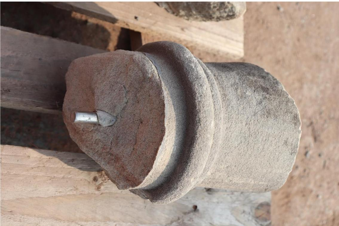
*Plate 17 Damaged baluster stainless steel dowel and acrylic resin bonding*
