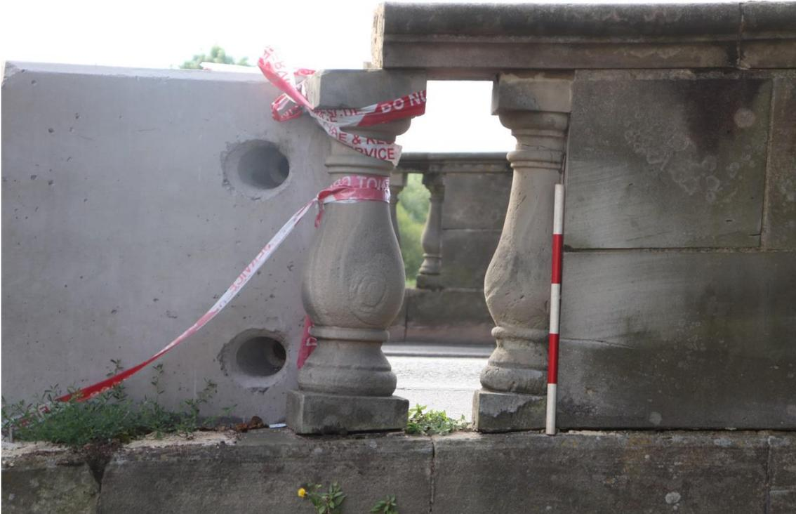
*Plate 14 Damaged area of the north parapet, baluster detail, looking east*
