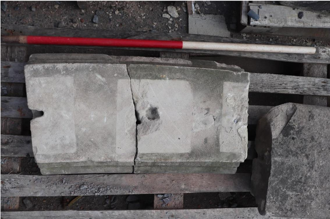
*Plate 20 Rail stone underside with evidence of circular saw conversion with drill holes for a stainless steel dowel and acrylic resin bonding*
