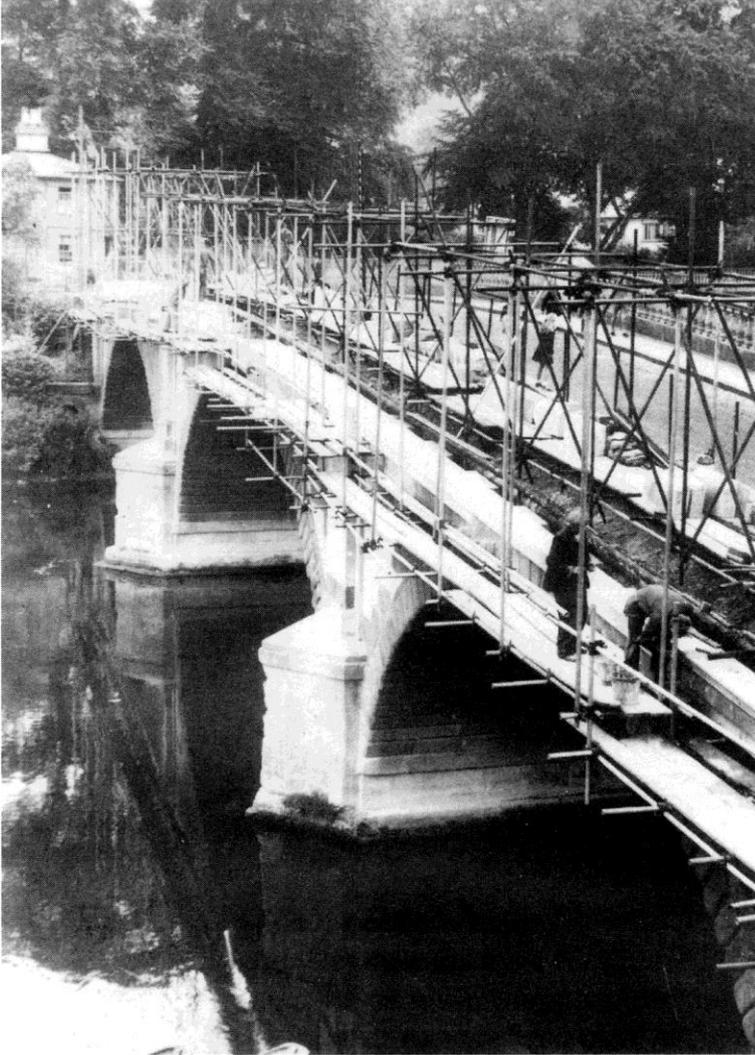
*Plate 7 Entire removal and possible complete replacement of the north parapet of the bridge as photographed in 1950. New stone is clearly being used for the reinstatement (Bewdley Historical Research Group 2005)*
