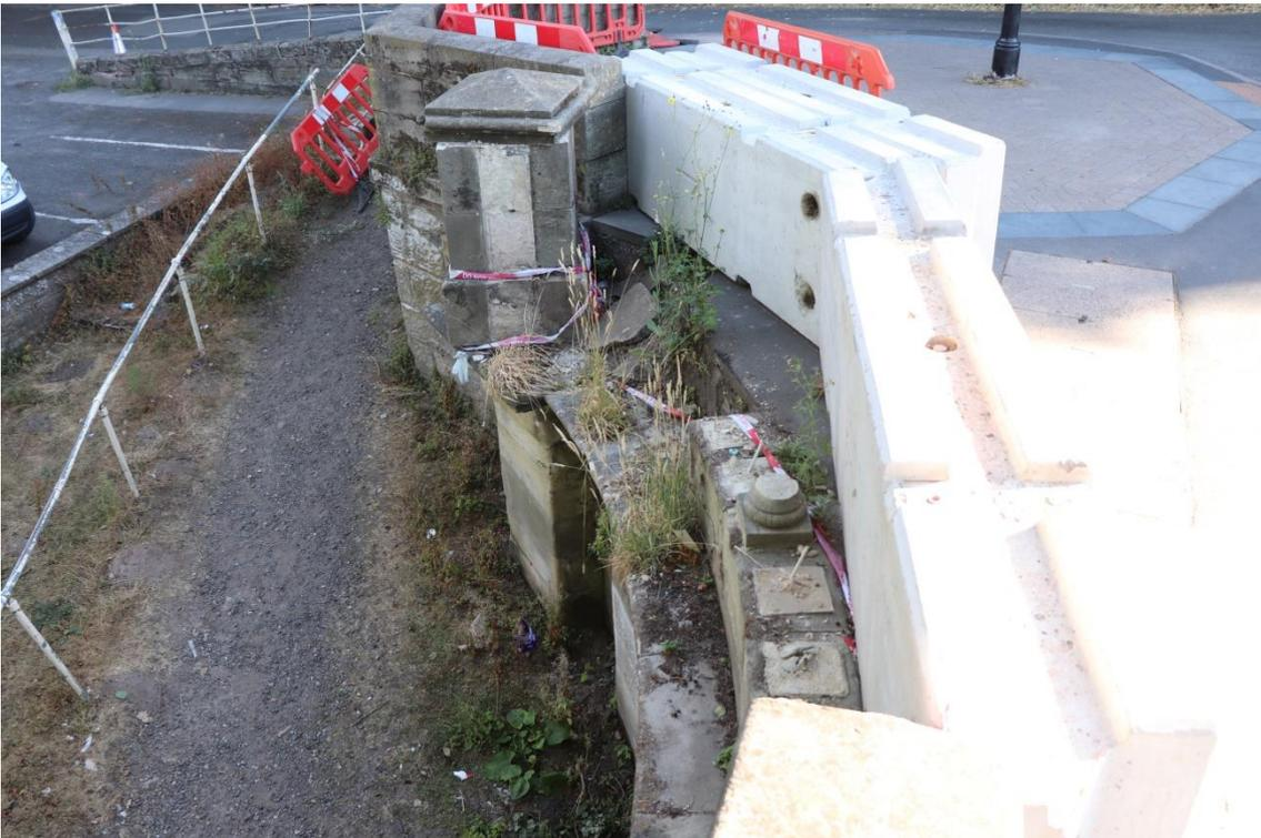
*Plate 13 Damaged area of the north parapet, looking north*
