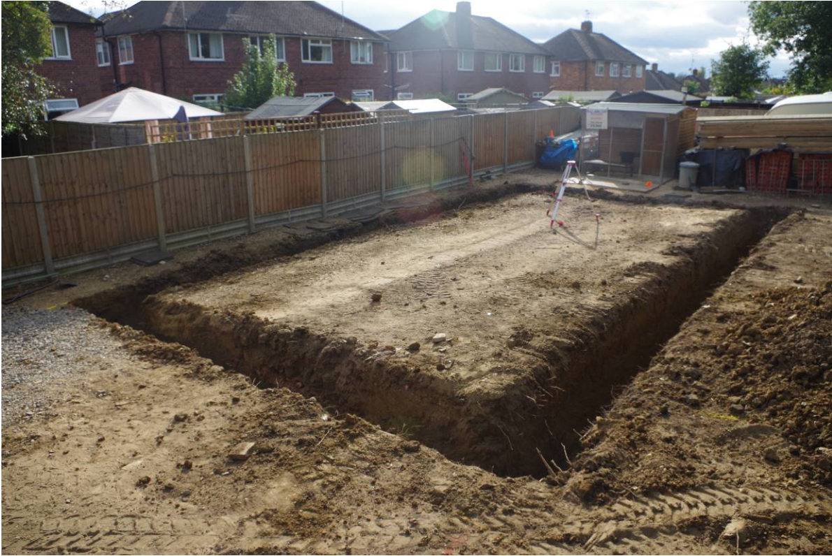
Plate 1: The excavated footing trench; view west; no scales
