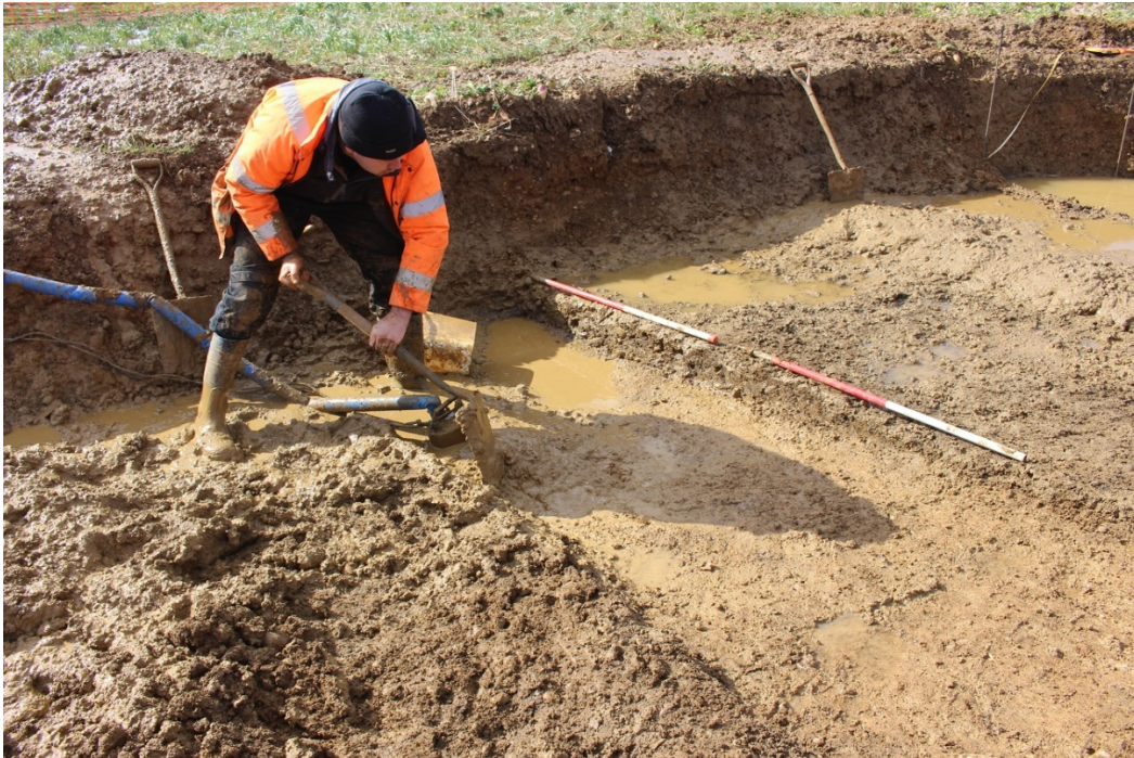
Plate 4: Working shot of slot in layer (3031), oblique view facing west (1m scales)
