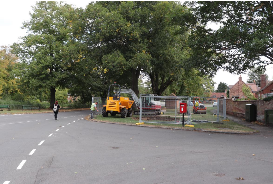
Plate 1 The site, facing east
