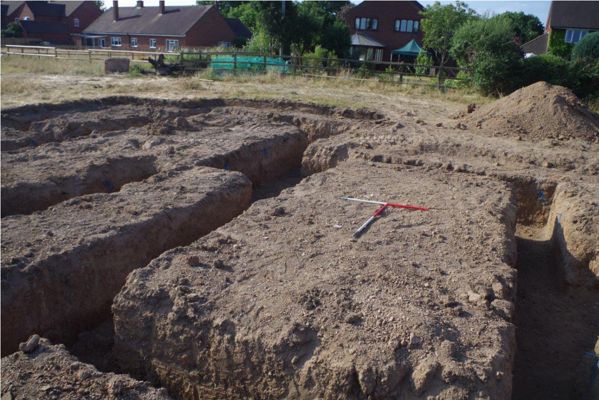
Plate 5 Trench 2, looking south-east (1m scales)
