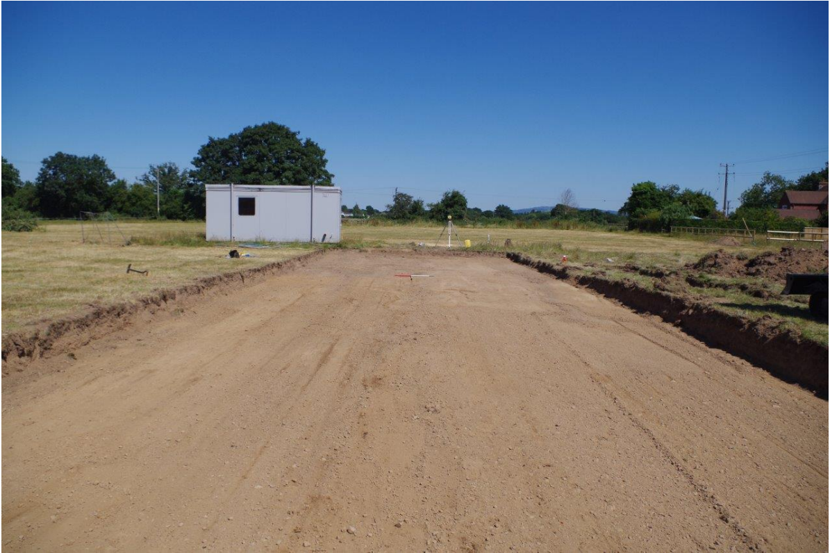
Plate 1 Trench 1, looking east (1m scales)
