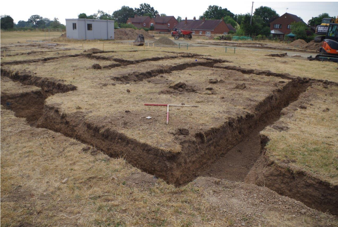
Plate 6 Trench 5, looking south-east (1m scales)
