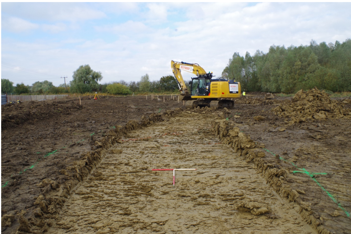
Plate 2: Stripping the site; view north-east; 2x 1m scales
