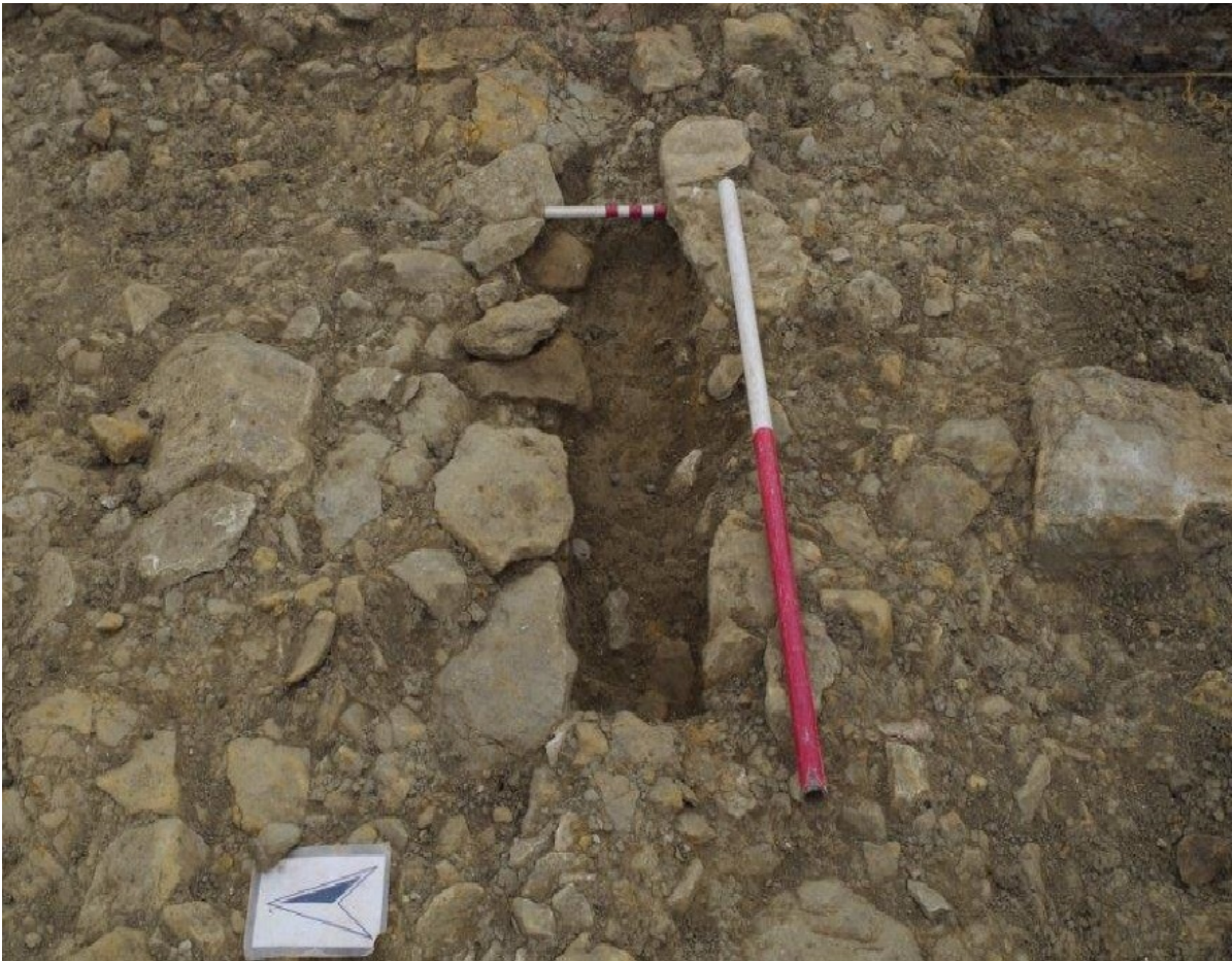
Plate 16 CG15 Culvert 2013, looking east (1m and 0.1m scales)
