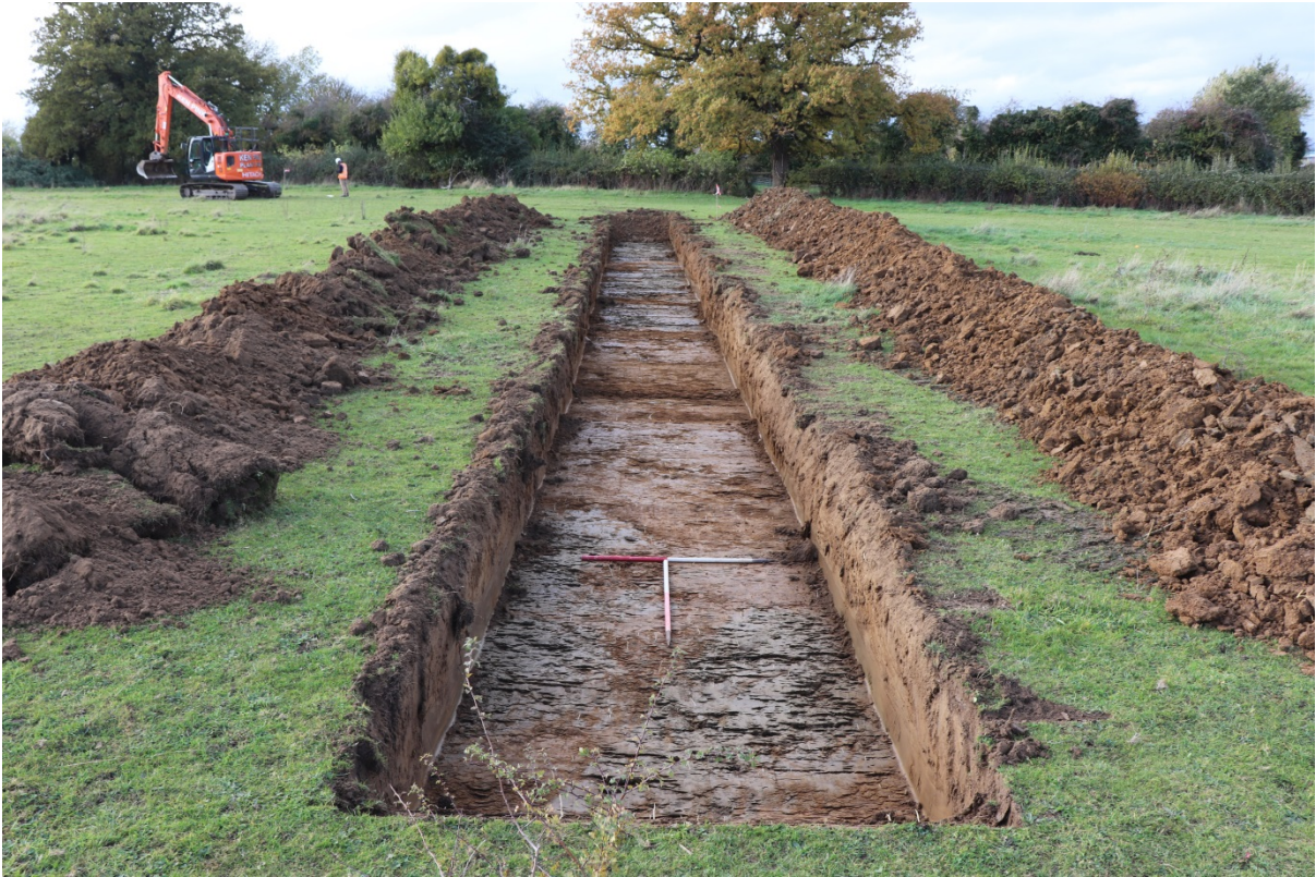
Plate 1: Trench 10, reddish brown silty sand overlying natural blue grey clay, view west, 2x 1m scales
