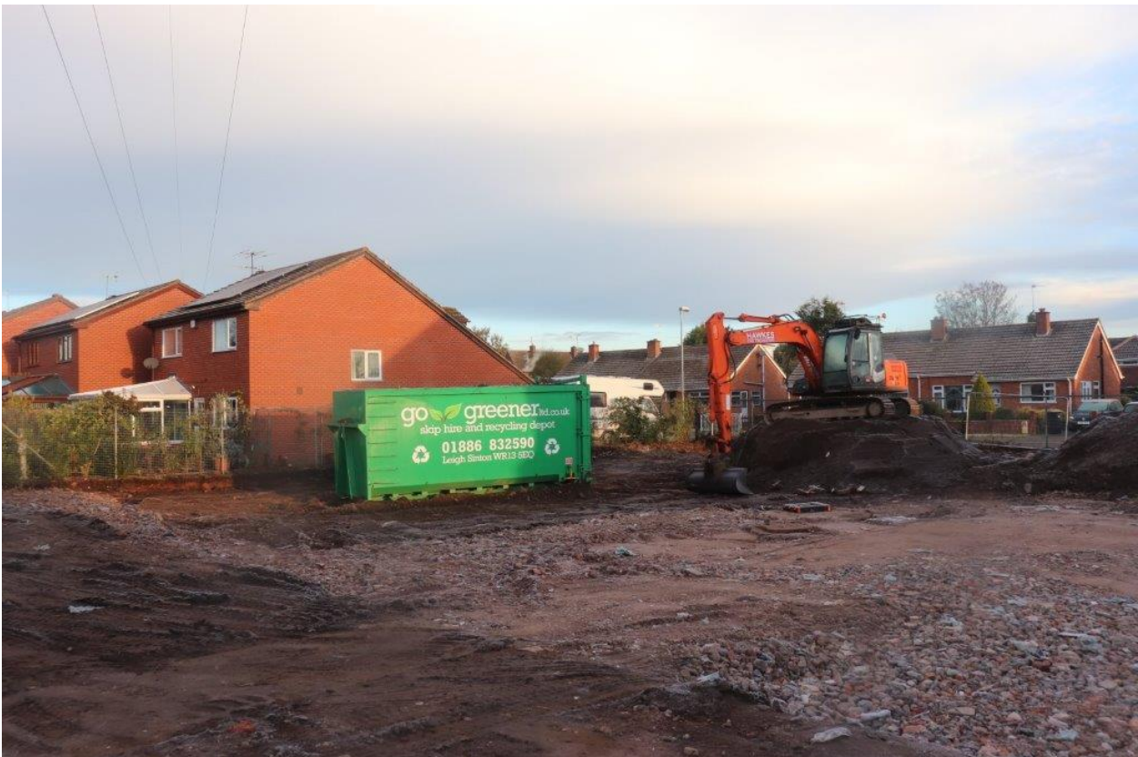
Plate 6 The site with piling mat following excavation works looking north.
