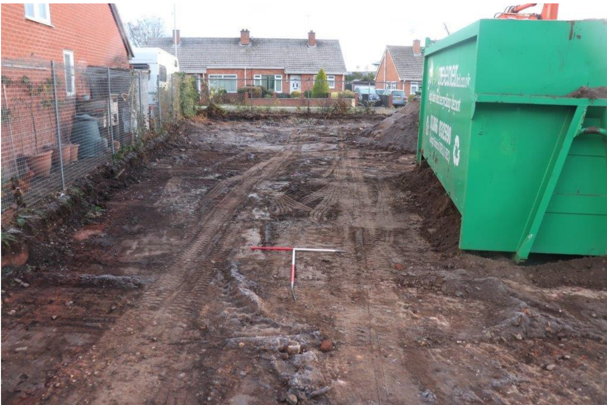
Plate 4 Northwest side of site stripped looking Northeast. 2x1m scales.
