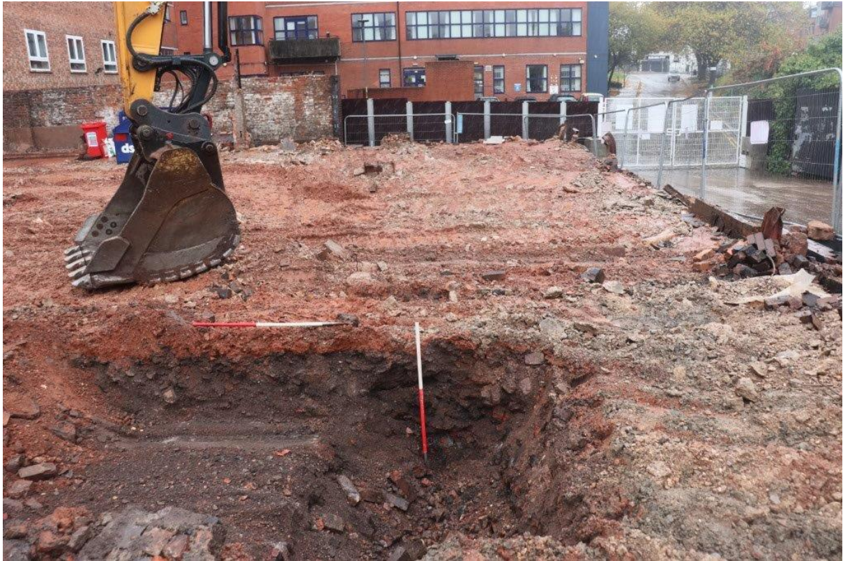
Plate 5: Trial Hole 3 showing concrete footing of existing warehouse. Looking west
