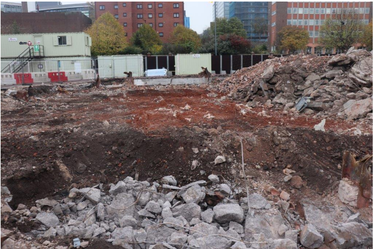
Plate 2: The eastern end of the demolished warehouse, looking south
