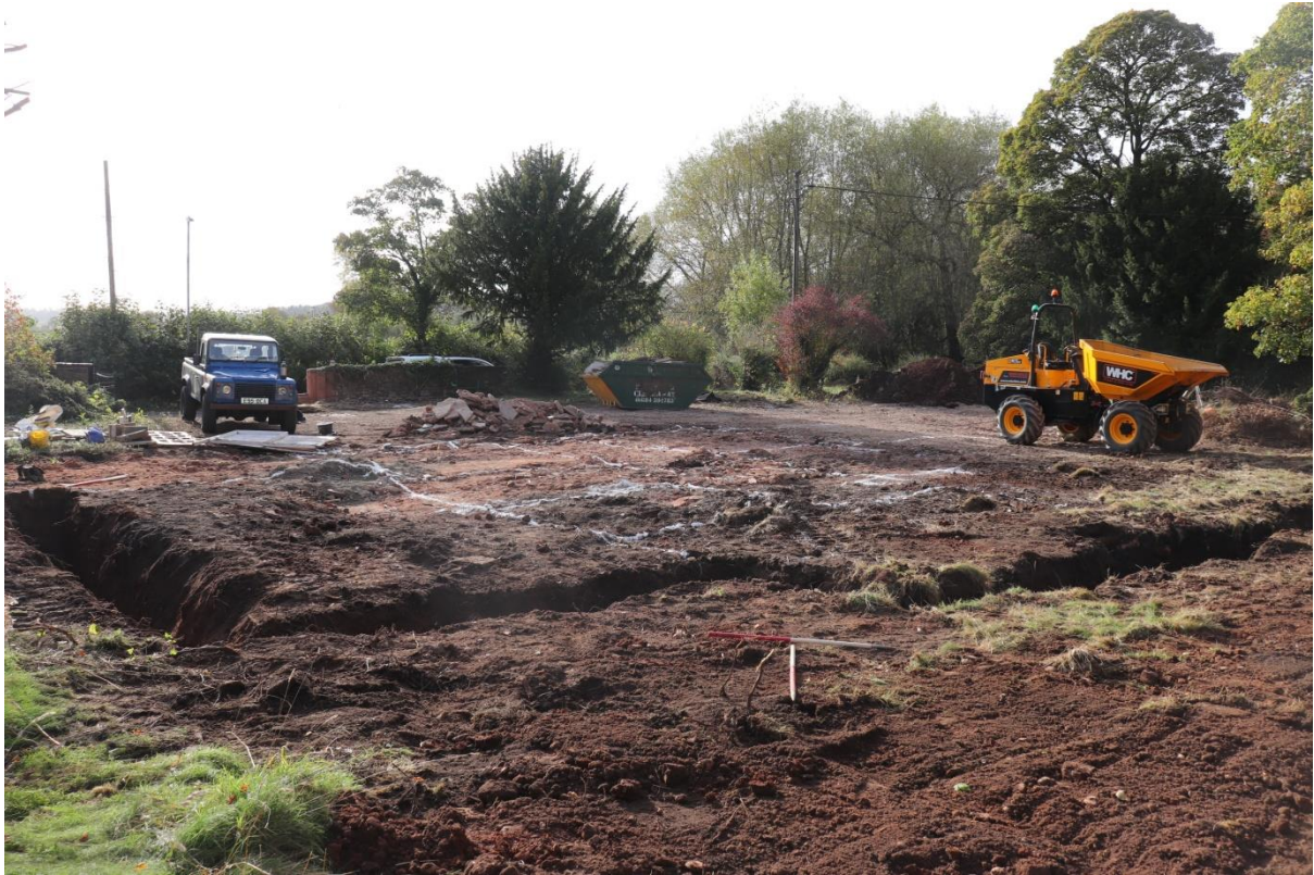
Plate 3: General shot of groundworks looking southwest with 2x1m scales
