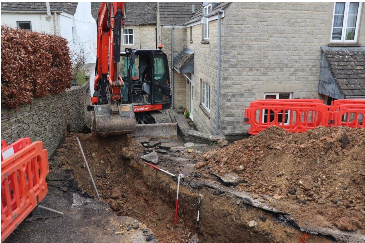
Plate 16: Service trench in progress looking south, with 2x1m scales
