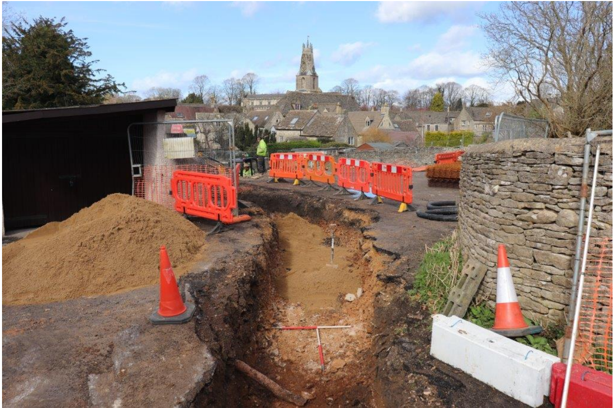
Plate 15: Service trench (Trench 3) looking northwest, with 2 x1m scales
