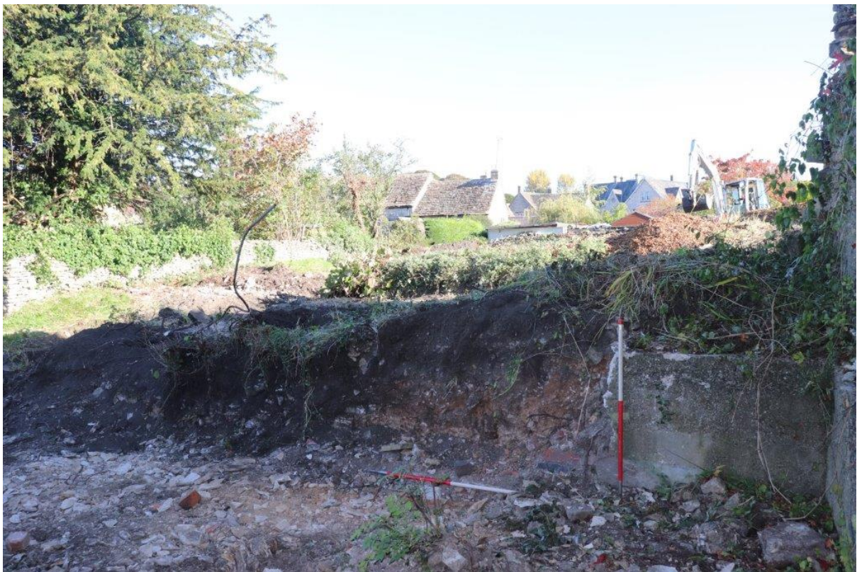
Plate 2: Example of made ground bank in the garden, looking northwest with 2 x 1m scales
