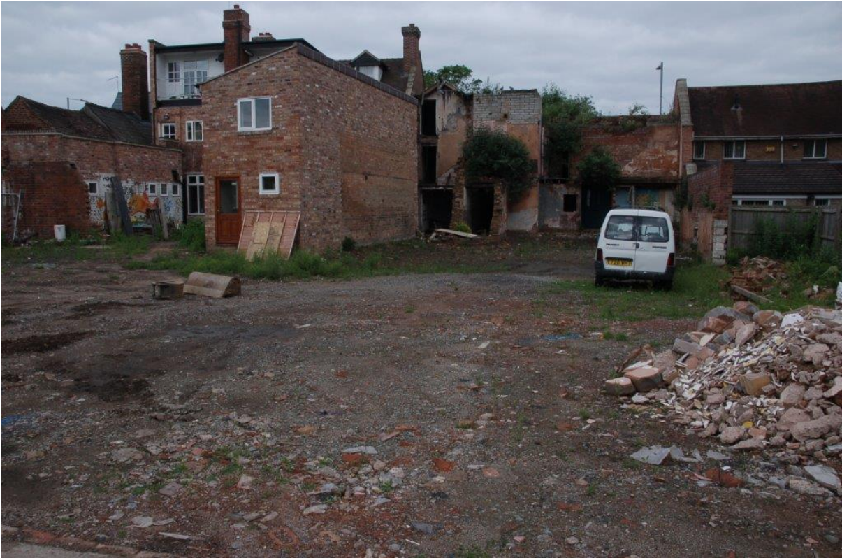
Plate 1 General shot of site, looking south-west, prior to site investigations
