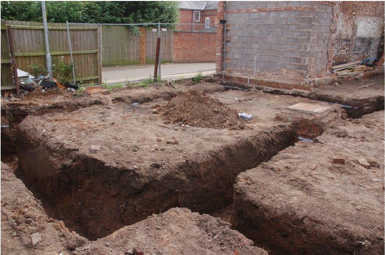
Plate 11 Trench 4 general shot, looking south-west
