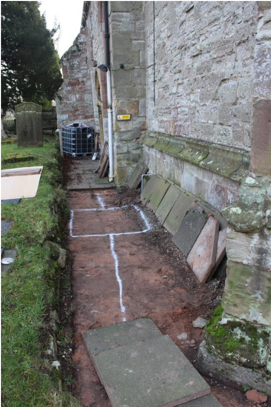
Plate 1: Pre-excavation view of drainage route on north side of church
