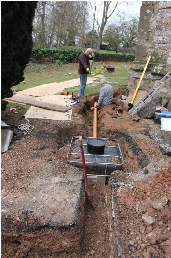
Plate 2: Working shot of drainage route on west side of church
