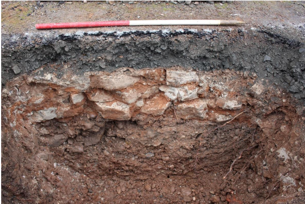
Plate 3: Wall foundation (103) below tarmac (102) west of church tower, facing east (scale 1m)
