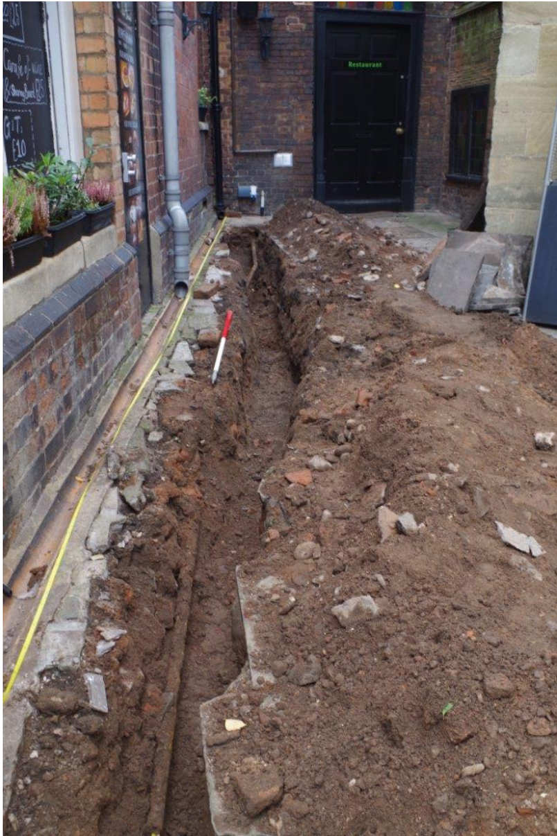
Plate 5: View north of trench, in courtyard; 1m scale
