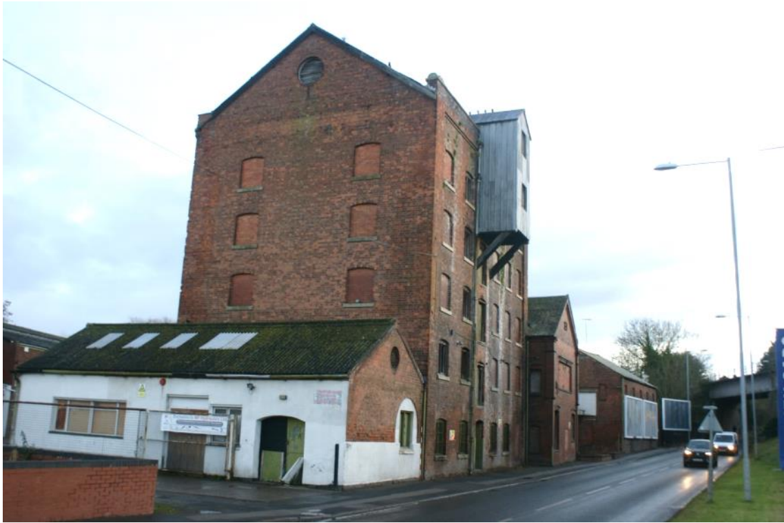
Plate 18 Building B, looking north-east
