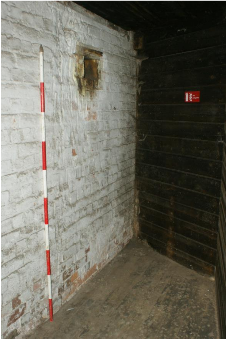
Plate 34 Building B third floor possible drive shaft hole, looking west
