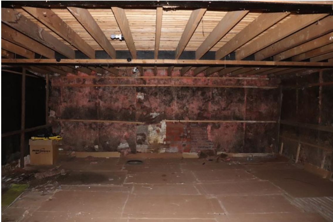
Plate 54 Building C ground floor, looking north
