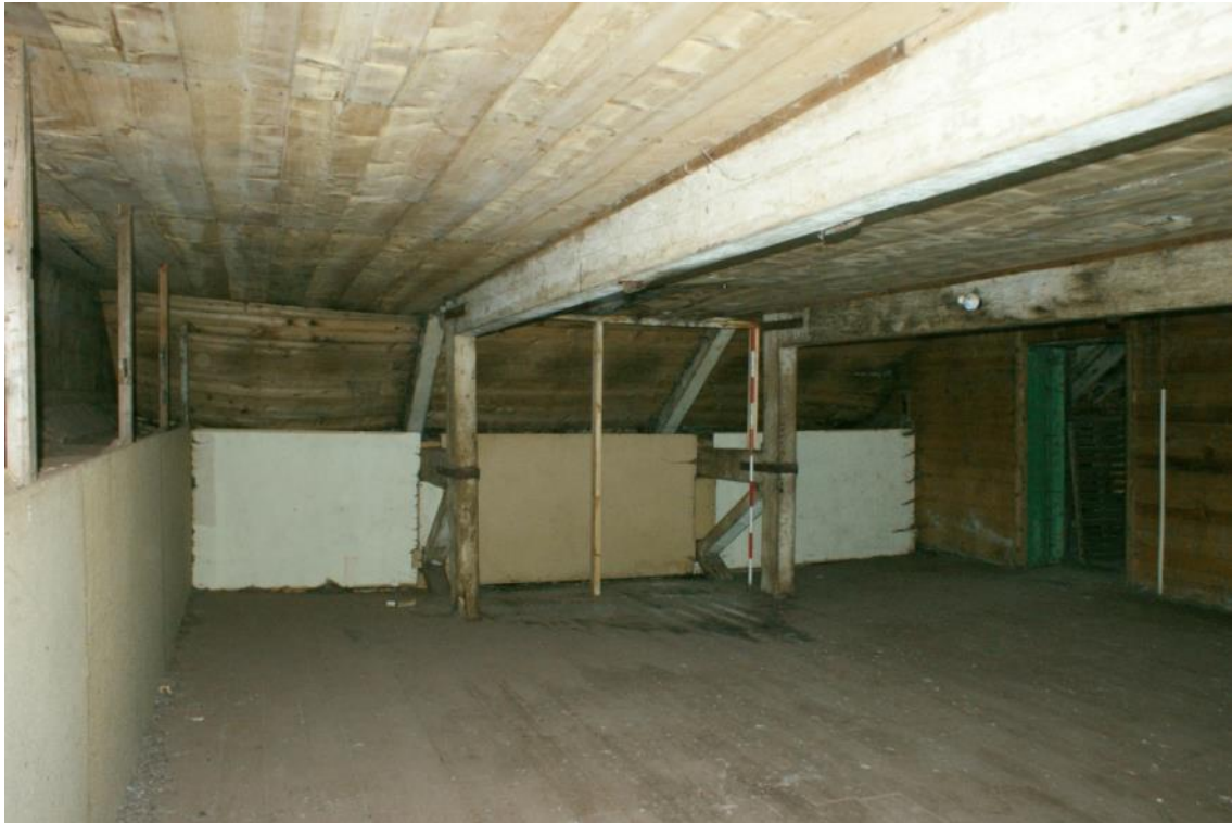
Plate 24 Building B fifth floor, looking south
