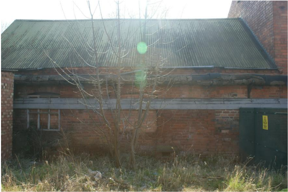
Plate 50 Building I, looking south
