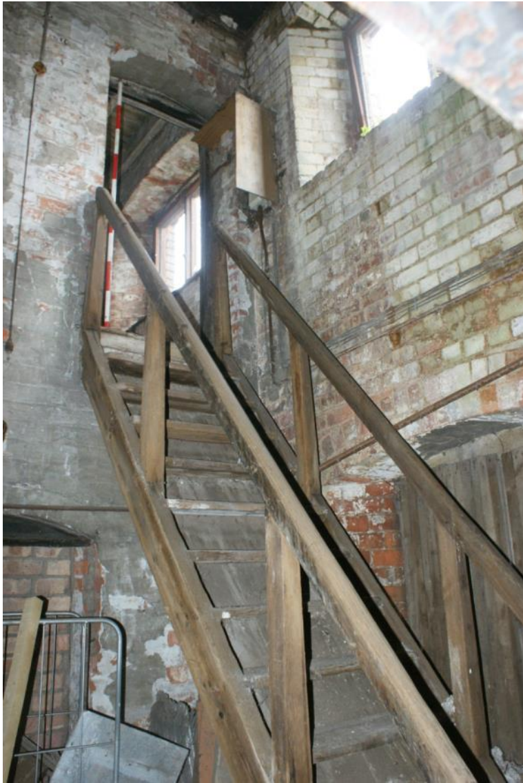
Plate 30 Building B ground floor, looking south-east
