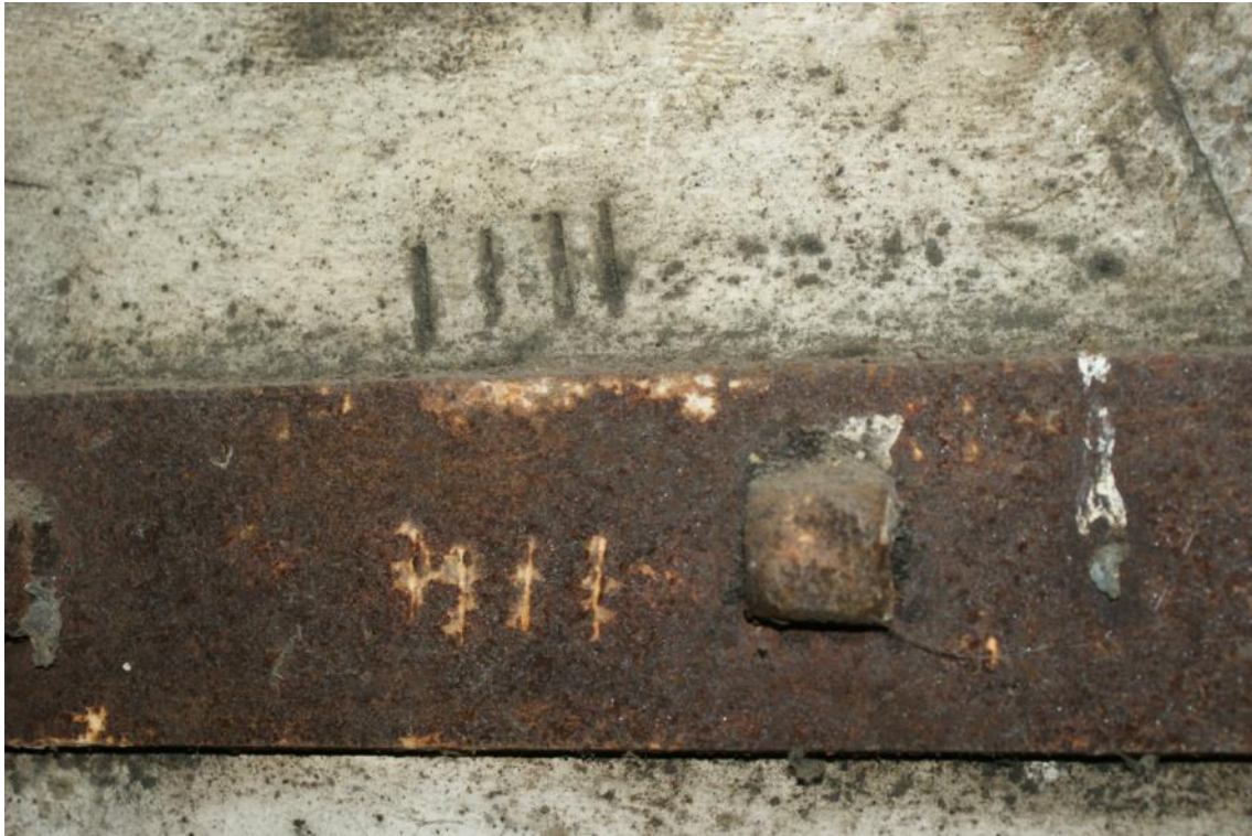
Plate 22 Building B fifth floor roof truss fastening and marks, looking east
