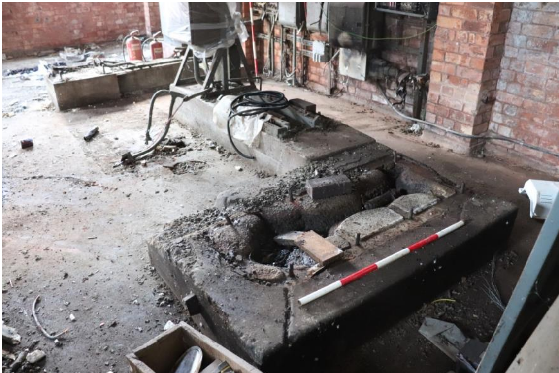
Plate 57 Building F interior machine bases, looking north-east
