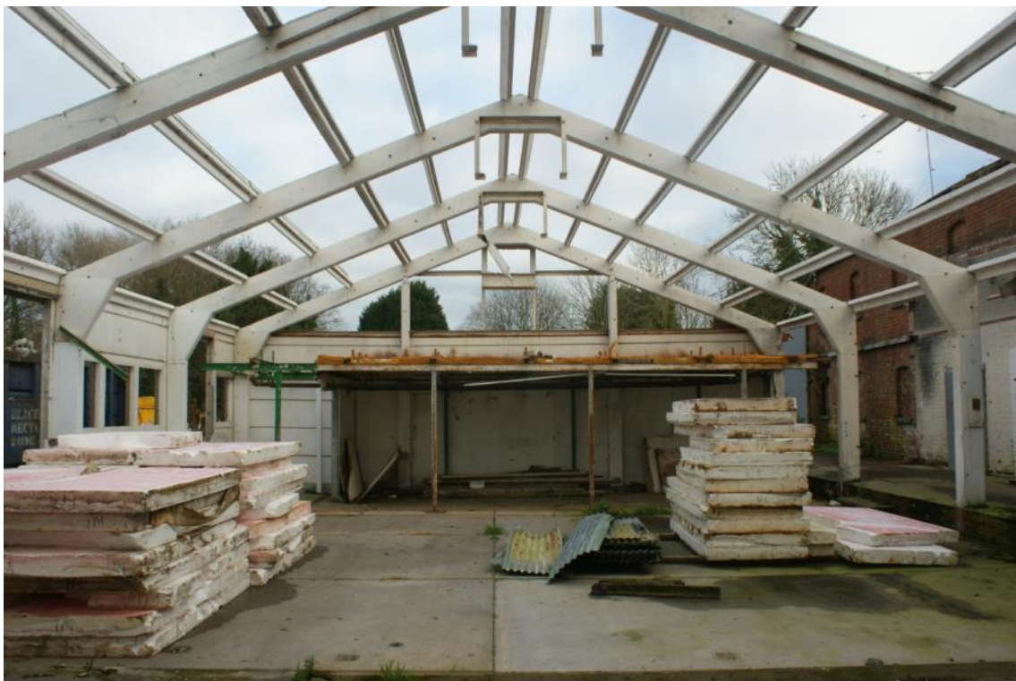
Plate 74 Building G, looking east
