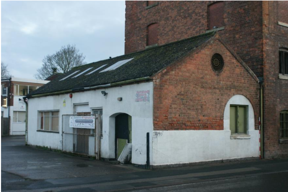
Plate 44 Building A, looking north-east
