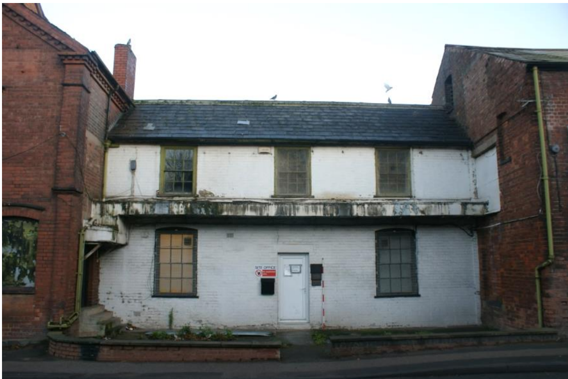
Plate 9 Building D, looking north
