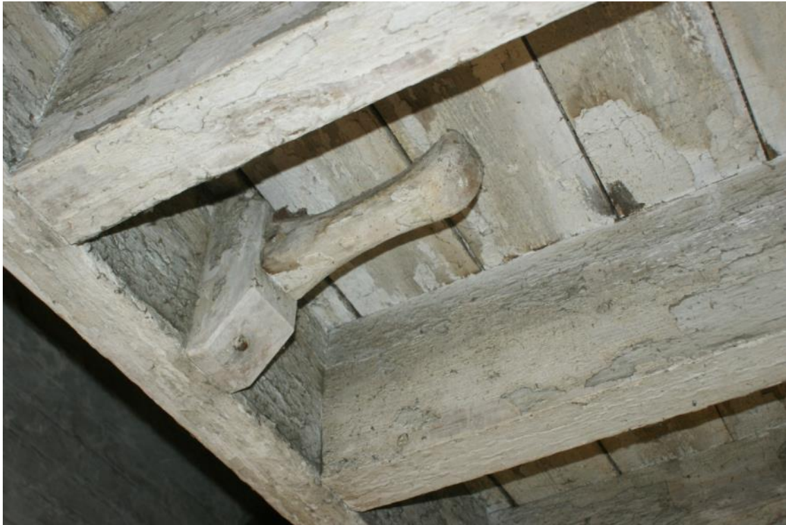
Plate 37 Building B first floor wooden hook, looking north-west
