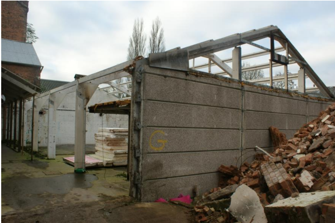
Plate 73 Building G, looking north-west
