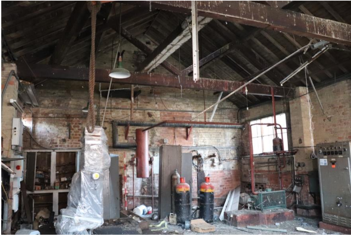
Plate 6 Phase 1 structure from within building F, looking south
