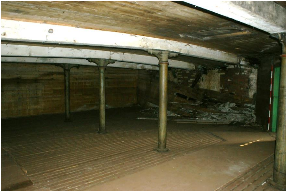
Plate 25 Building B fourth floor, looking south-east
