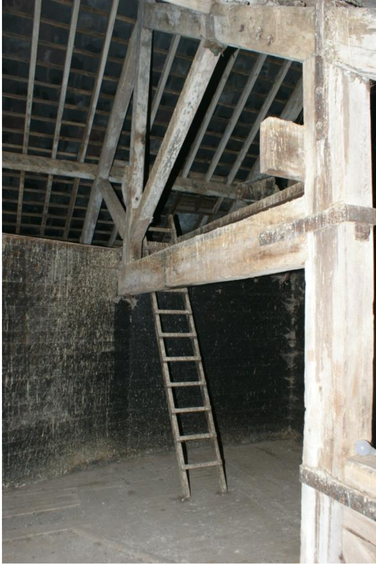
Plate 21 Building B fifth floor roof trusses, looking north
