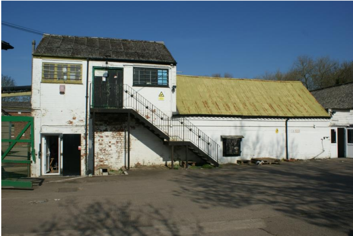
Plate 63 Building I, looking north
