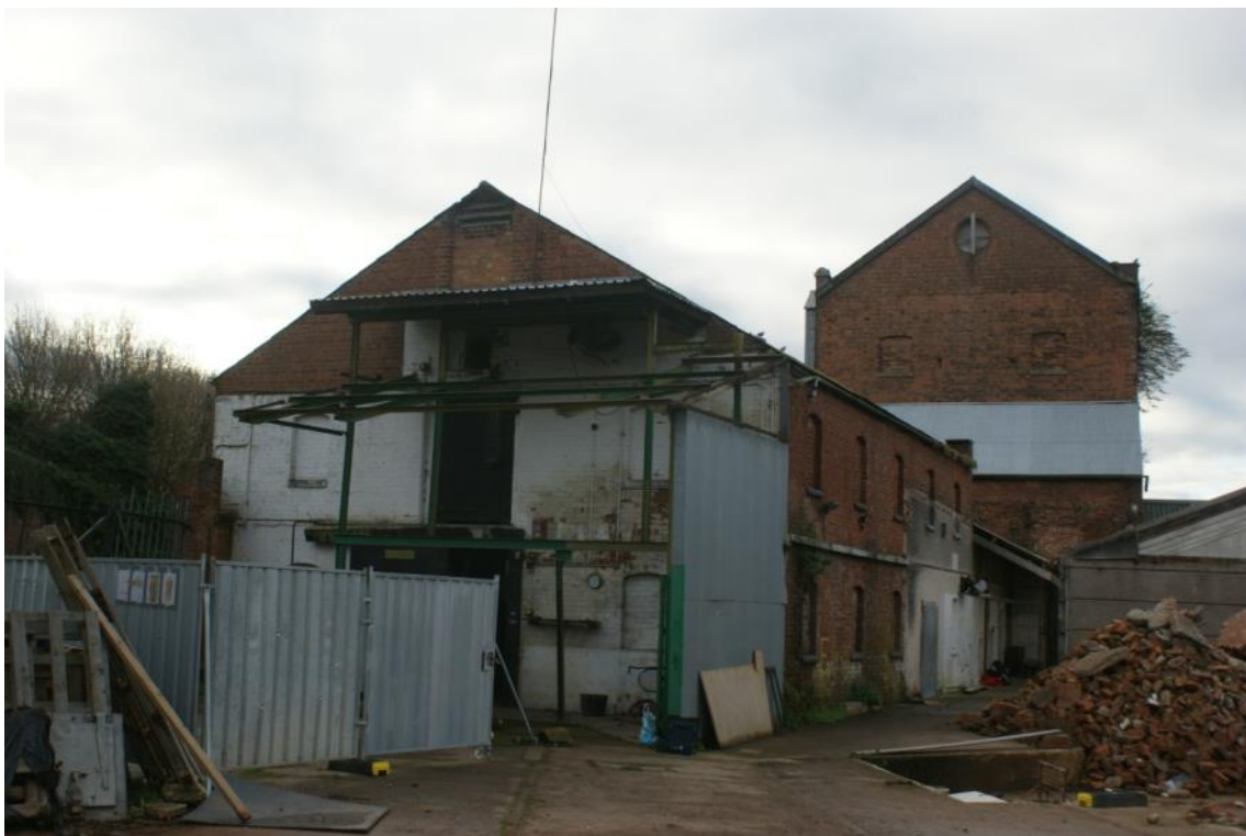
Plate 47 Building E, looking west
