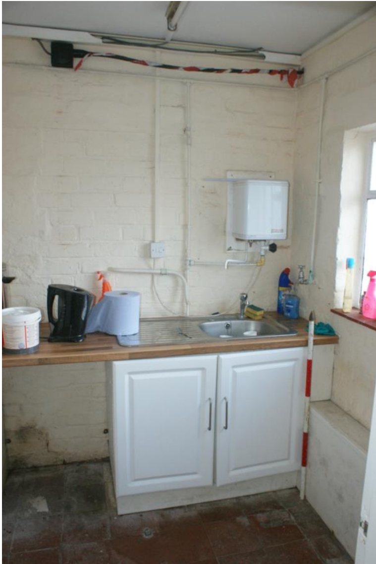
Plate 17 Building D rear extension ground floor, looking west
