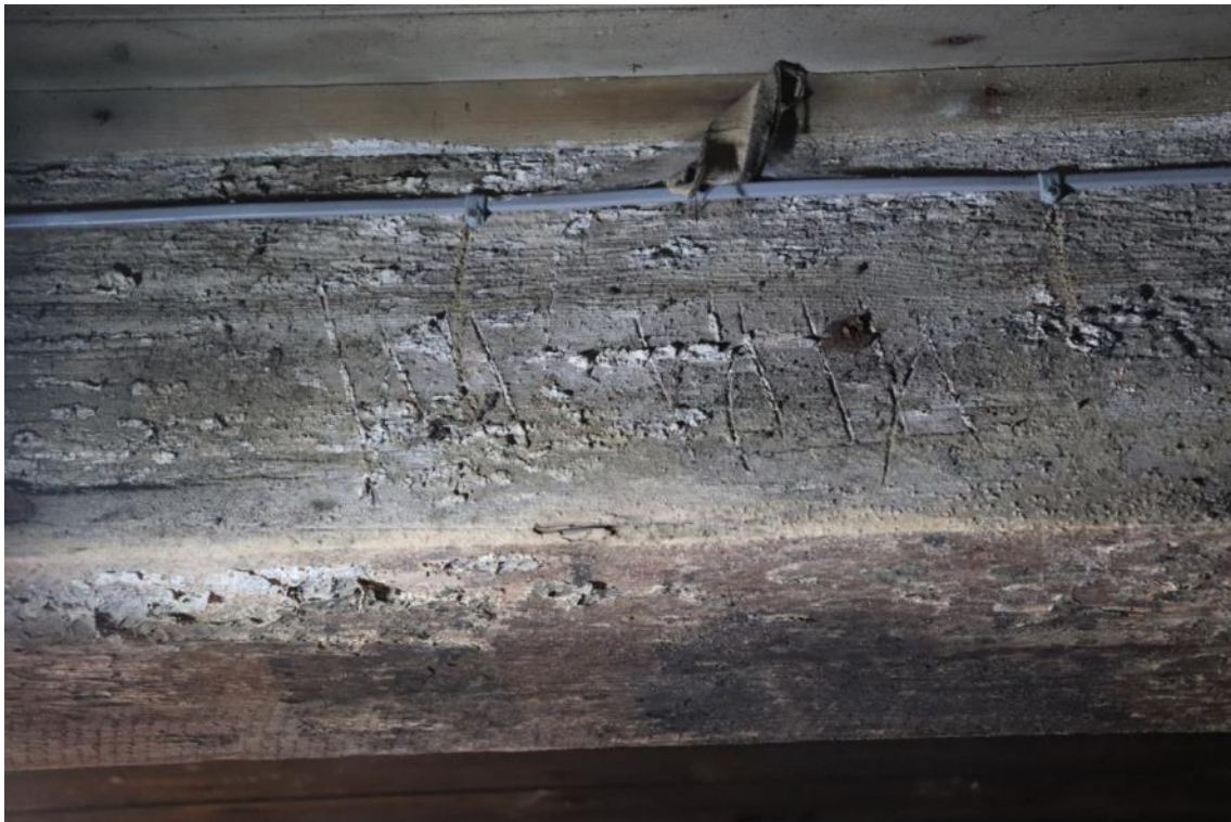
Plate 23 Building B ground floor ceiling joists Baltic timber marks, looking east
