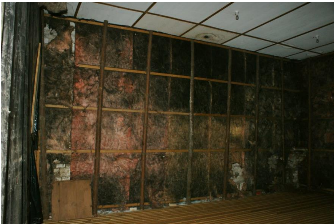
Plate 53 Building C first floor, looking north
