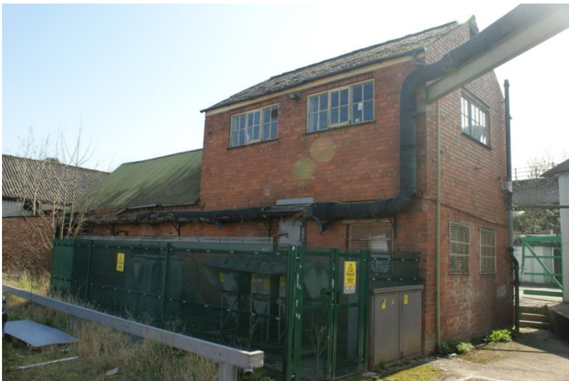
Plate 64 Building I, looking south-west
