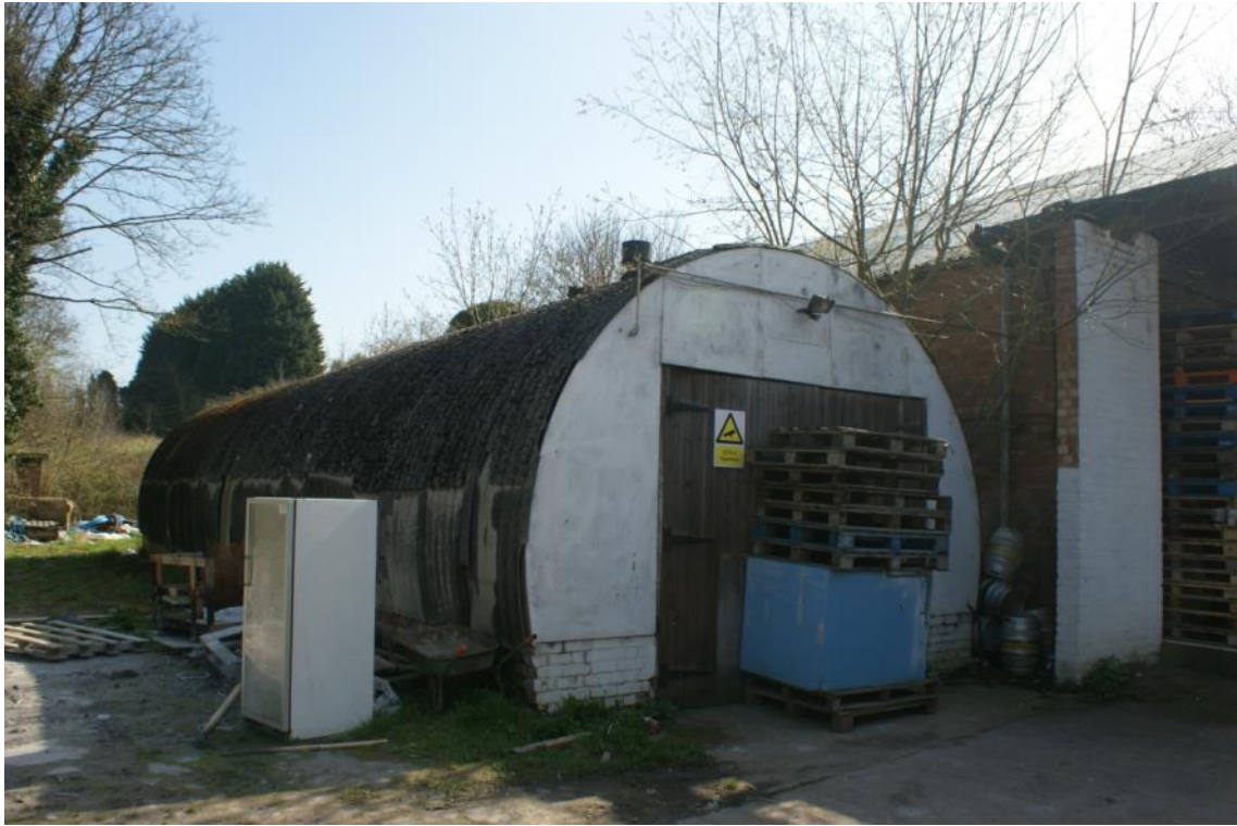
Plate 70 Building K, looking east
