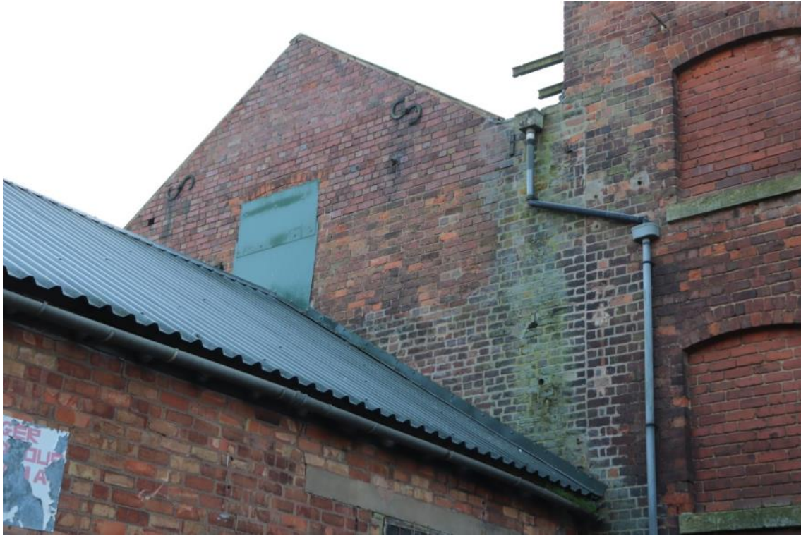
Plate 4 Phase 1 structure, looking south-east
