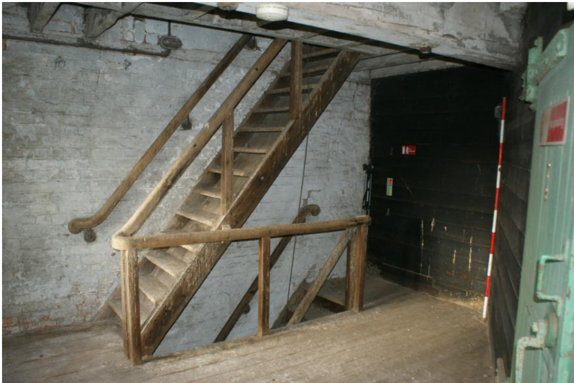
Plate 29 Building B fourth floor, looking north-west
