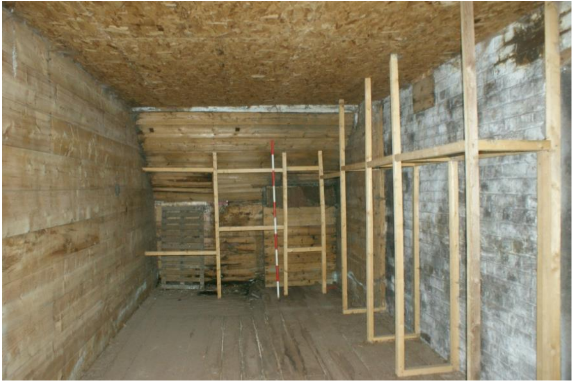
Plate 41 Building B fifth floor, looking north
