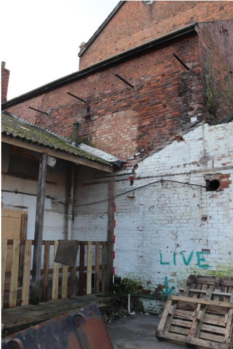
Plate 3 Phase 1 structure, looking south-west
