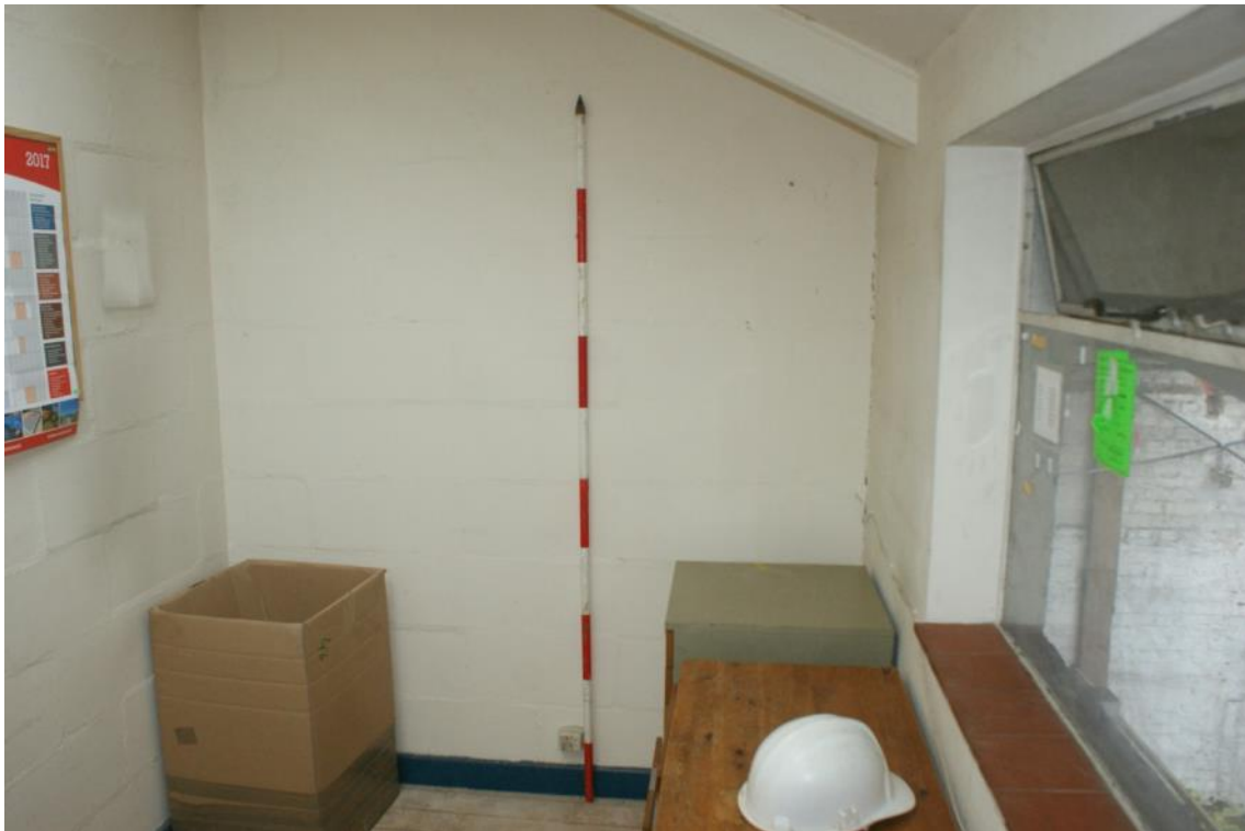
Plate 62 Building D first floor extension, looking west
