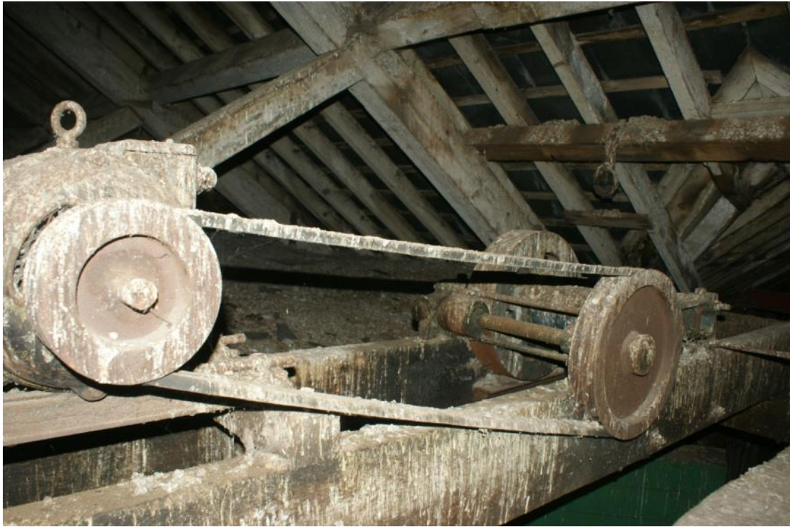
Plate 31 Building B fifth floor hoist machinery, looking south-east
