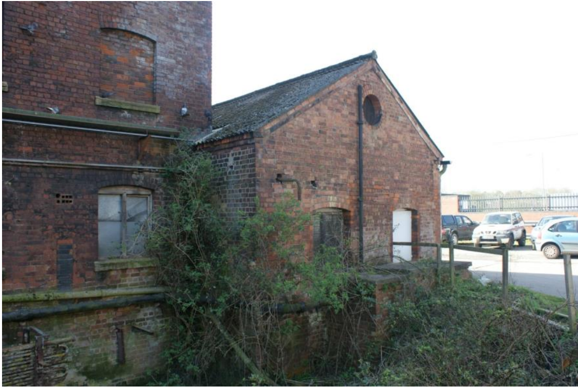
Plate 39 Buildings A and B, looking south- west
