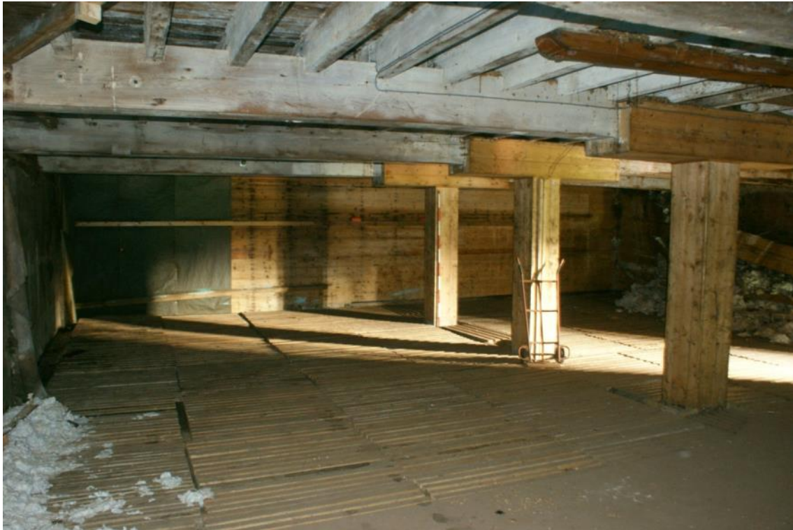
Plate 26 Building B third floor, looking east
