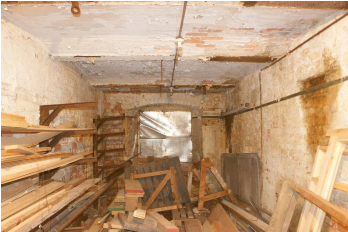
Plate 40 Building B ground floor, looking north
