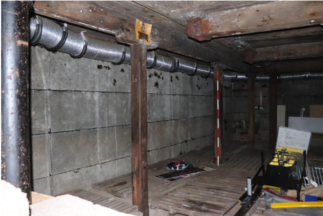
Plate 28 Building B ground floor, looking north-east
