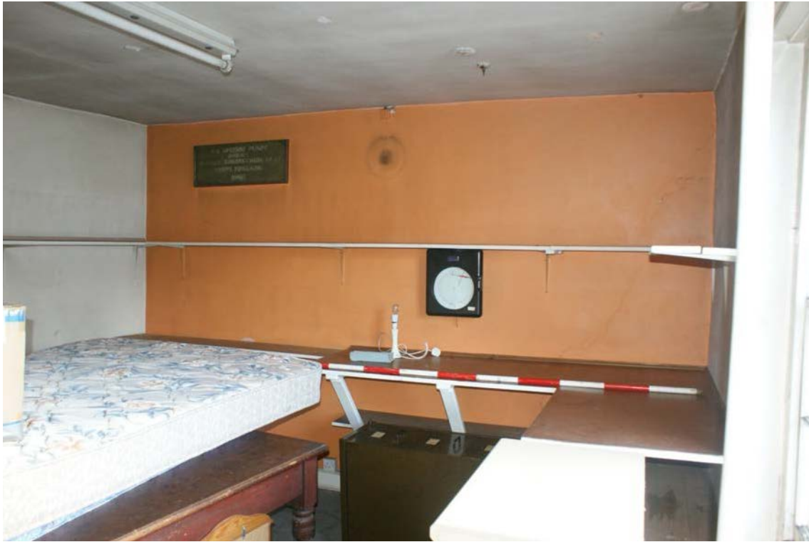
Plate 13 Building D first floor, looking east
