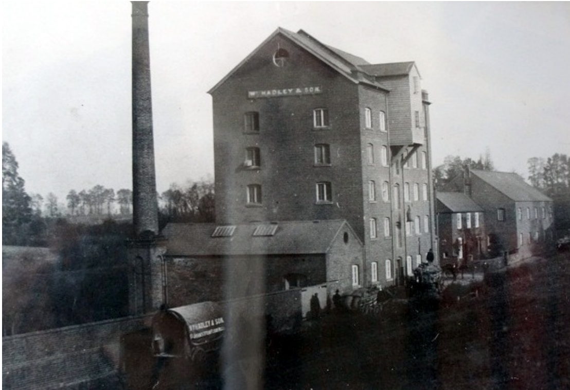
Plate 20 Buildings A, B, D and E in the early 1880s, looking north-east. Note the sack in the process of being lifted below the lucam (reproduced courtesy of Worcester and Midland Coldstores Ltd)
