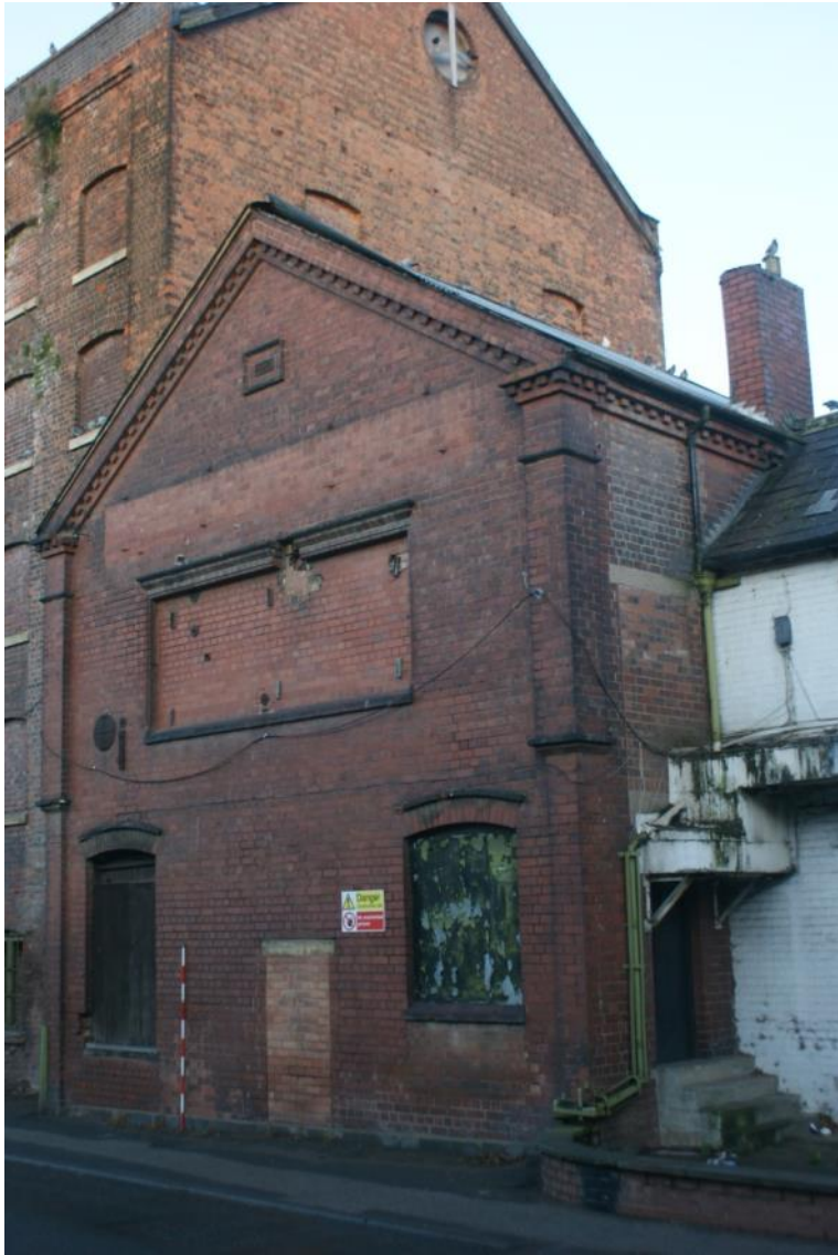
Plate 51 Building C, looking north-west
