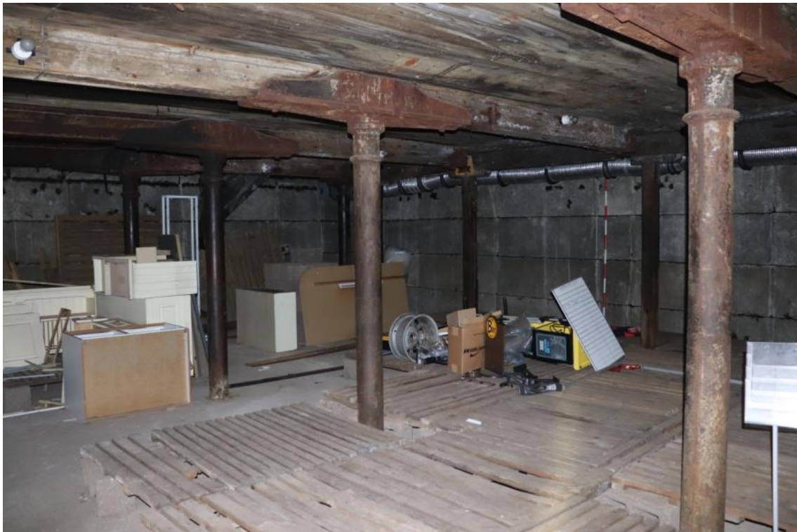
Plate 27 Building B ground floor, looking north-west
