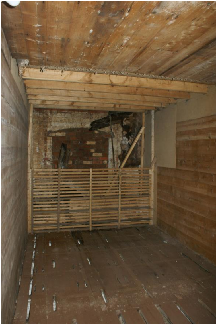
Plate 42 Building B fourth floor, looking south
