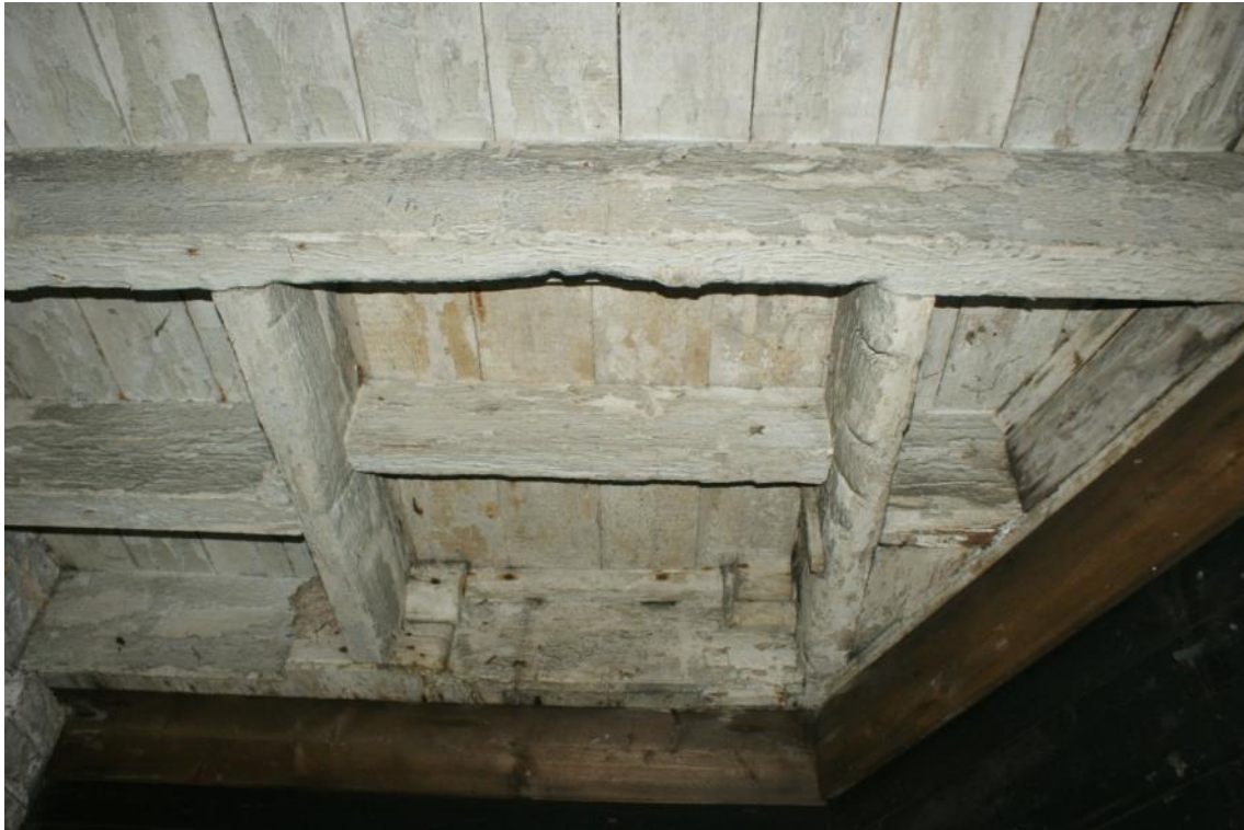
Plate 35 Building B first floor hatch, looking north
