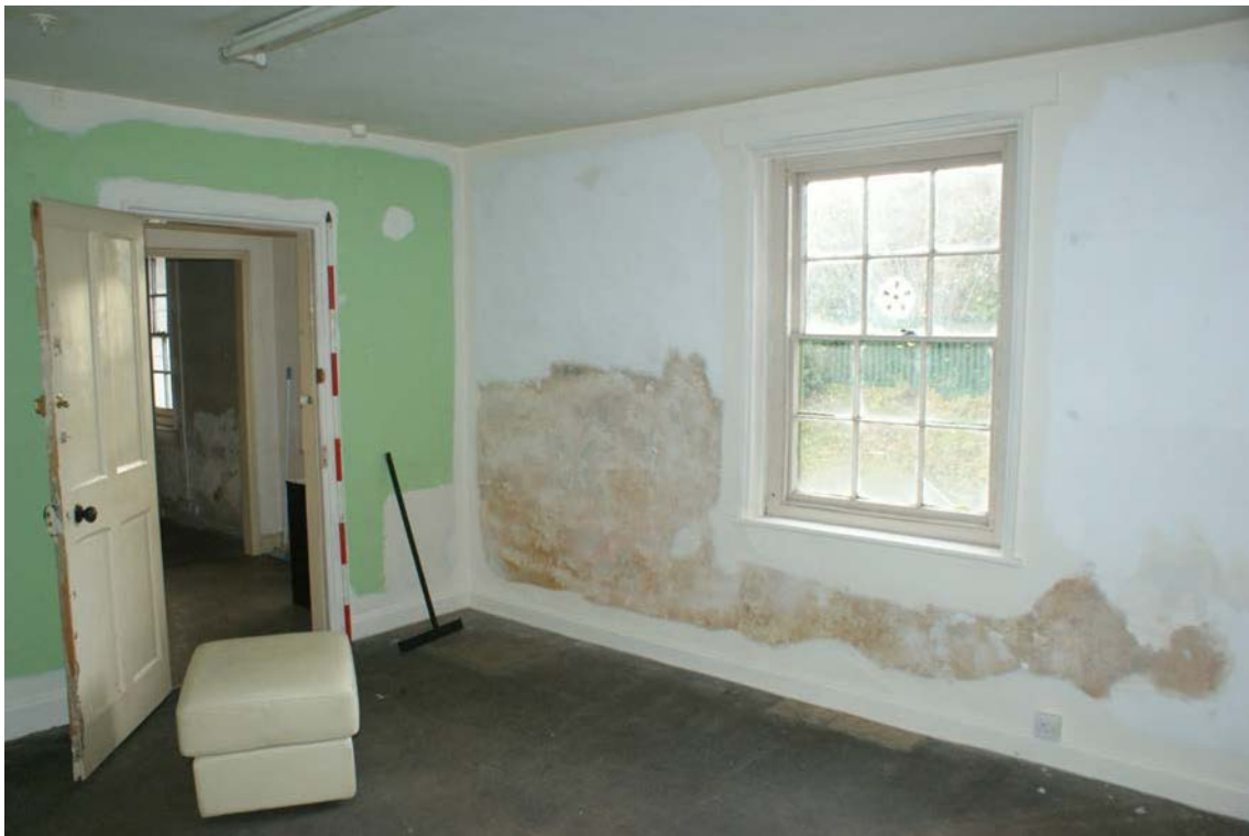
Plate 14 Building D first floor, looking south-east
