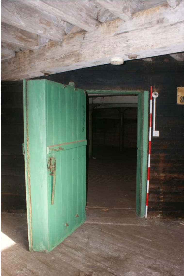
Plate 58 Building B fourth floor. looking north-east
