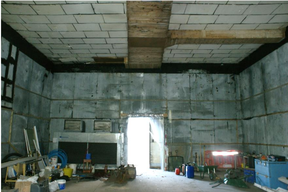
Plate 48 Building E interior, looking east
