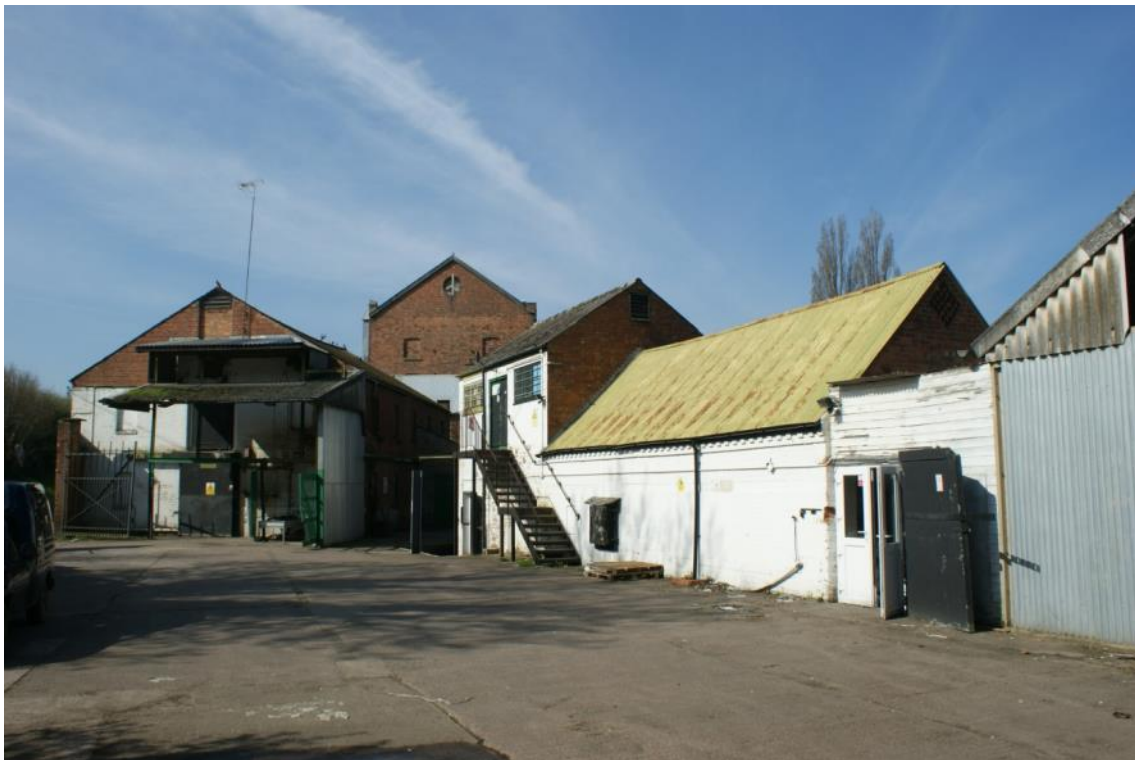
Plate 2 The former Ice Works buildings, looking north-east
