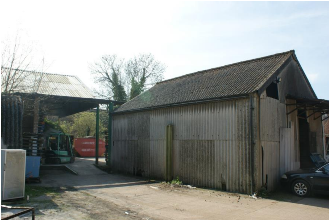
Plate 71 Building J, looking south
