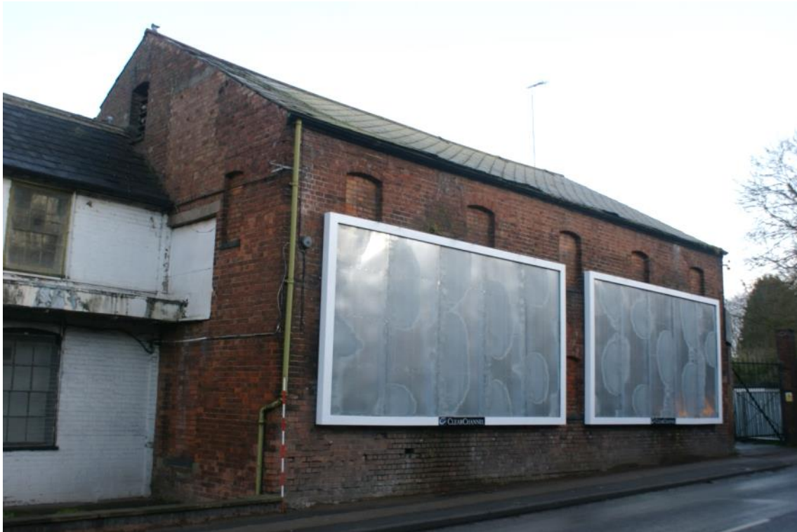
Plate 46 Building E, looking north-east
