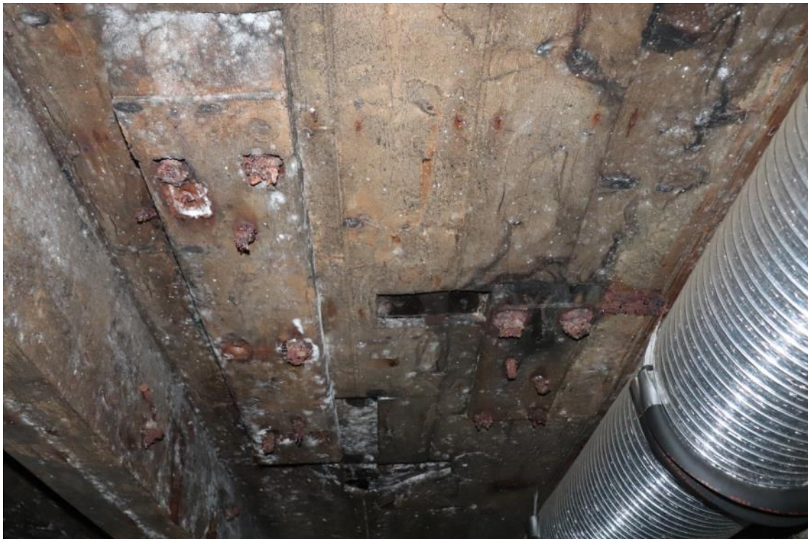
Plate 38 Building B ground floor possible machine positions, looking east
