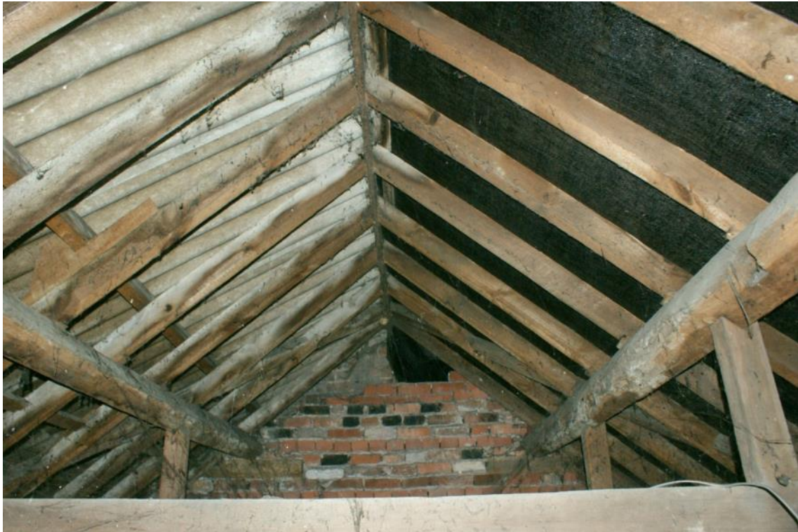
Plate 15 Building D roof space, looking east
