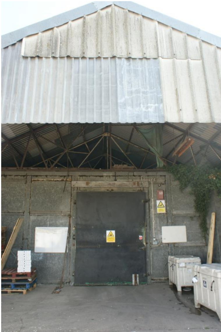
Plate 72 Building L, looking east
