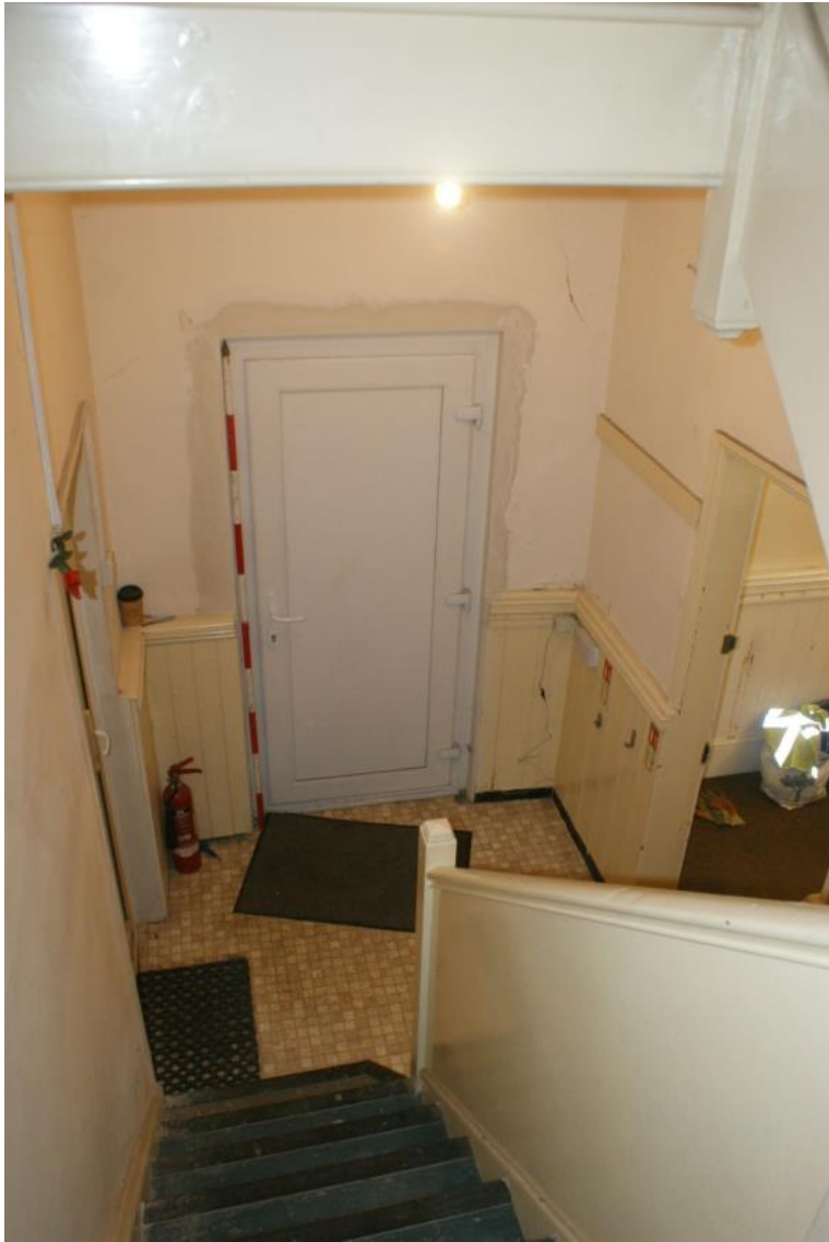
Plate 12 Building D first floor, looking south
