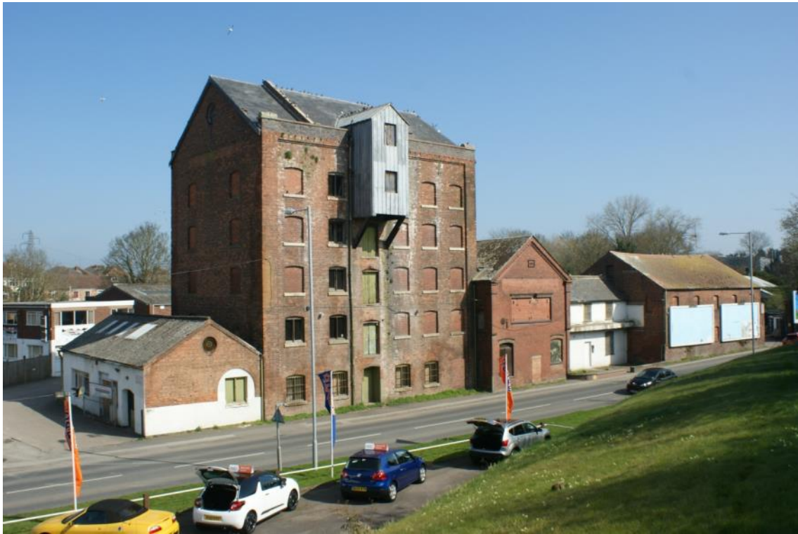
Plate 1 The former Ice Works buildings, looking north-east
