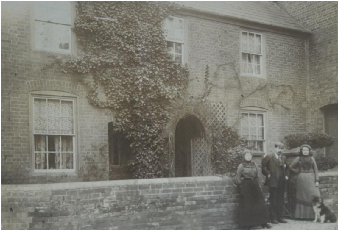
Plate 8 Building D c 1890-1910, looking north-east (reproduced courtesy of Worcester and Midland Coldstores Ltd)
