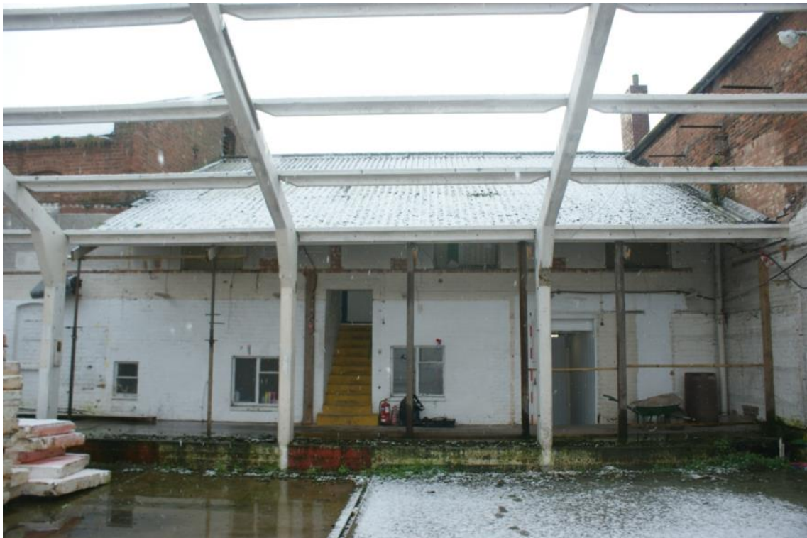
Plate 16 Building D rear extension, looking south
