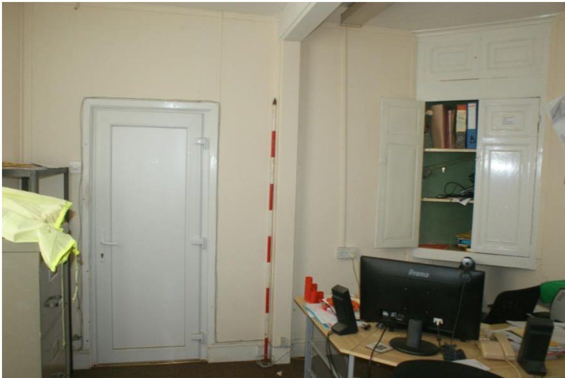
Plate 11 Building D ground floor, looking west
