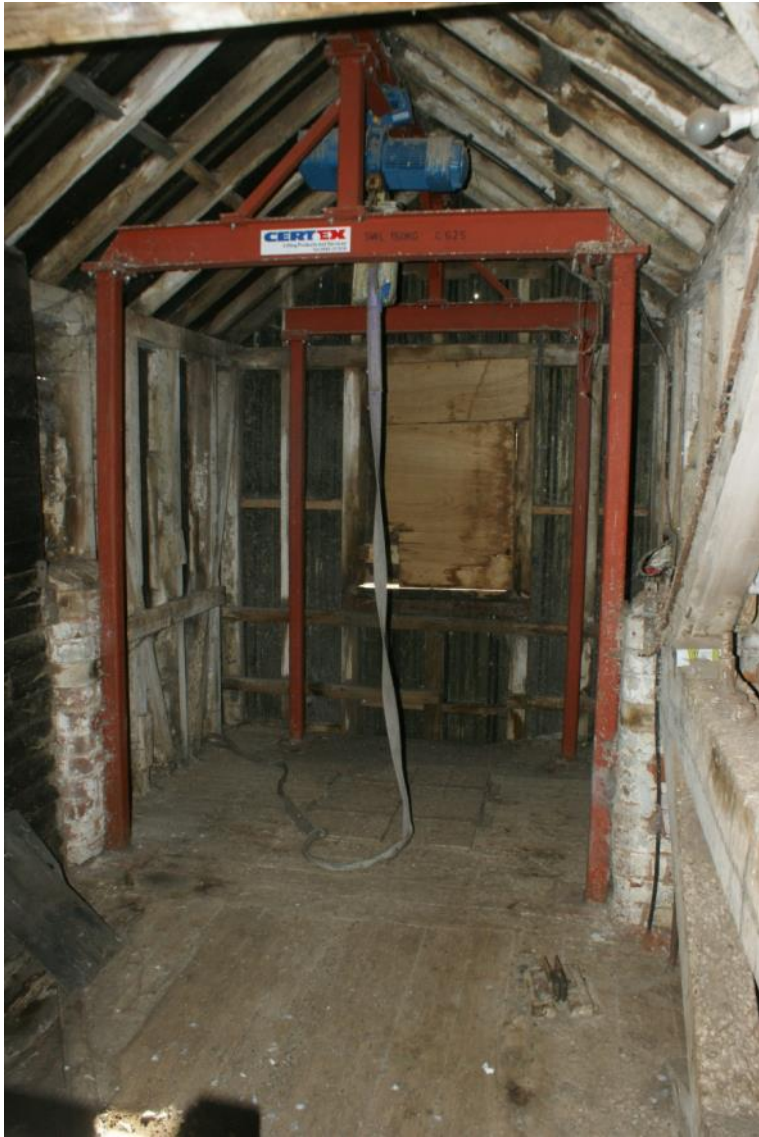
Plate 32 Building B fifth floor lucam interior, looking south
