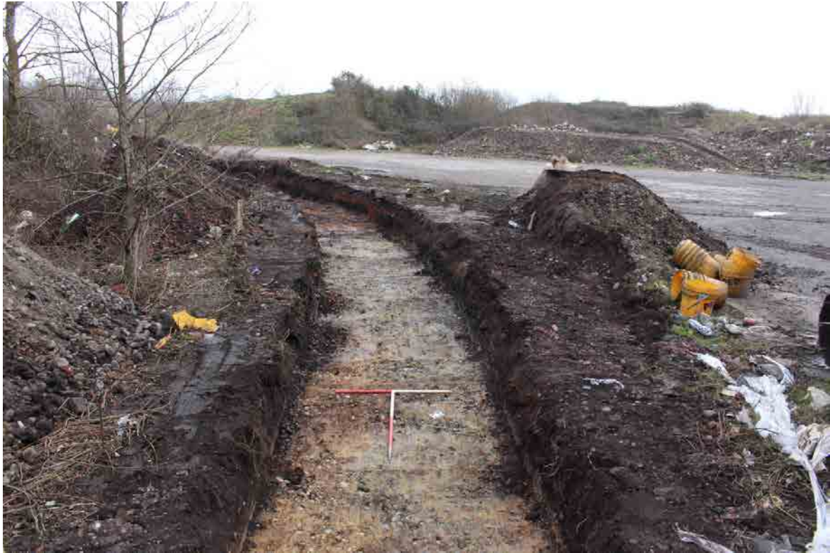
Plate 5: Trench 8 general view, facing south-east, 2x 1m scales
