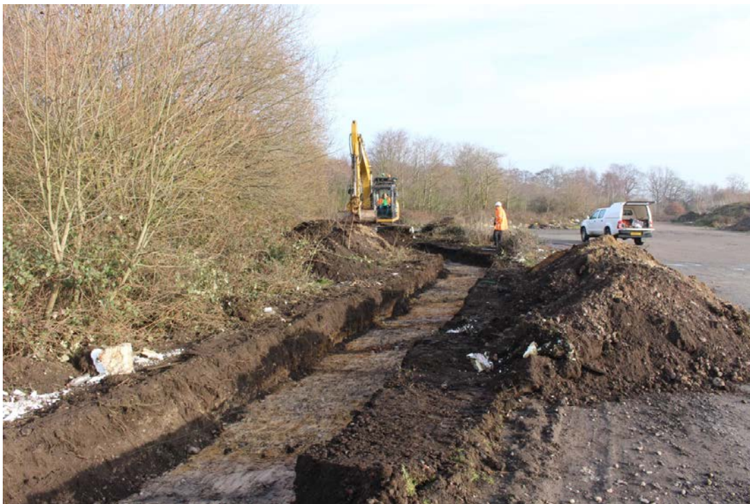
Plate 2: General working shot of Trench 7 during excavation, facing north-east, no scales
