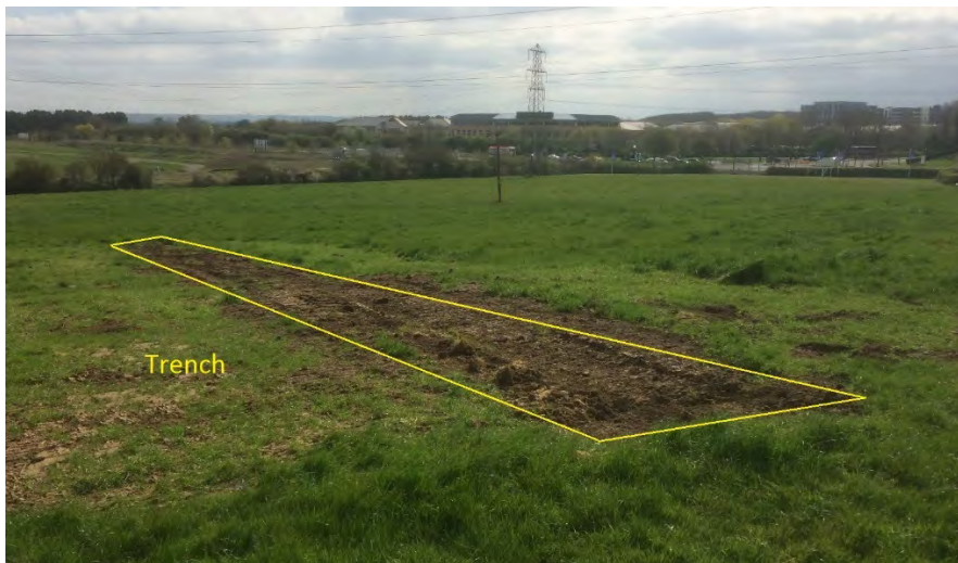
View of backfilled trench
