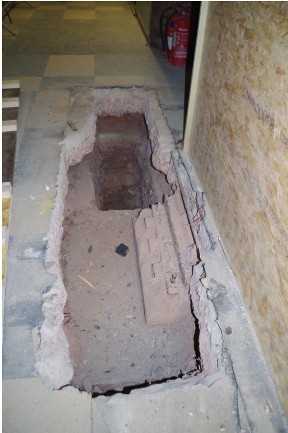
Plate 17: Trial Hole 5, looking north-east
